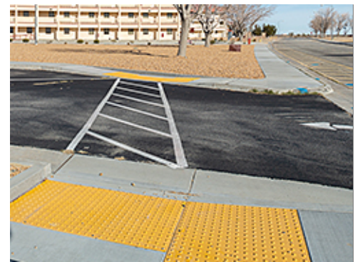
Accessible Ramp and Crosswalk
