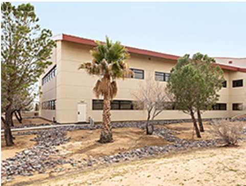
Roof Drains to Rock Mulch Swale
