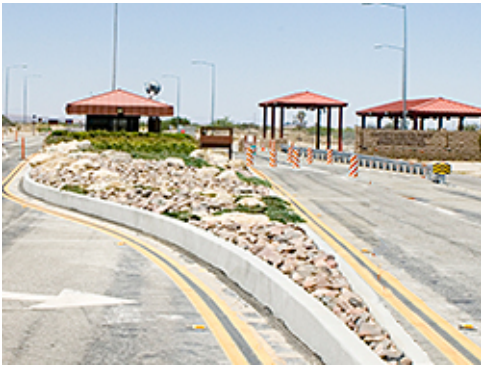
Main Entrance Facilities and Landscape
