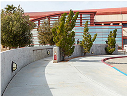
Site Ramp at Group 1
