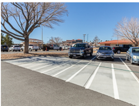
Concrete Paving and White Striping
