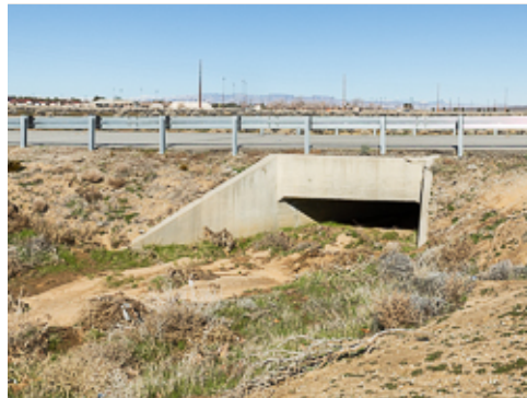
Concrete Box Culvert
