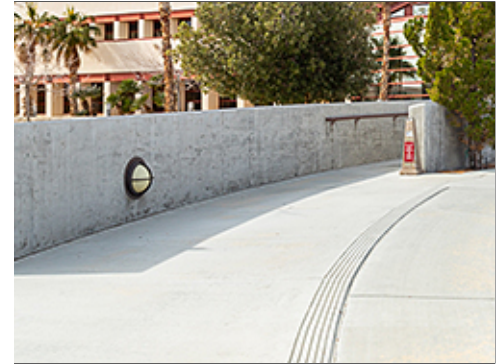
Wall Mounted Light Fixture
