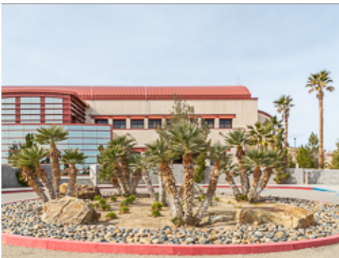
Accent Planting at Facility Group 1
