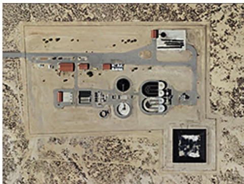
Base Water Treatment Plant
