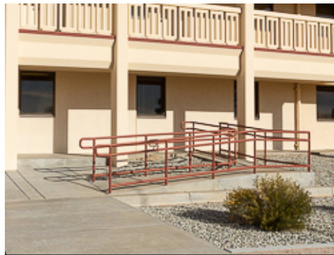
Site Ramp at Group 2
