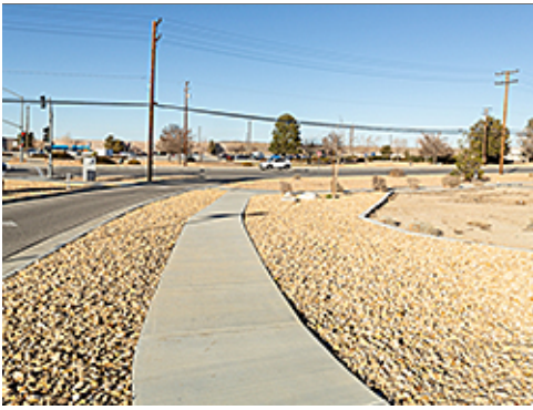
Detached Sidewalk along Street
