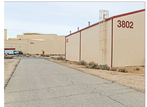
Local Street at Group 3
