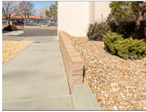
Sidewalk at Group 2 Facility
