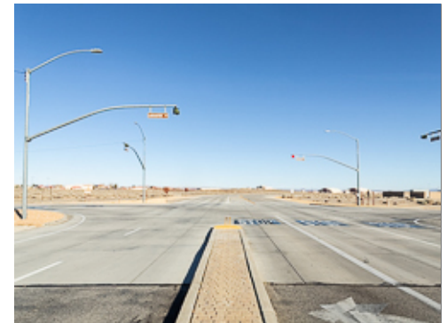
Arterial with Paved Median
