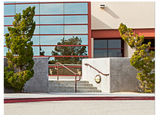
Site Stair at Group 1
