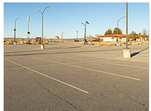
Striping with Coordinated Light Fixtures
