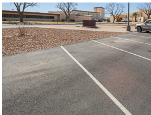
Asphalt Paving and White Striping
