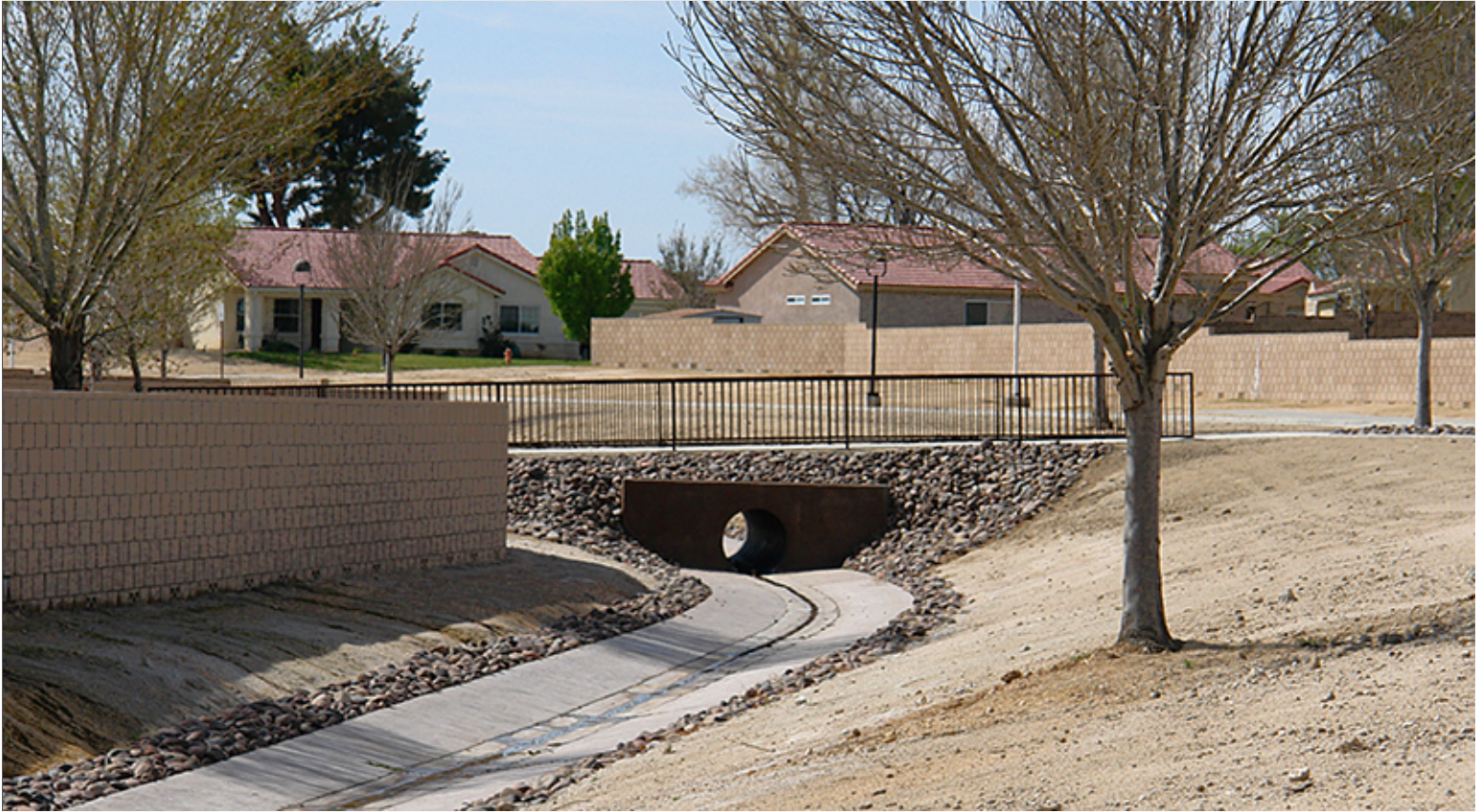
Stormwater Feature as an Amenity
