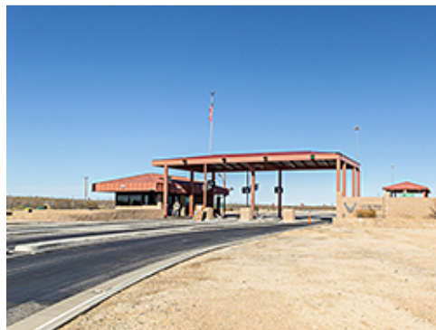
Main Gate at Perimeter Fence
