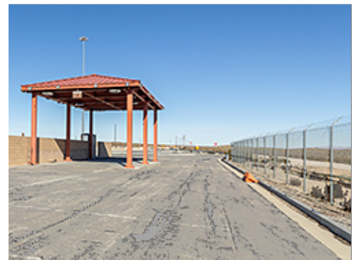
Fencing at Entrance Control Facility
