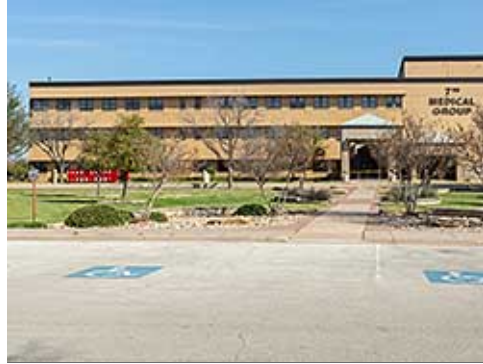
Asphalt Paving at Group 1
