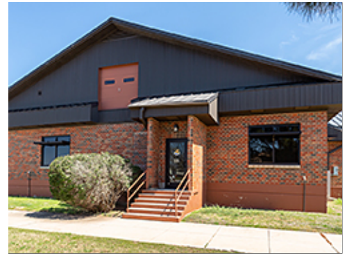
Stair at Secondary Entrance
