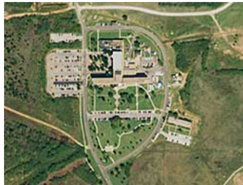
Hospital Wing with East-West Orientation
