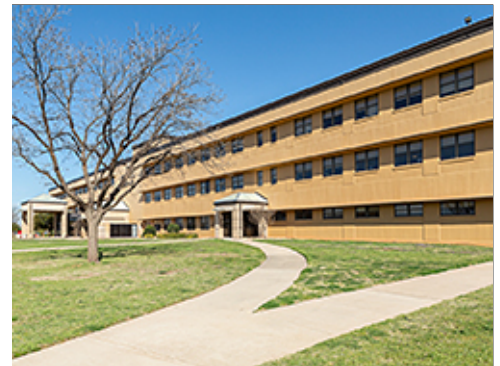
Natural Concrete at Secondary Entrances
