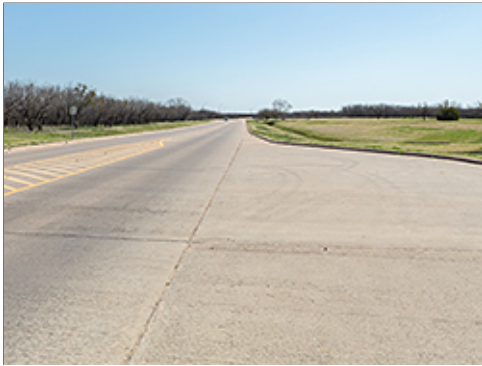
Concrete Paving
