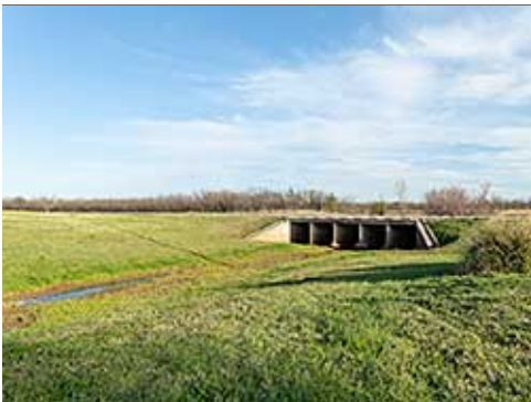
Vegetated Drainage Swale
