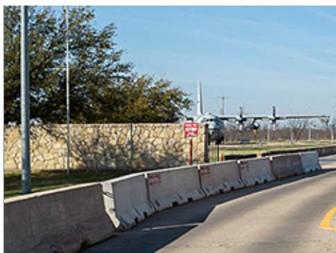
Stone Wall at Main Gate Entrance
