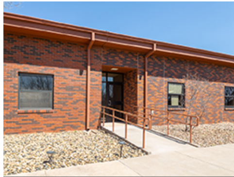
Ramp at Secondary Entrance
