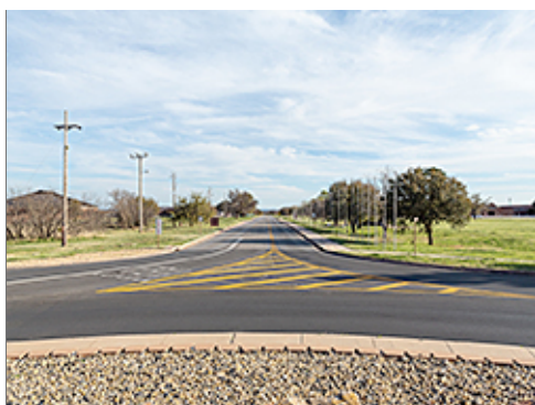
Special Striping at Roundabout
