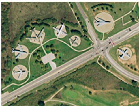
Aerial Photo of Dyess AFB Linear Air Park
