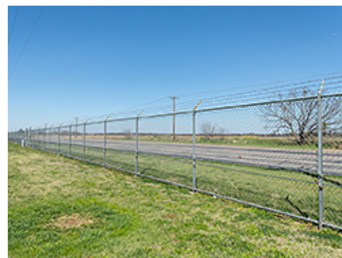
Chain Link Fencing along Group 3
