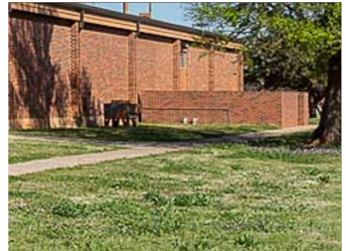
Masonry Screen Wall
