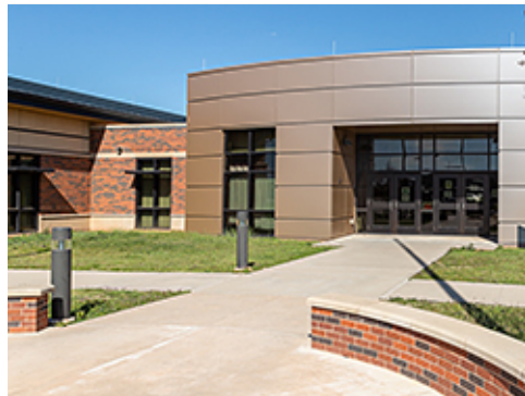
Masonry Low Wall at Group 1
