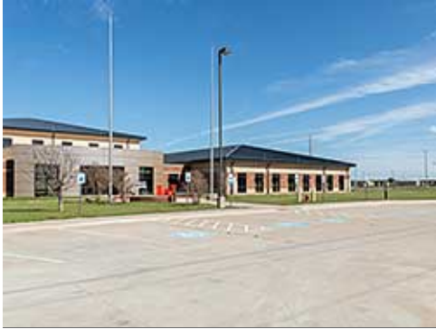
Concrete Paving at Group 1
