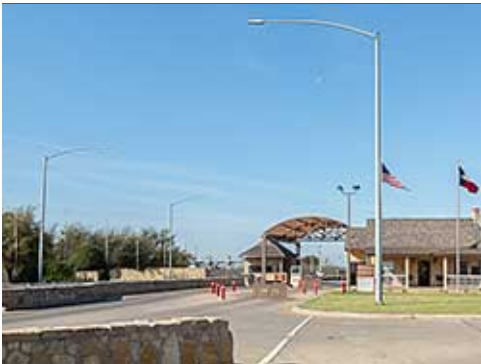
Street Fixtures at Main Gate
