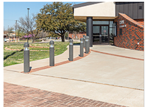
Lighted Bollards at Main Entrance
