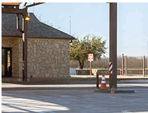
Steel Fencing Near Main Gate
