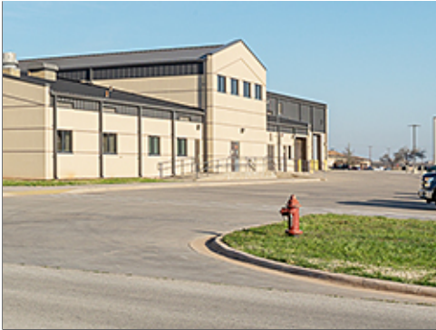
Typical Fire Hydrant
