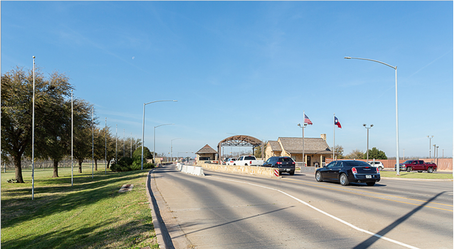
Main Gate at Arnold Boulevard
