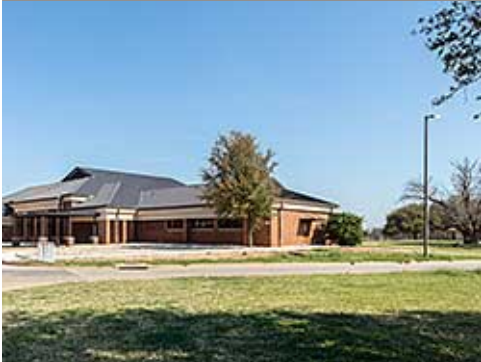
Buried Utility Service Lines
