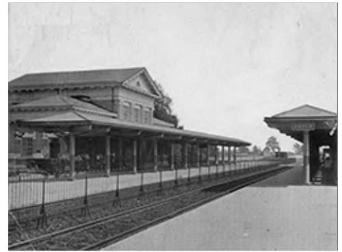
Track-side PRR Station Dover, Delaware
