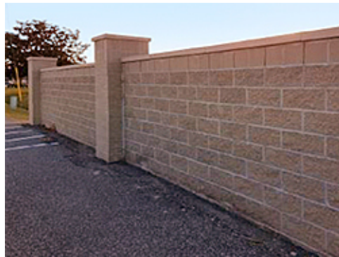
Group 2 CMU Screen Wall
