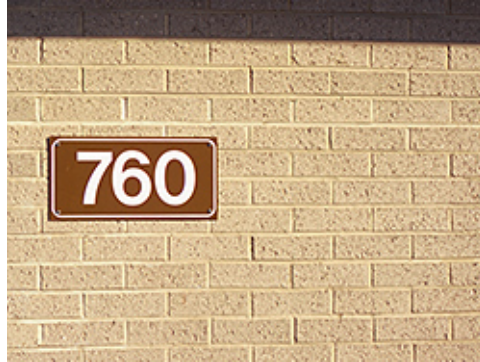
Building Number Sign
