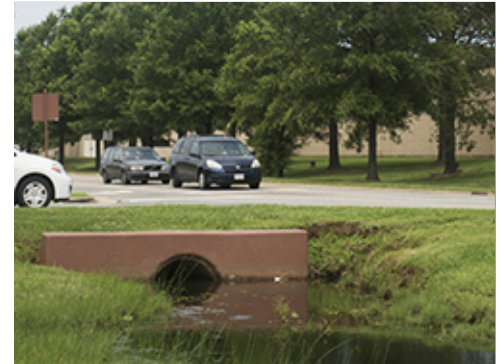
Stormwater Discharge to Swale
