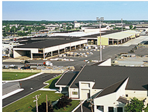
Dover AFB Flightline Support Facilities
