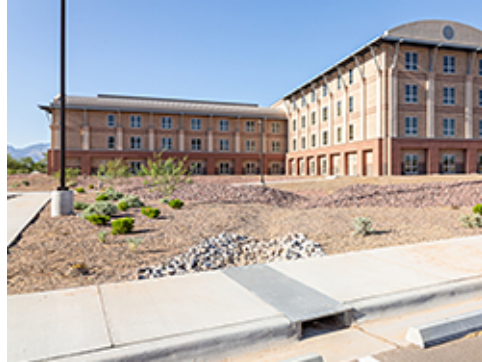
Storm Drainage Elements
