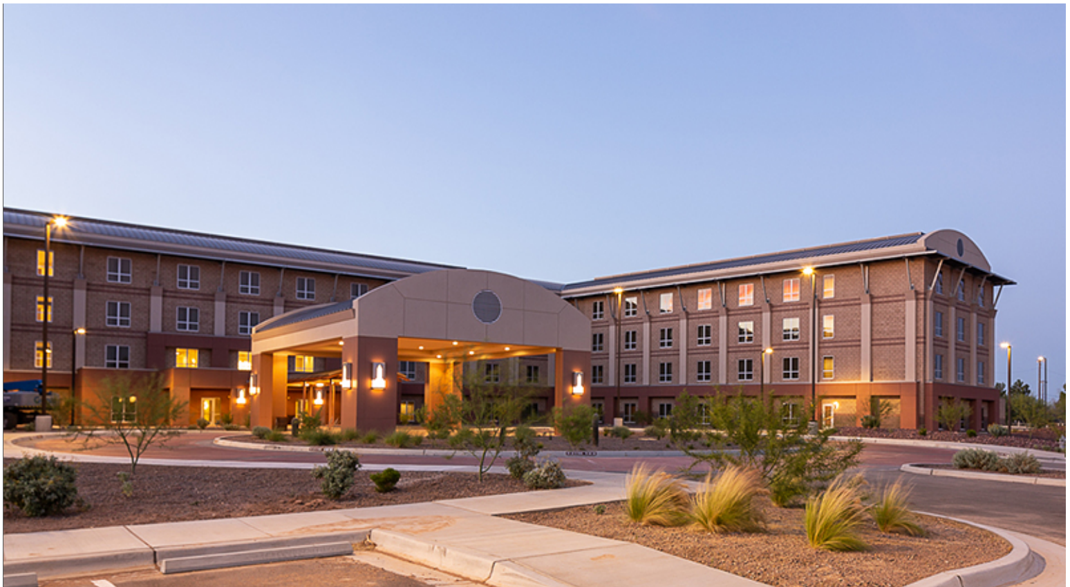
Ambient Lighting From Parking Lot Fixtures and Building Fixtures
