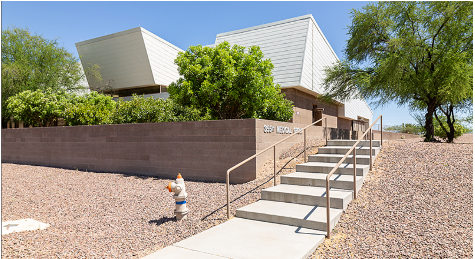
Site Stair at Group 1
