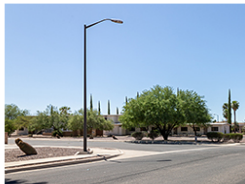
Lighting at Group 4
