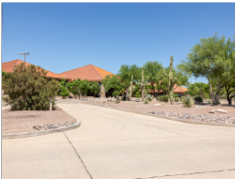
Limited Access Drive in Group 1
