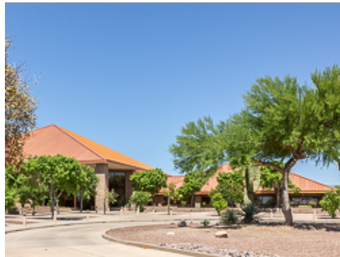
Group 1 Standing Seam Roofing
