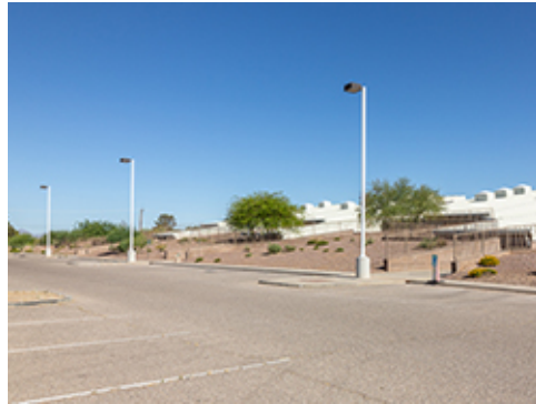
Parking Lot Lighting
