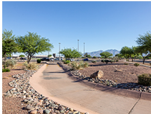
Drainage Feature Serving as Sidewalk
