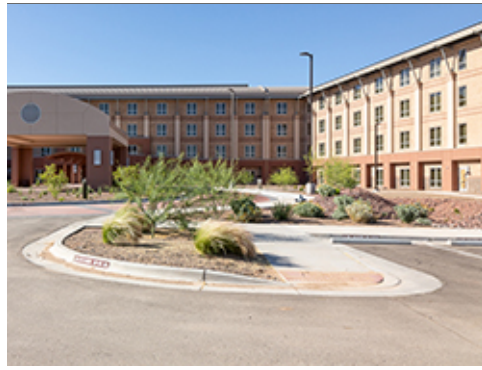
Curb Ramp at Group 2
