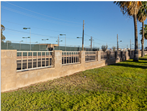
Masonry Fencing near Group 1
