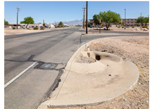
Drainage Inlet Element
