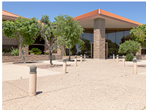
Exposed Aggregate Paving at Group 1
