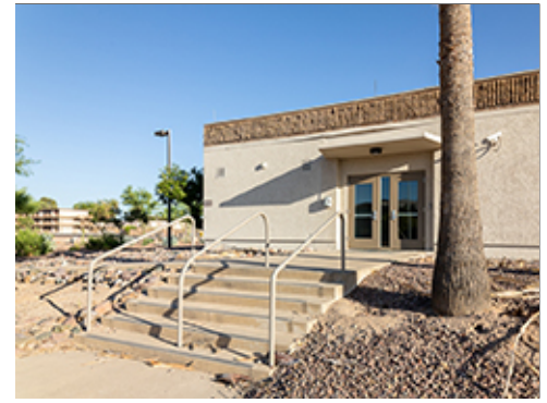
Site Stair at Group 3
