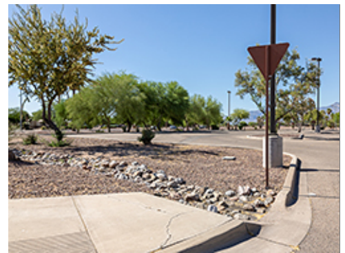
Integrated Drainage Elements
