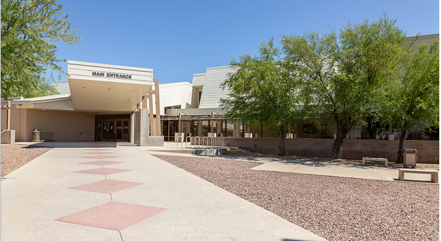
Concrete Paving with Colored Concrete Accents
