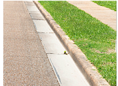
Standard Curb and Gutter
