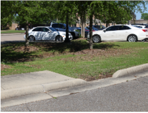
Curb Cut for Stormwater Management
