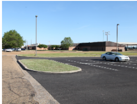
Group 2 Asphalt Paving and Striping
