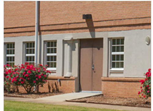
Facade Lighting Also Serving Sidewalk
