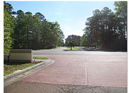
Special Paving at Intersection
