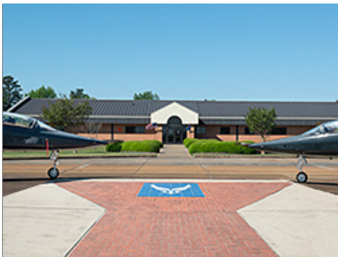
Colored Paving at DV Entrance
