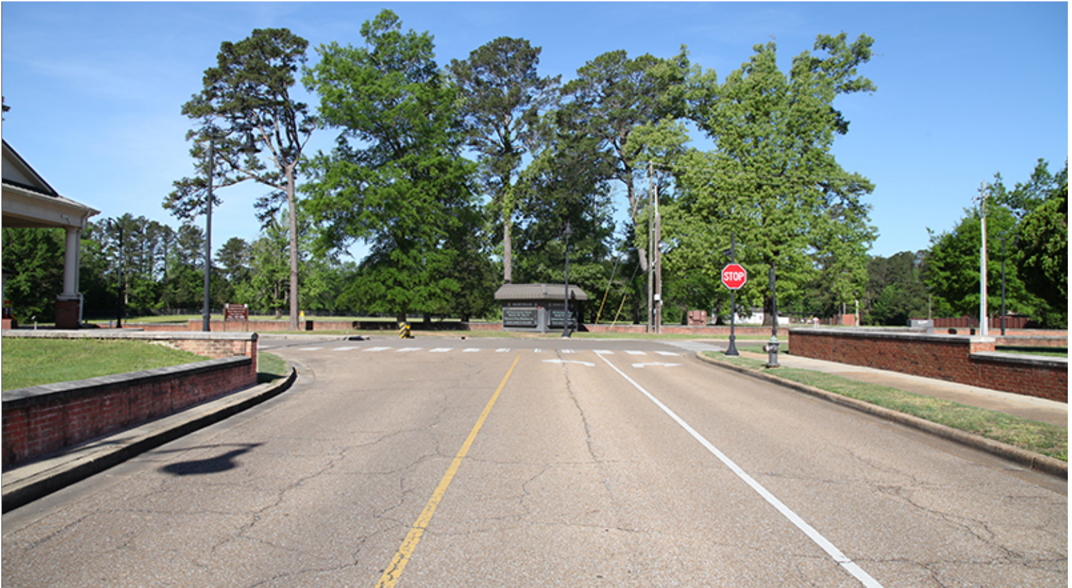
T Intersection at Group 1 Gate Facility
