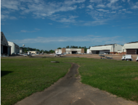
Concrete Used in Stormwater Management
