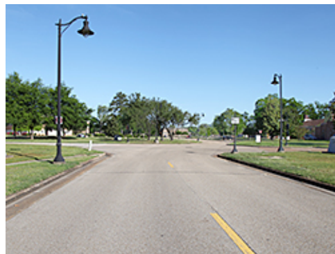
Collector along Group 1 and 2 Facilities
