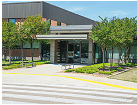
Vegetation Outlining Building Entrance
