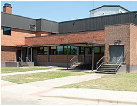
Stairs Serving Multiple Locations on a Facility
