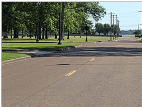
Bituminous Asphaltic Concrete Paving
