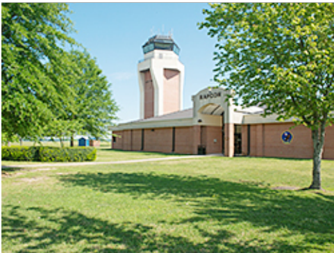
Group 2: RAPCON and Control Tower
