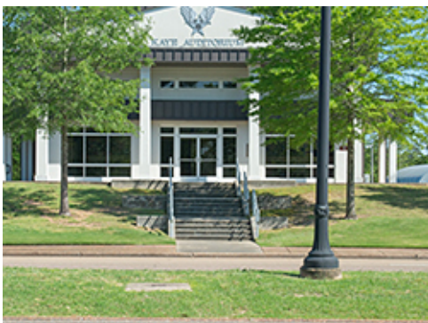
Stair Entrance to Group 1 Building
