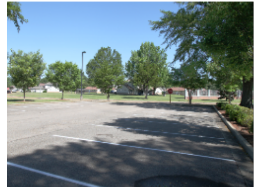
Group 4 Asphalt Paving and Striping
