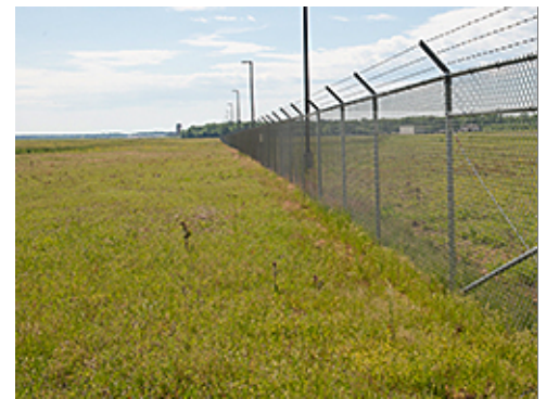
Chain Link Perimeter Fence at Group 3
