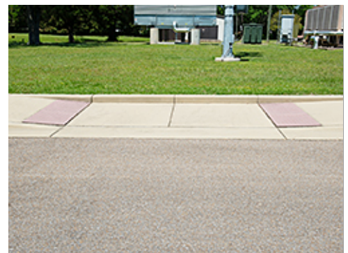
Curb Cut for Handicap Access
