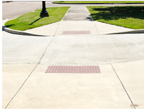
Sidewalk Curb Cuts with Warning Treads
