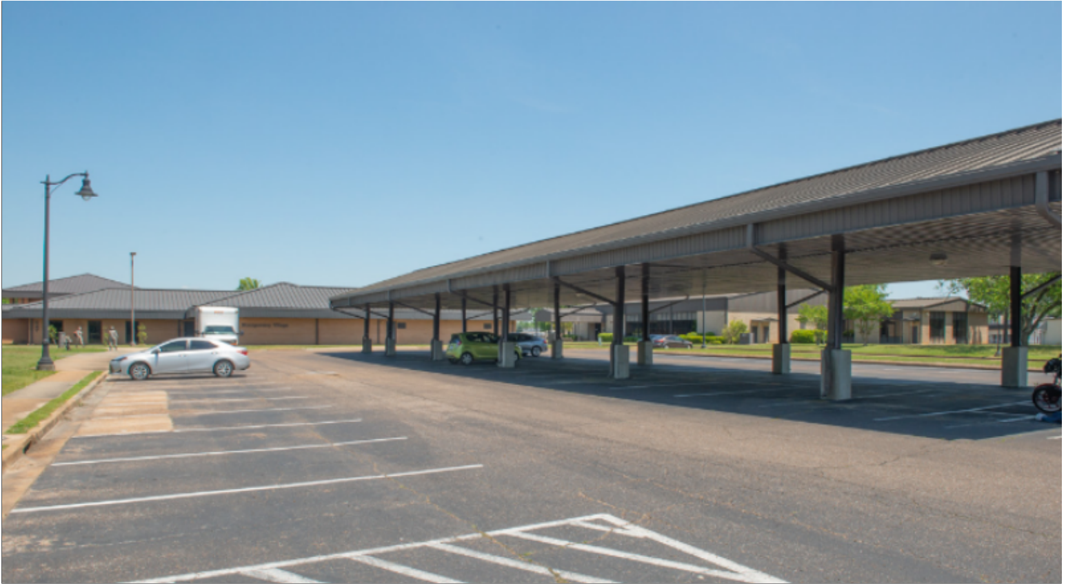
Group 2 Covered Parking Structure
