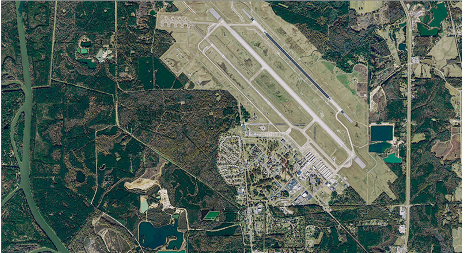
Aerial of Main Cantonment Area
