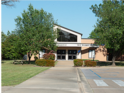
Sidewalk with Curbing at Parking
