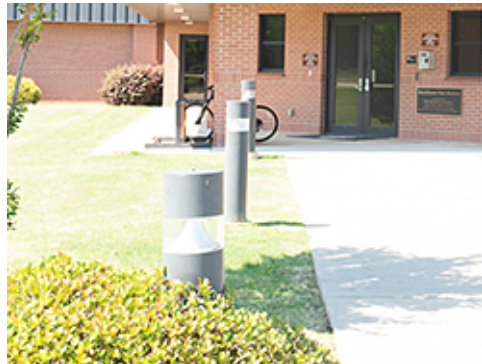
Lit Bollards Adjacent to Sidewalk
