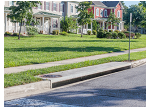
Stormwater Inlet at Curbing
