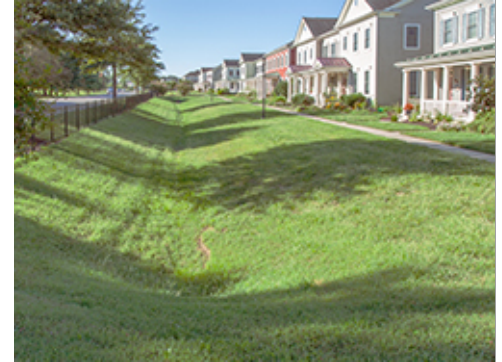
Swale with Grass Planting
