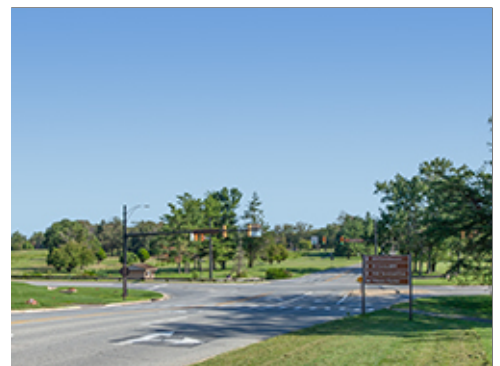
Virginia Avenue near Gate
