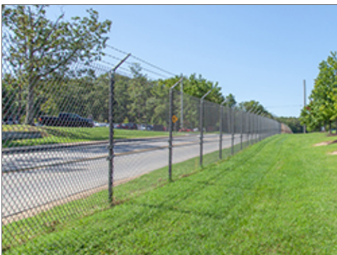
Galvanized Fencing along Perimeter Road
