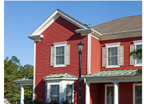
Gable End Wall in Group 4
