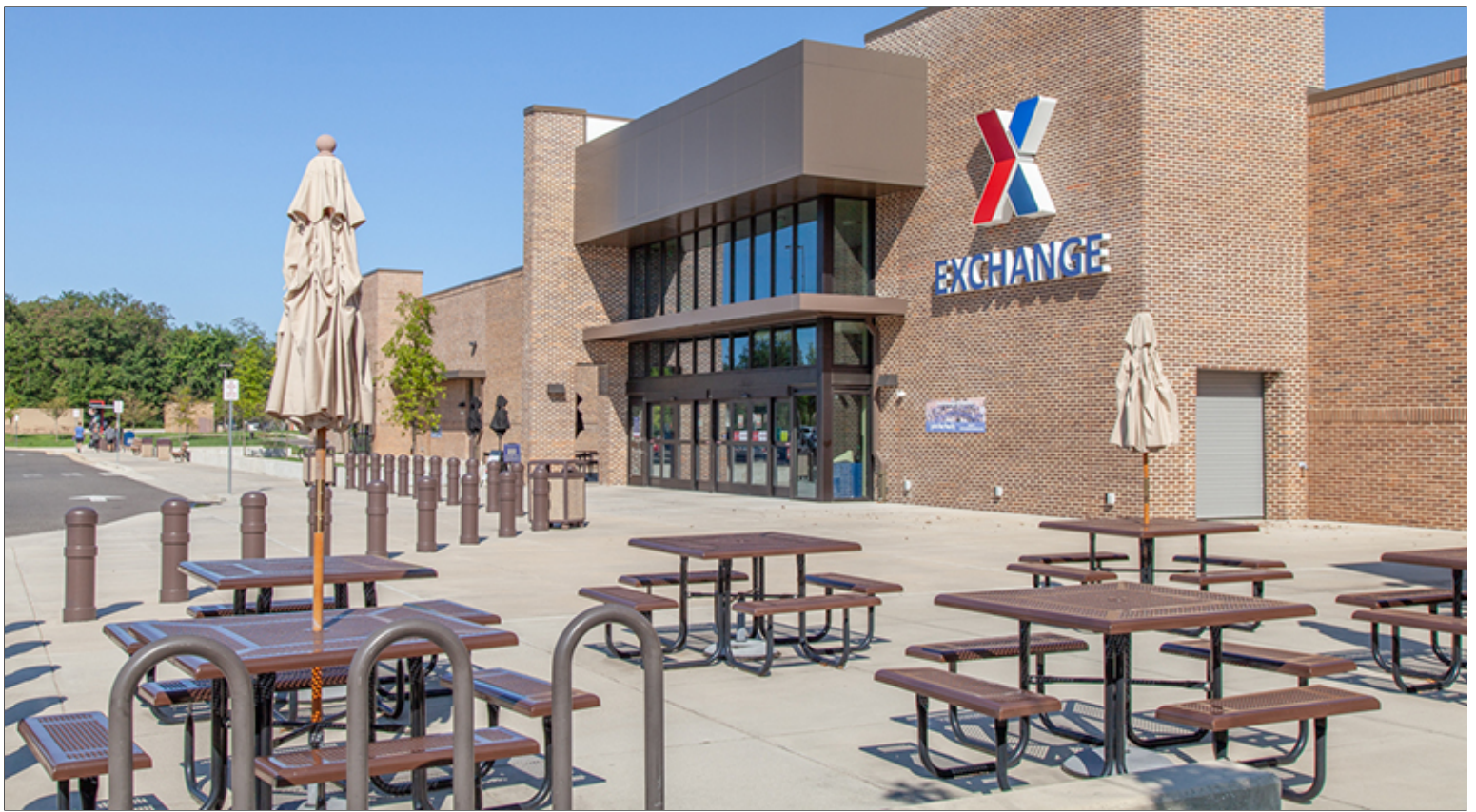
Concrete Paving with Integrated Site Furnishings at Group 2
