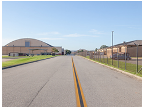
Fencing Adjacent to Restricted Facility
