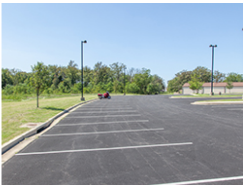
Bituminous Paving and White Striping
