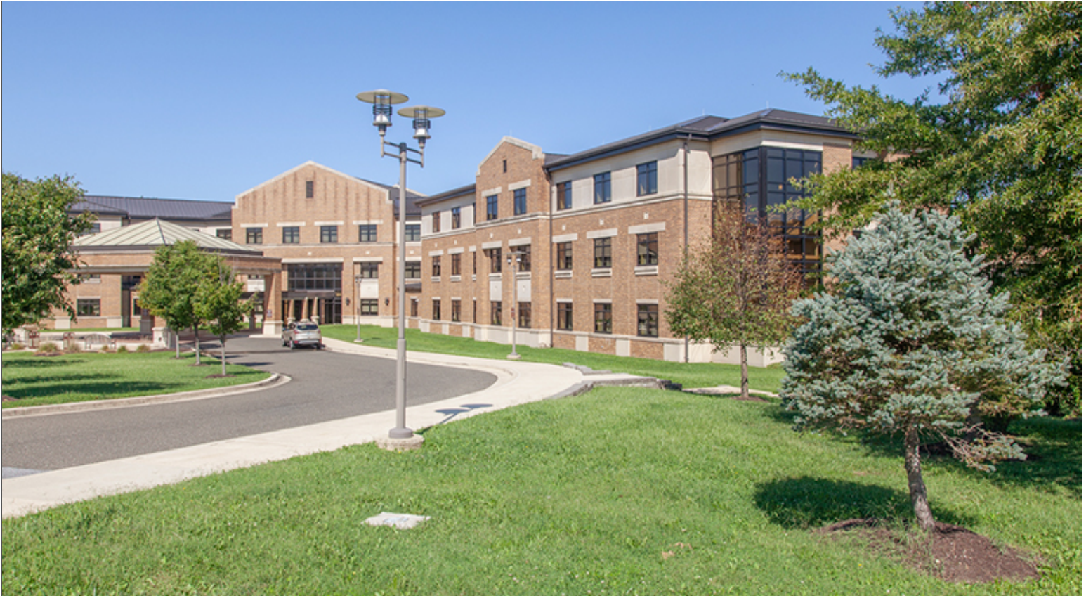
Attached Sidewalk at Group 2
