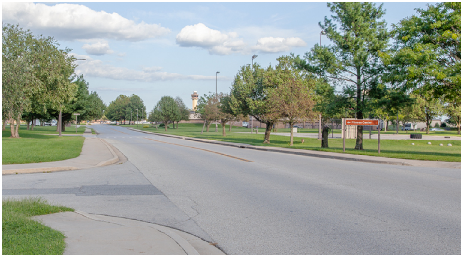
Unobstructed Lines of Sight at Intersection
