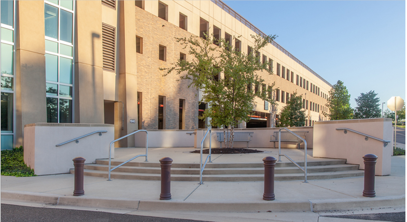
Concrete Plaza at Group 1
