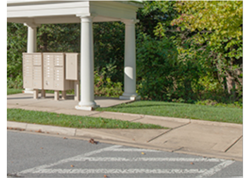
Curb Ramp at Street Crossing
