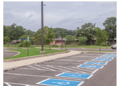
Striping at Accessible Parking
