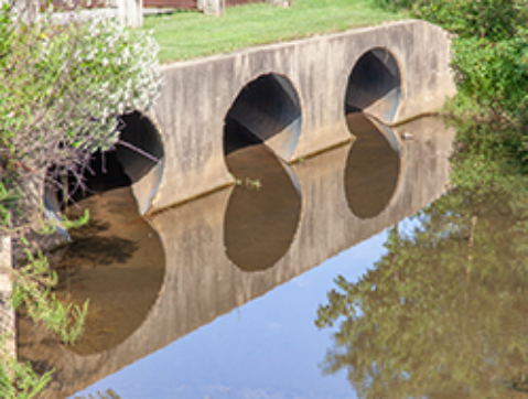
Storm Drainage Element
