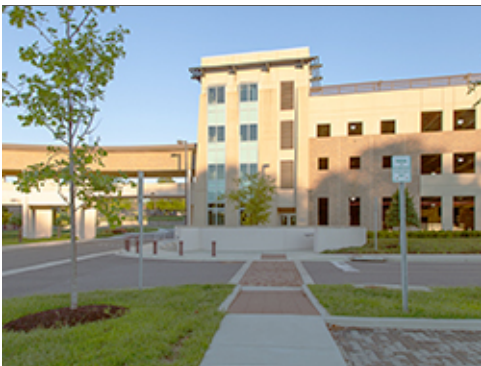
Parking Areas Linked to Entrance
