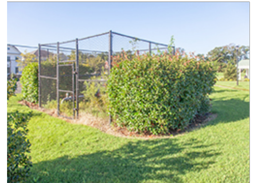
Landscape Screening at Utility Enclosure
