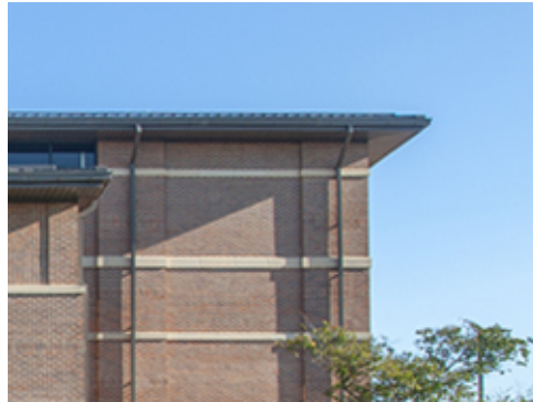
Roof Eave in Group 2
