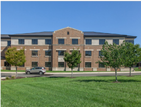
Group 2 Use of Brick and Precast
