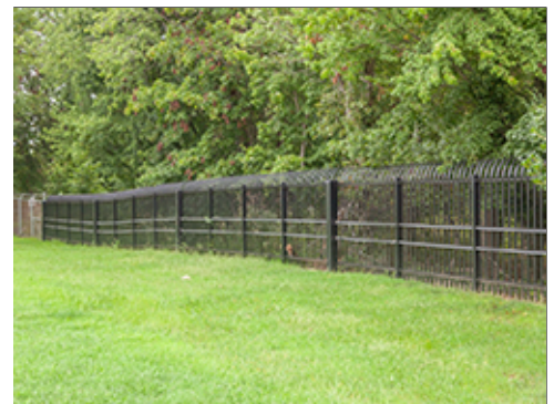
Metal Fence at Woodland Buffer
