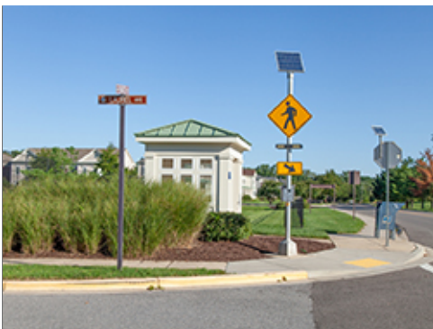
Coordinated Placement of Signs
