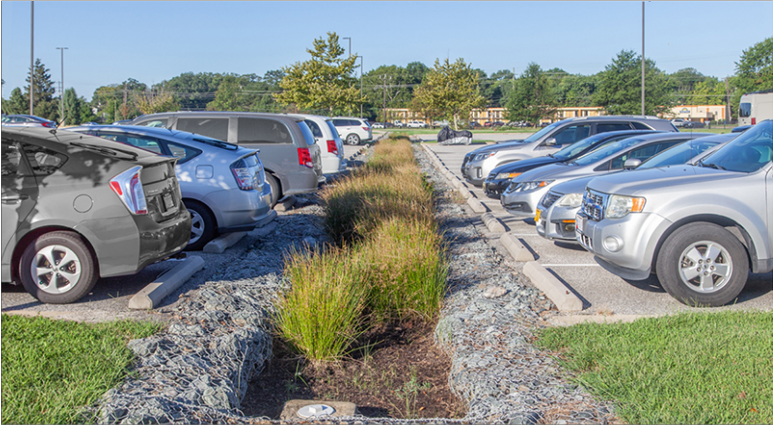
Bioswale and Stormwater Filtration
