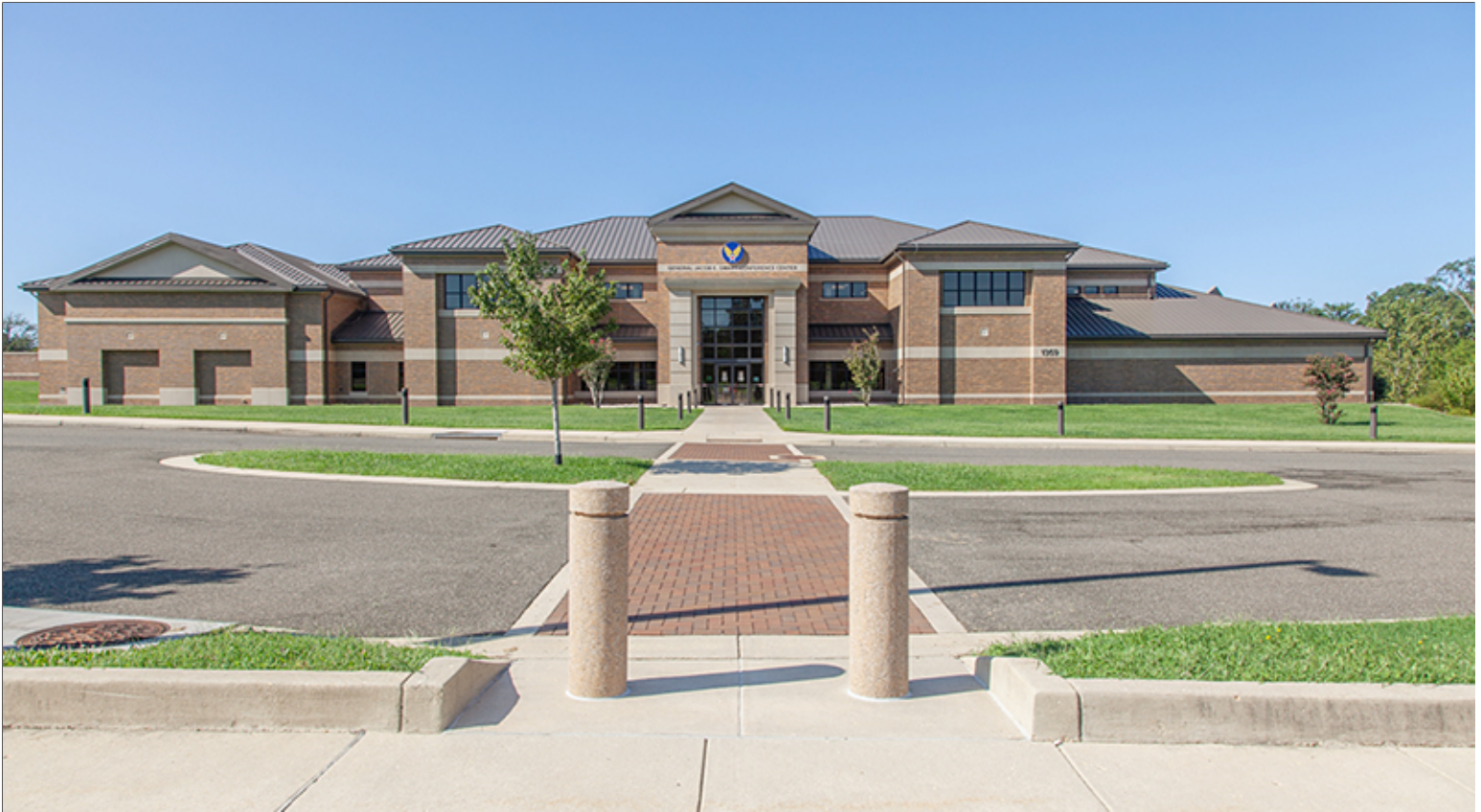
Connectivity at Group 2 Defined with Colored Pavers and Concrete Edging
