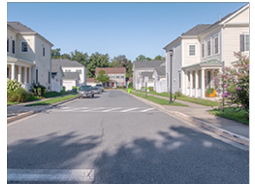
Standard Street Markings
