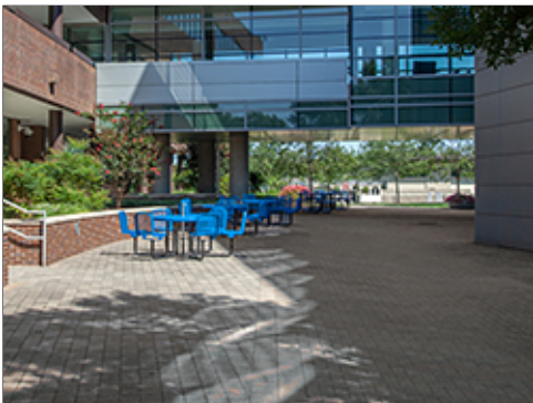
Interlocking Pavers at Group 1
