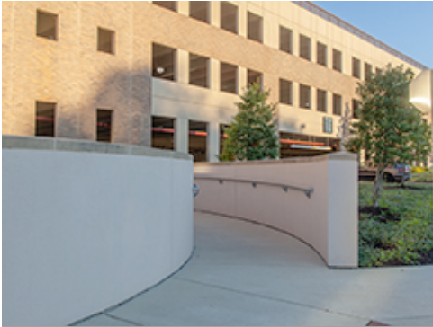
Site Ramp with Retaining Wall
