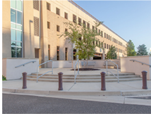
Site Stair at Group 1
