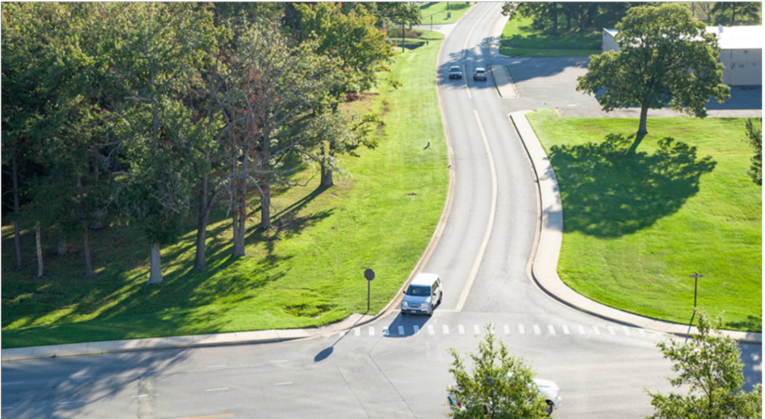
T-Intersection at F Street and Alabama Avenue
