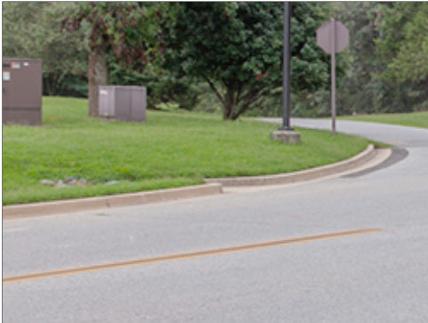
Unobtrusive Location for Cabinets
