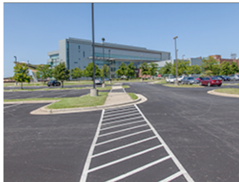
Striping Indicating Connection to Entrance
