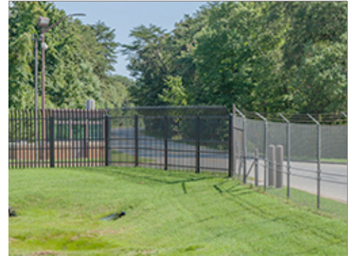
Transition from Metal to Chain Link
