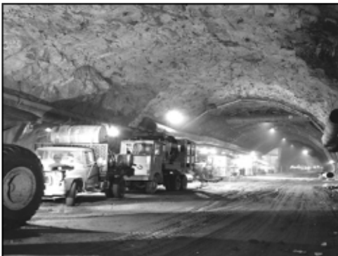
Cheyenne Mountain Complex Construction
