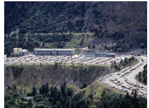
Current North Portal Entrance
