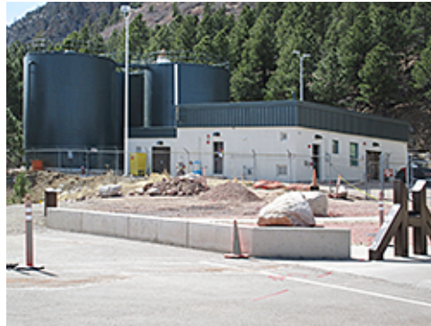
Coordinated Facilities and Equipment
