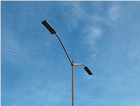
Double Arm with LED Lamping
