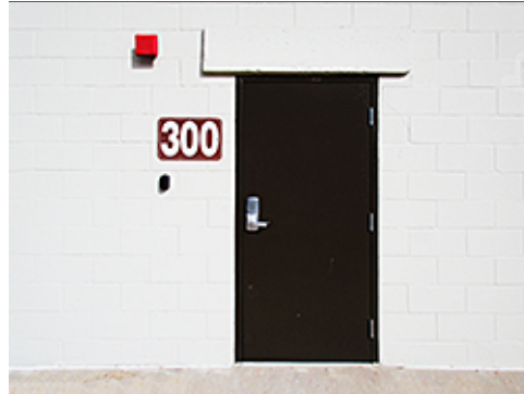
Building Number Sign Placement
