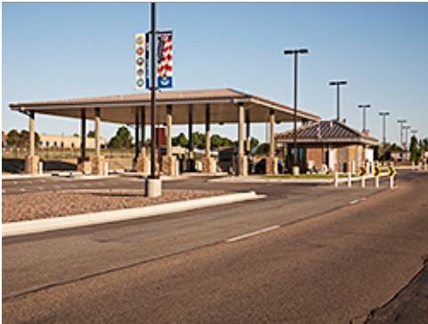
Buried Utilities at Group 1
