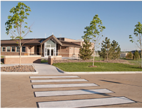
Alignment with Main Entrance
