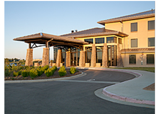
Porte Cochere at Group 2 Lodging
