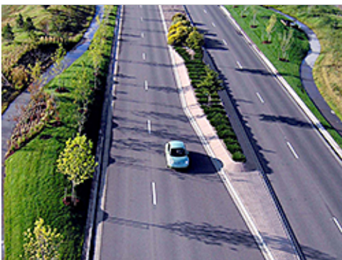
Street with Integrated Stormwater System
