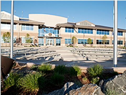
Concrete Paving at Plaza
