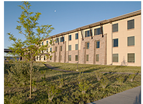
Trees and Shrubs near Building Entrance
