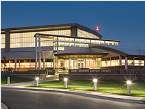
Coordinated Site and Facility Lighting
