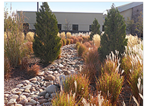
Rock Mulch at Drainage Swale
