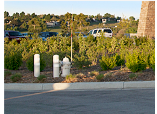
Hydrant at Group 2
