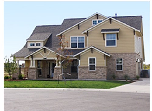
Group 4 Architectural Features
