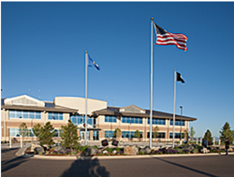
Group 1 Architectural Features
