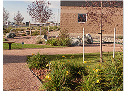
Pervious Paving Adjacent to Plantings
