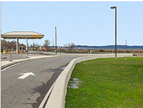
T Intersection at Gate
