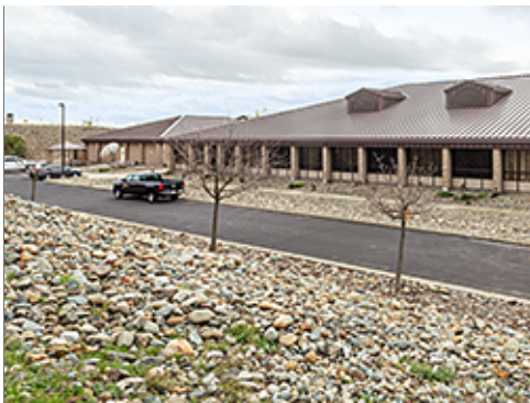
Local Street in Group 2
