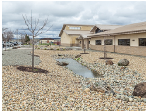
Rock Mulch Retention Area
