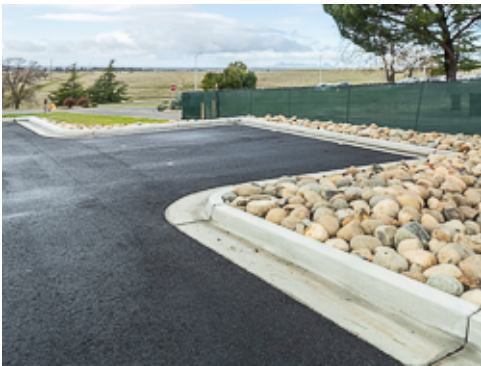
Asphaltic Concrete Paving
