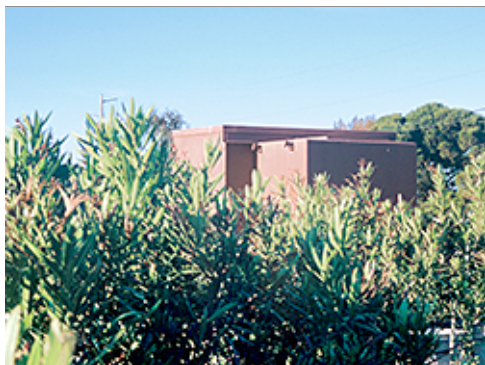
Screening of Utility Cabinet
