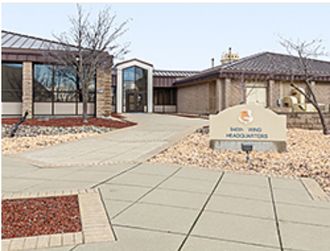
Sidewalk and Entrance Plaza at Group 1
