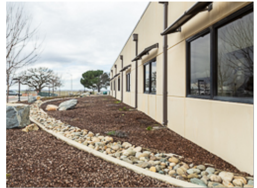
Roof Drainage as Irrigation
