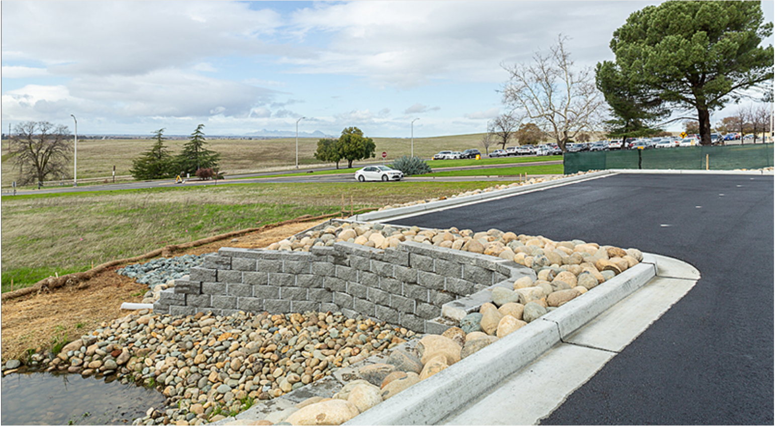
On Site Stormwater System
