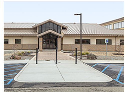
Concrete and Unit Pavers at Group 2
