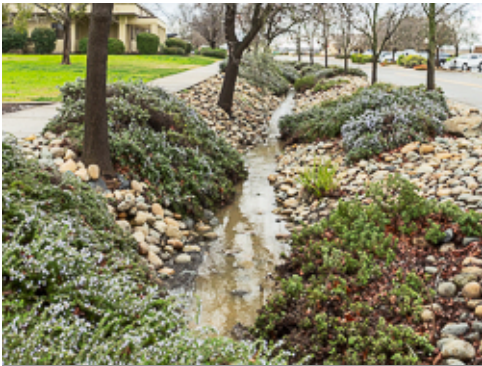
Bioswale Providing Irrigation
