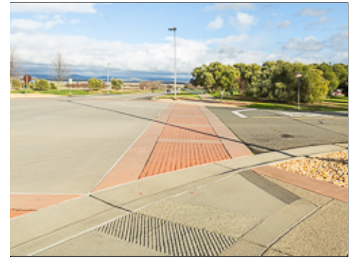
Decorative Pavers and Edging at Group 1
