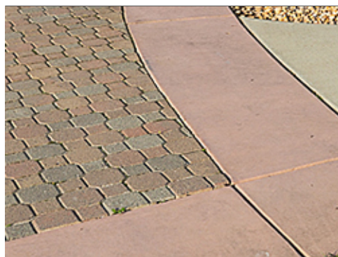
Interlocking Pavers and Concrete Edging
