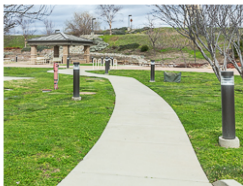
Bollards with Protective Bases
