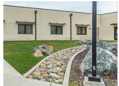
Defined Drainage Area and Mulched Bed
