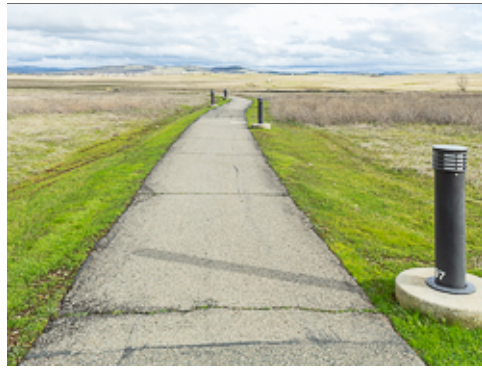
Asphaltic Concrete Paving at Trail
