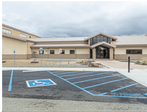
Blue Striping at Accessible Parking Stalls
