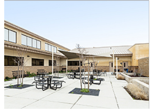
Roof Collection to Underground System
