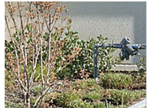
Landscape Screening at Water Service
