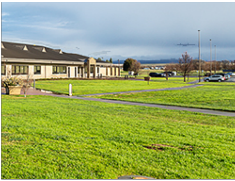
Building Expansion Area
