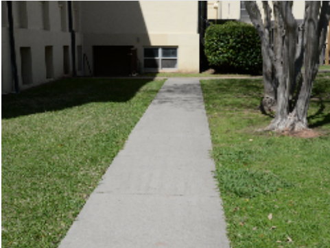
Typical Concrete Paving
