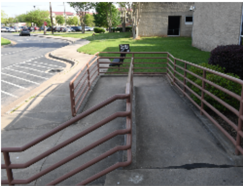
Typical U-Shaped Ramp
