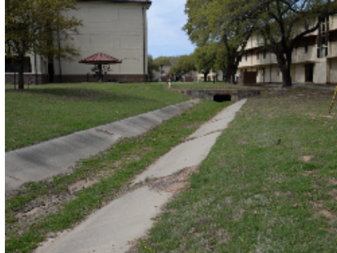
Concrete Drainage Swale
