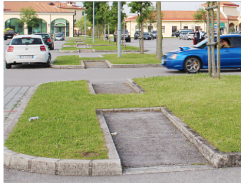
Ramps for Walkway
