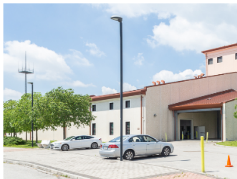
Medium Height Mast Lighting
