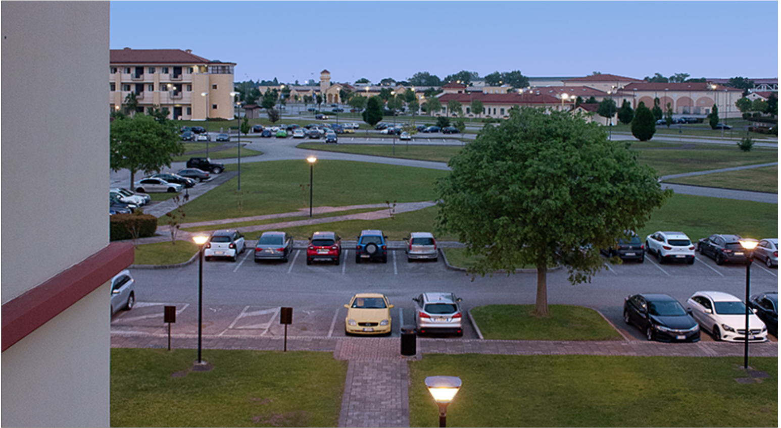
Parking Lot Lighting
