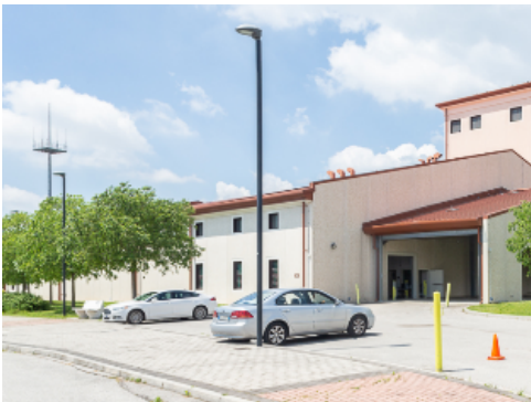
Pole Lighting at Street
