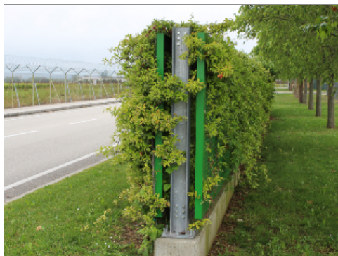
Vines in Mesh Screen Entry
