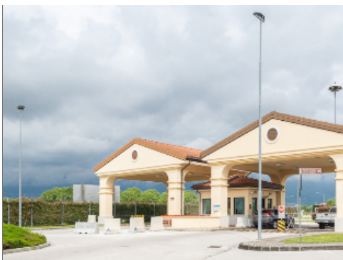
Tall Mast Lighting
