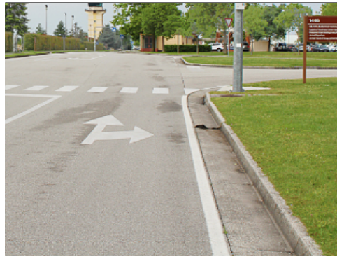
Concrete Curb and Gutter
