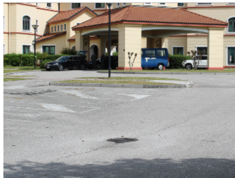
Drain in Parking Lot
