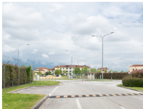
Shrubs Line Perimeter Fence
