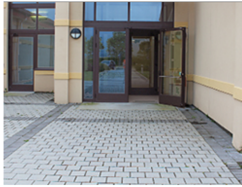
Walk outside Building
