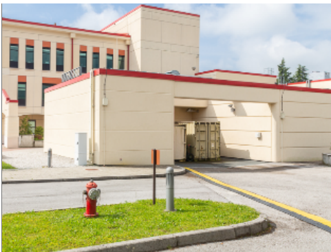
Hydrant in Median
