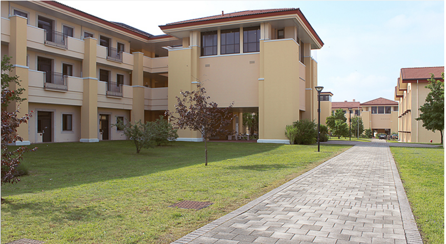
Walk through Dormitory Area
