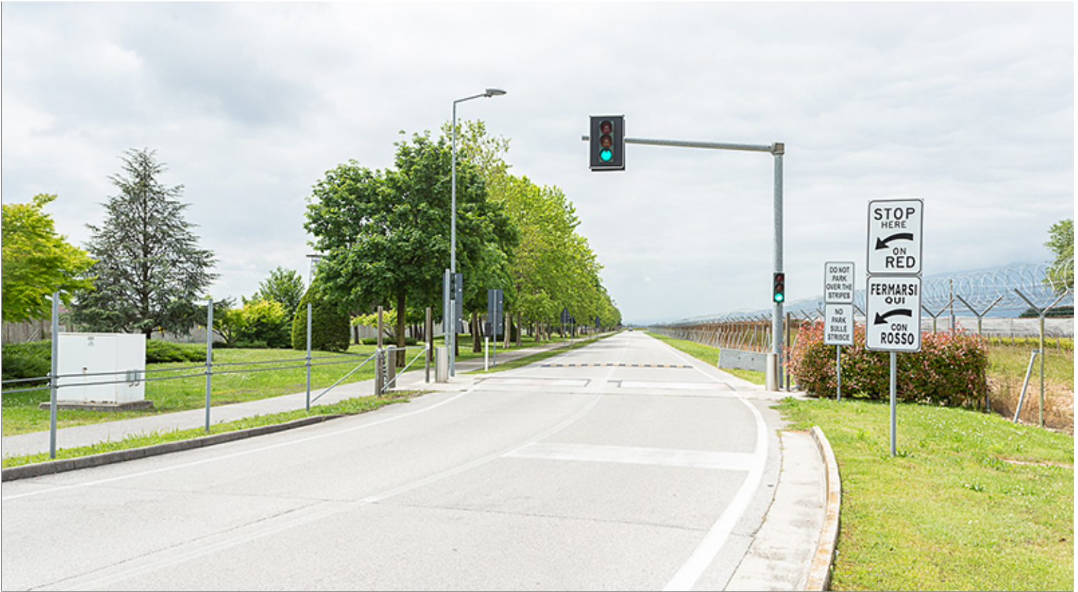
Signal at End of Runway
