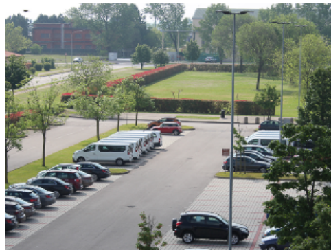
Pole Lighting at Parking Lot
