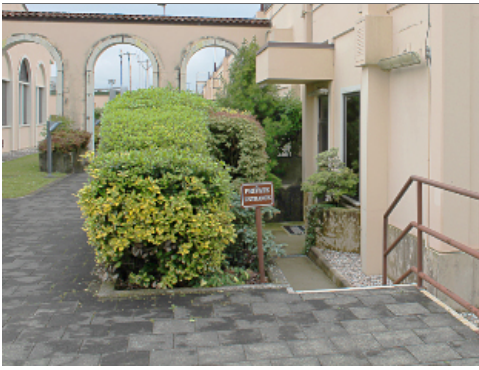
Stair at Headquarters
