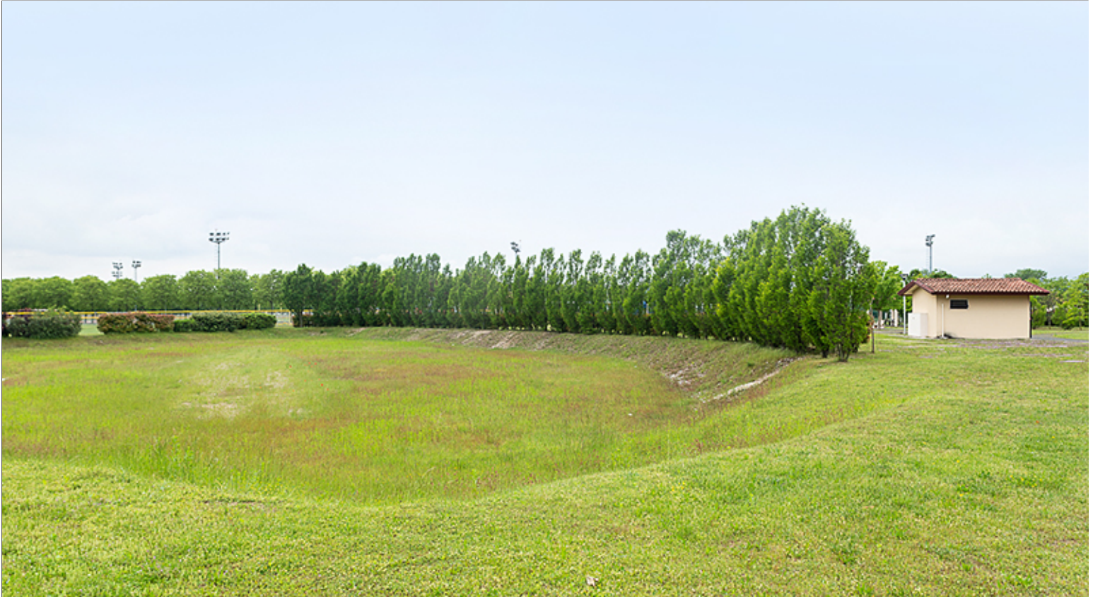
Basin for Slowing Water Discharge
