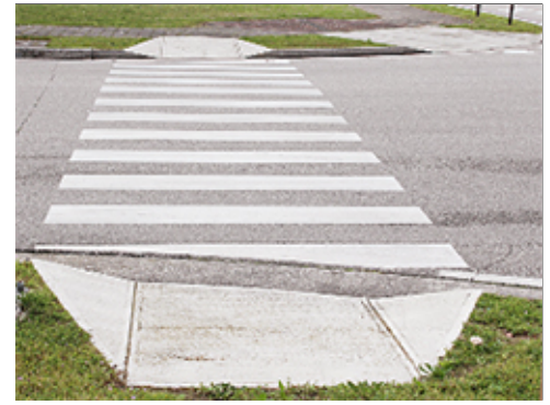
Ramp at Crosswalk
