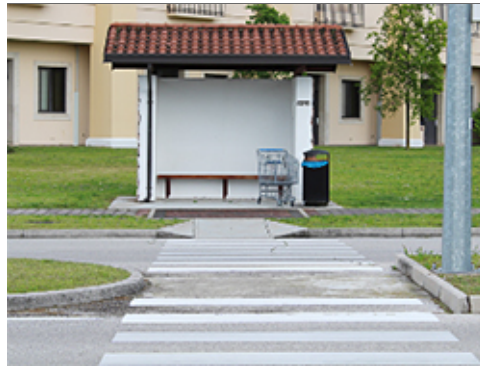
Ramp at Bus Stop
