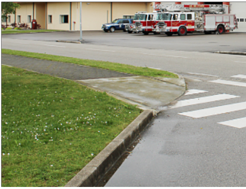
Curb Ramp at Crosswalk
