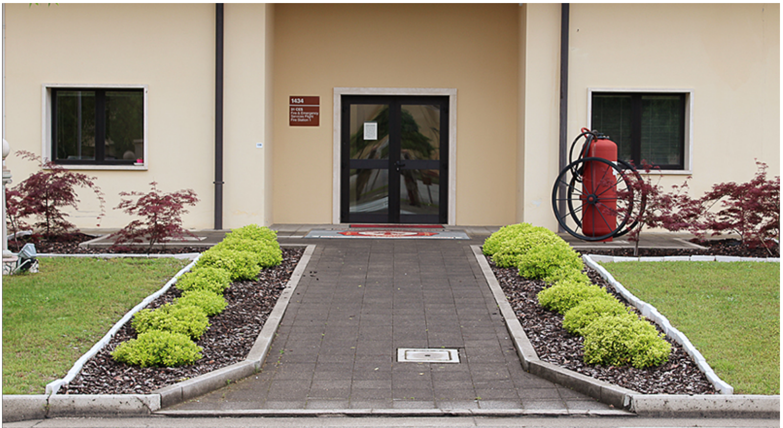
Ramp at Fire Station Entry
