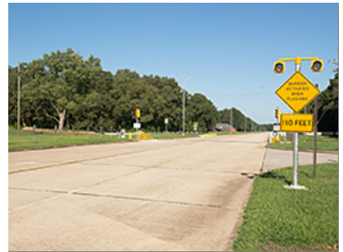
Operable Barrier Near Gate
