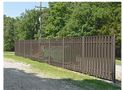
Metal Screen Wall
