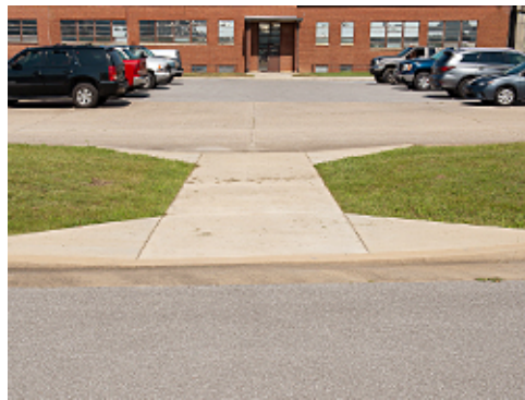
Alignment with Main Entrance
