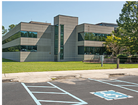
Accessible Parking Area Striping
