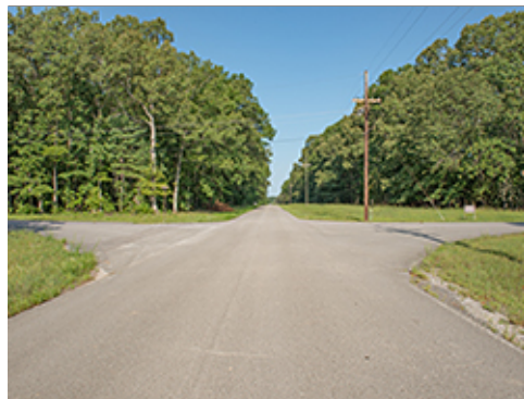
Overhead Utility Lines near Group 3
