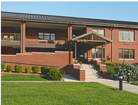
Stair and Ramp at Building Entrance
