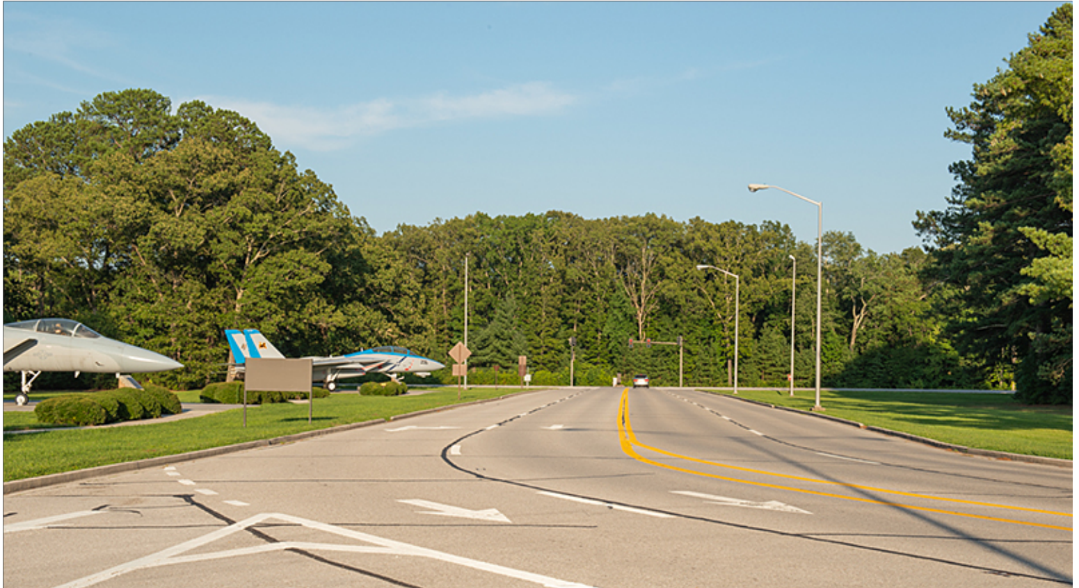
Installation Elements: Base-wide Infrastructure
