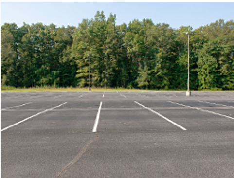
Bituminous Paving with White Striping
