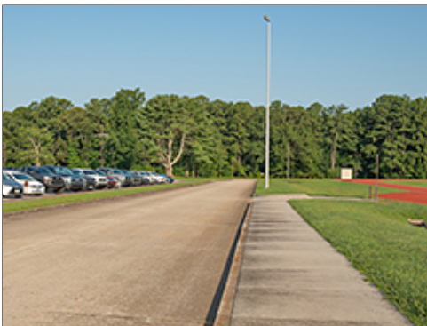
Buried Electric Service Lines near Group 2
