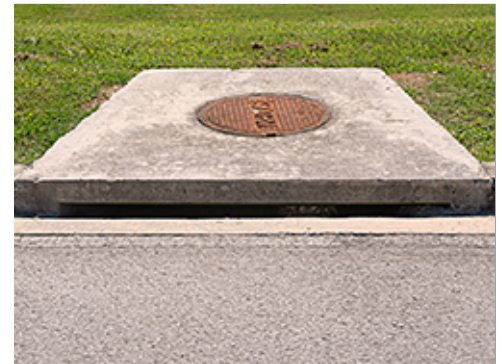
Drainage Element Intergrated with Gutter
