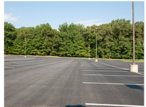
Integrated Light Fixtures and Bases
