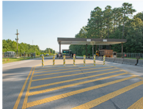
Barriers near Gate
