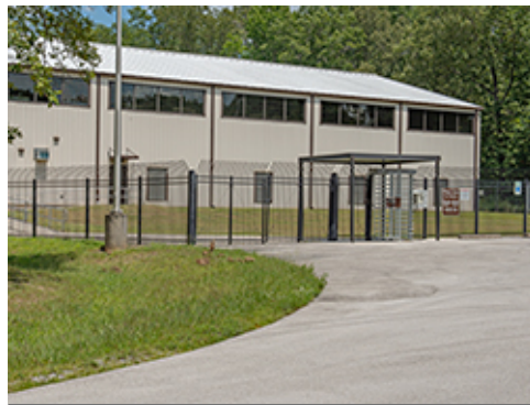
Security Fence and Controlled Access
