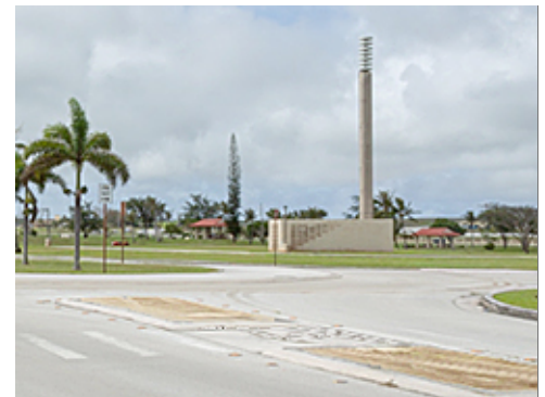
Colored Concrete Pavers at Median
