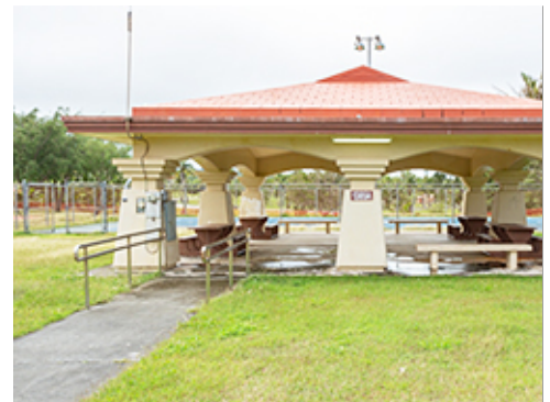
Ramp at Picnic Plaza
