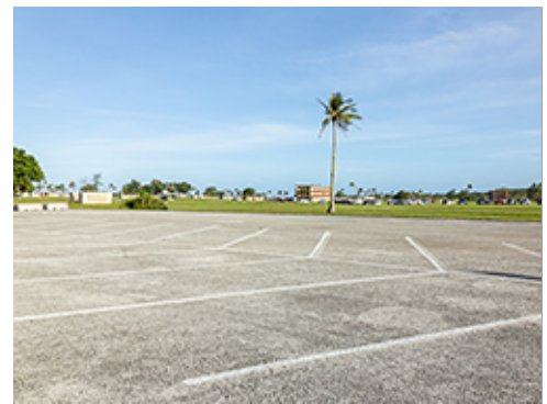
Asphaltic Concrete with White Striping
