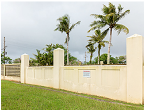
Perimeter Fence at Main Gate
