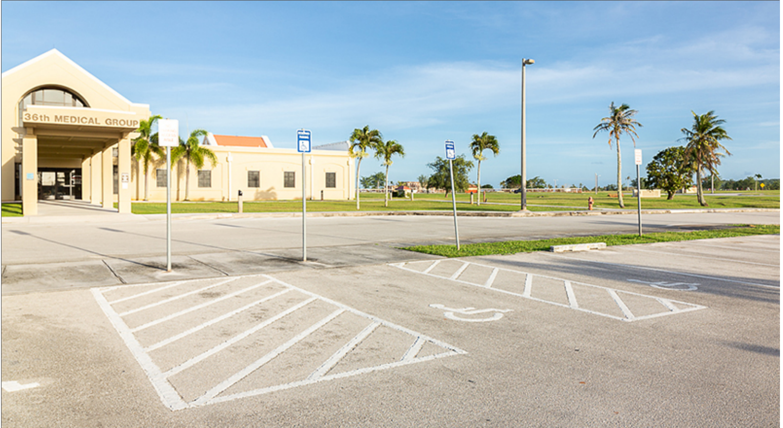
Direct Link to Main and Secondary Entrances
