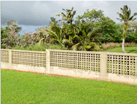
Perimeter Fence at Main Gate
