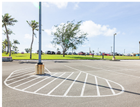
Asphaltic Concrete with White Striping
