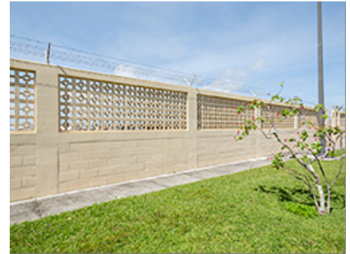
Perimeter Fence at Group 3
