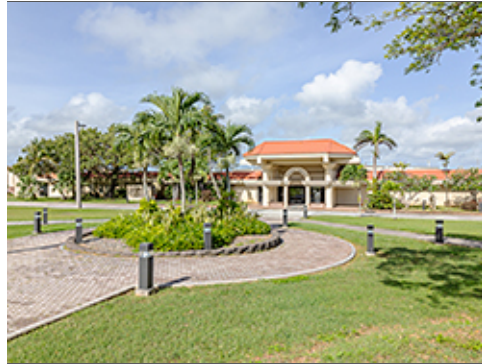
Lighted Bollards Defining Sidewalk
