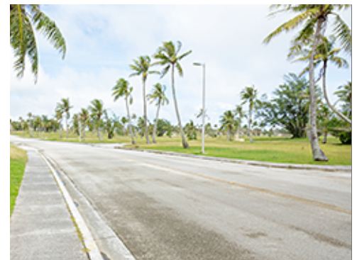
Sidewalk on Single Side
