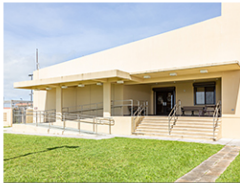
Ramp and Stair at Entrance
