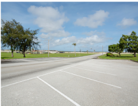
Asphaltic Concrete with White Striping
