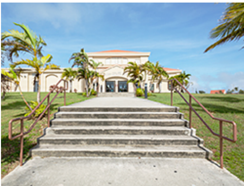
Site Cast Stair at Entrance
