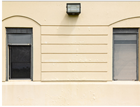
Wall Mounted Fixture Group 2
