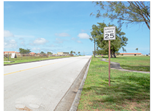
Traffic Control Sign
