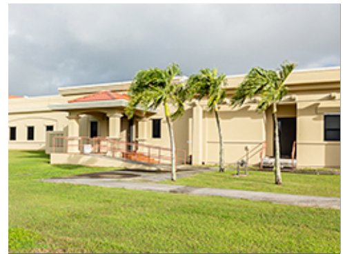
Ramp and Stair at Entrance
