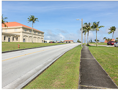
Bituminous Pavement and Asphaltic Path
