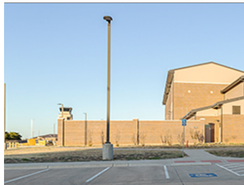
Fixtures at Group 3
