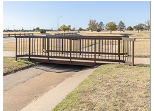
Paved Drainage with Bridge as an Amenity
