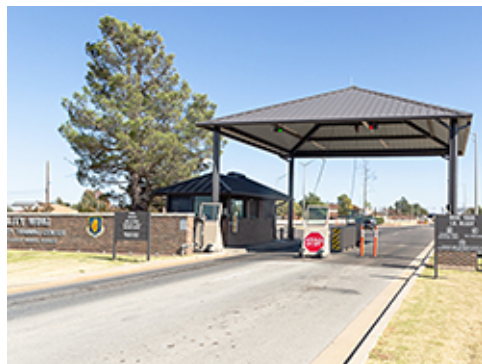
Trees and Grasses at Entry Gate
