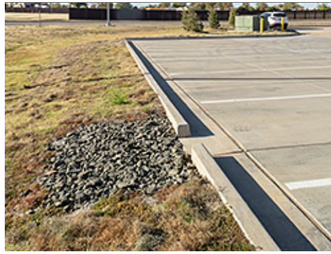
Parking with Rip Rap at Stormwater Outlet
