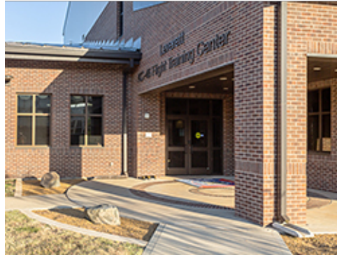
Roof Drainage Directed through Rock Mulch
