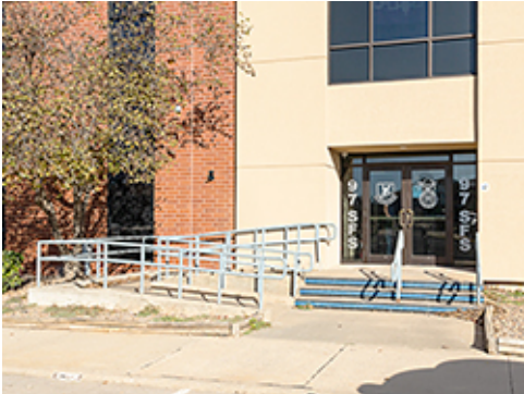
Ramp and Stair at Entrance
