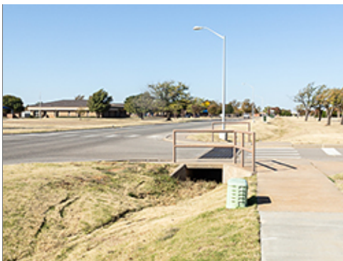
Engineered Culvert and Channel
