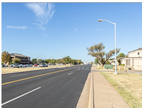
Attached Sidewalk on Single Side of Street
