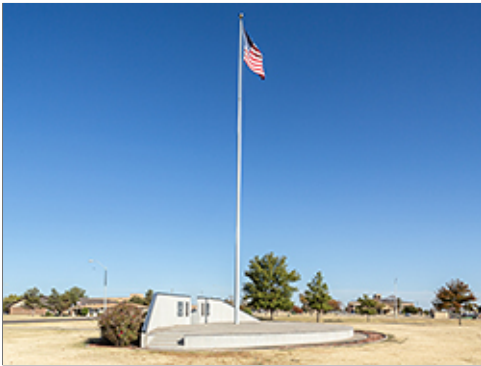
Concrete Plaza at Display
