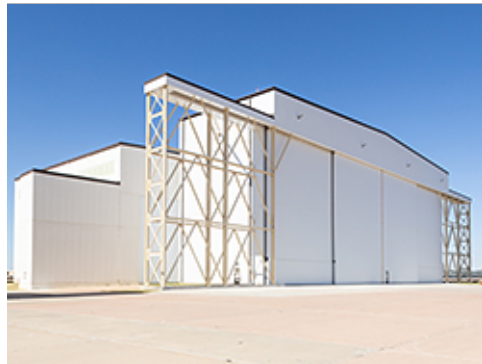
Group 3 Three-Bay Hangar
