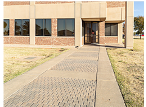
Decorative Paving at Group 1
