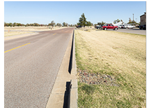
Curb and Gutter with Drainage
