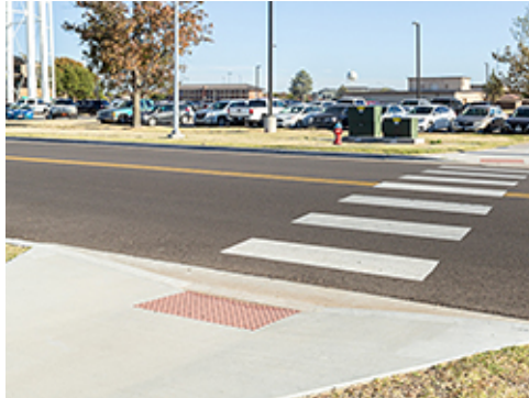
Curb Ramp at Crosswalk
