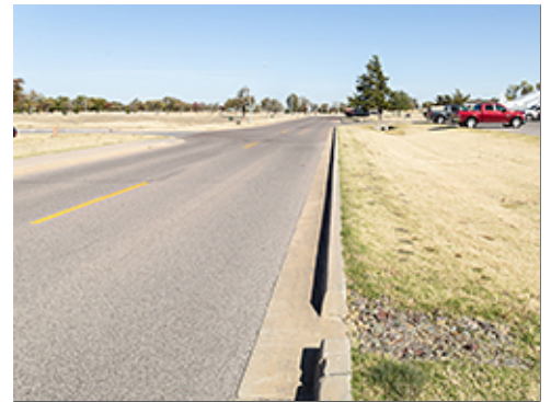
Curb and Gutter
