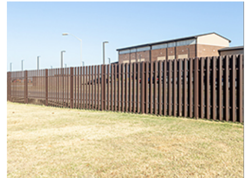
Metal Fence near Group 3
