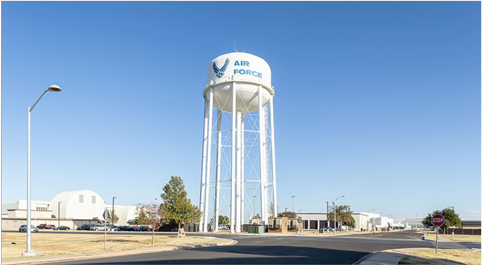
Altus Water Tower
