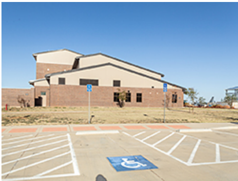
Accessible Parking Space Striping
