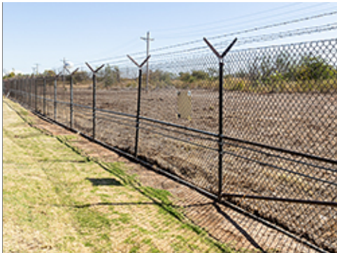
Chain Link Fencing at Perimeter
