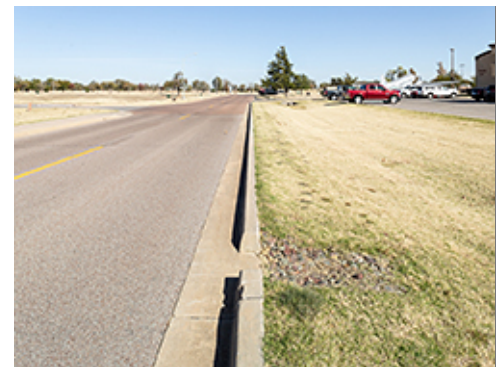
Curb and Gutter with Storm Water Drainage
