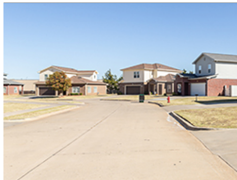
Paving at Family Housing
