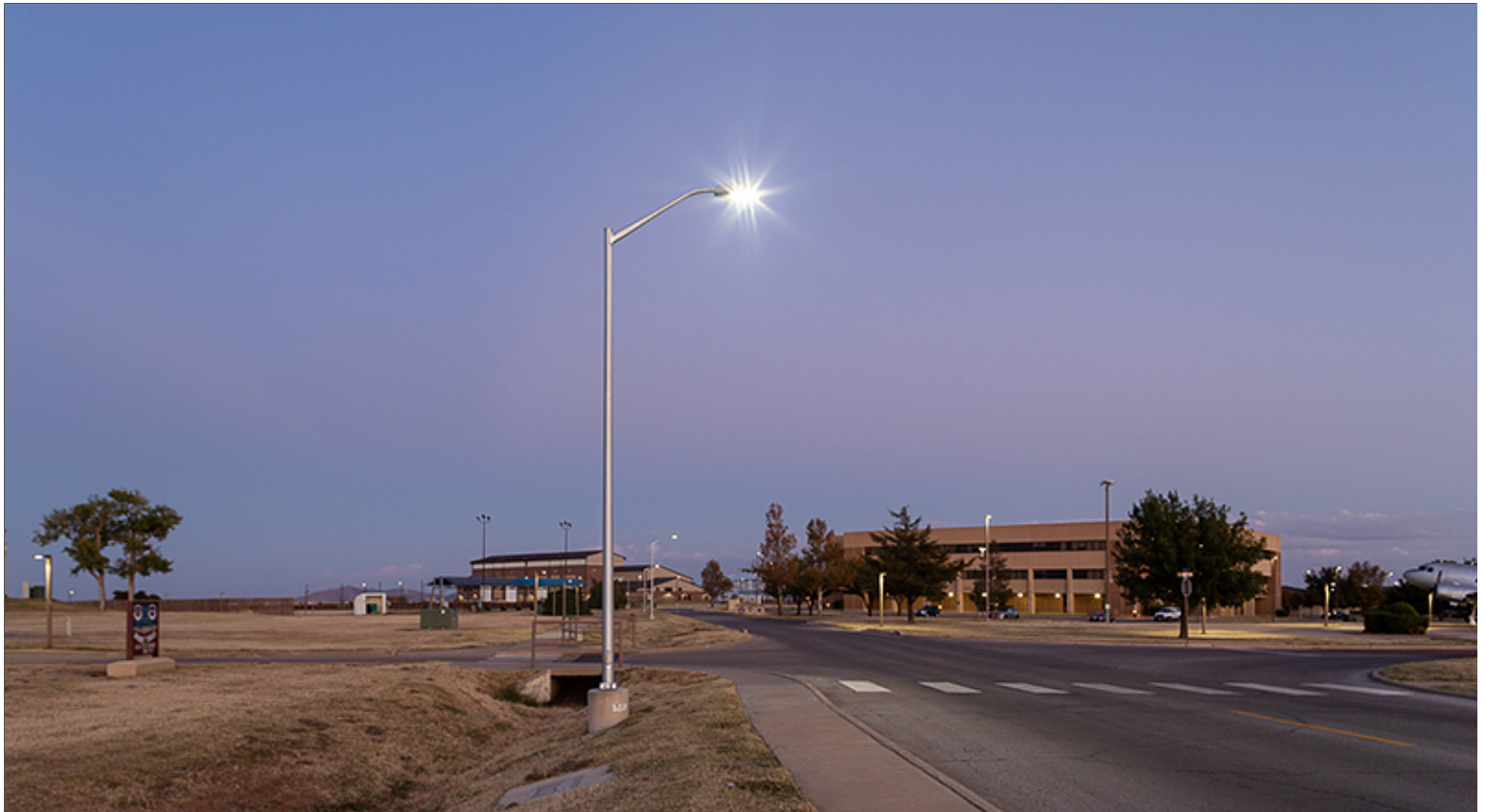
Street Lighting at Crosswalk
