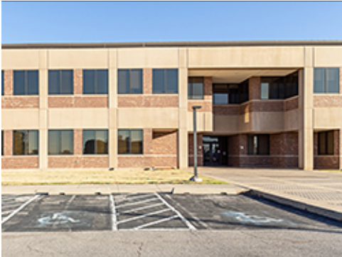
Direct Link to Main and Secondary Entrances
