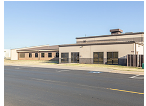
Accessible Parking Adjacent to Building
