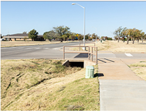
Stormwater Providing Irrigation
