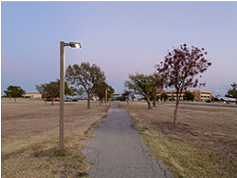
Fixture along Walking Trail
