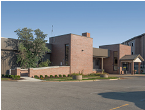
Flat Roofed Elements Defining Entrance
