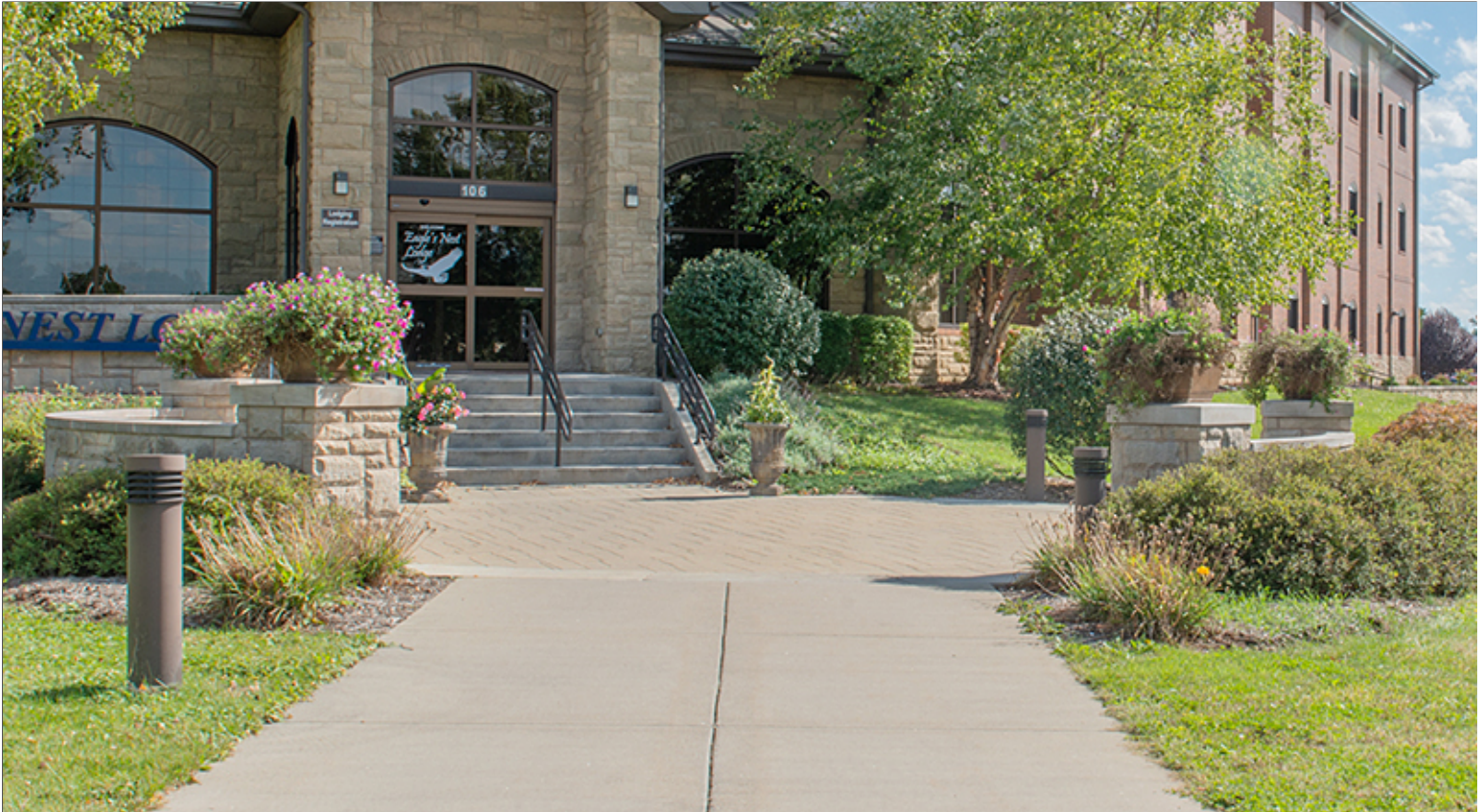
Tan Colored Concrete at Group 2
