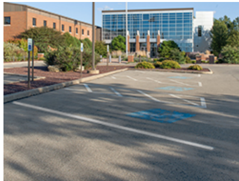
Accessible Parking Striping and Graphics
