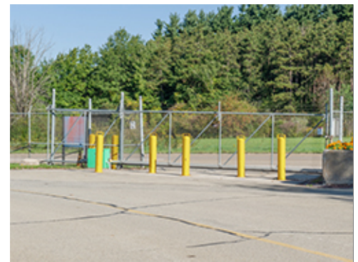
Fencing with Gate System
