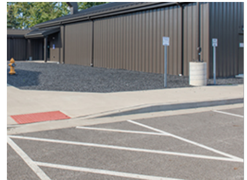
Aisle and Curb Ramp
