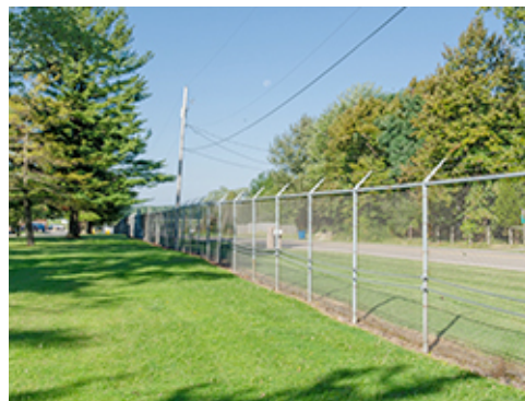
Overhead Utility Lines
