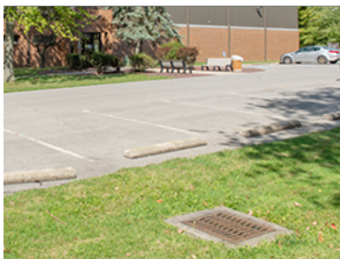
Site Grading to Inlet
