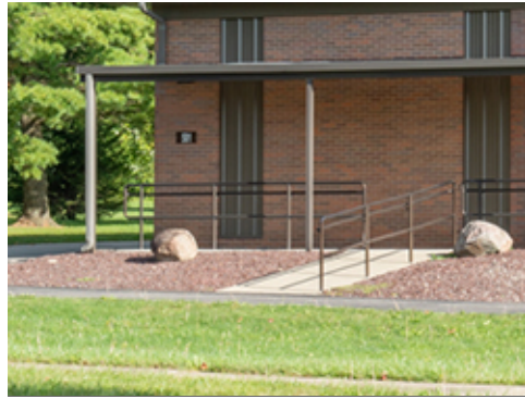
Site Ramp with Railing
