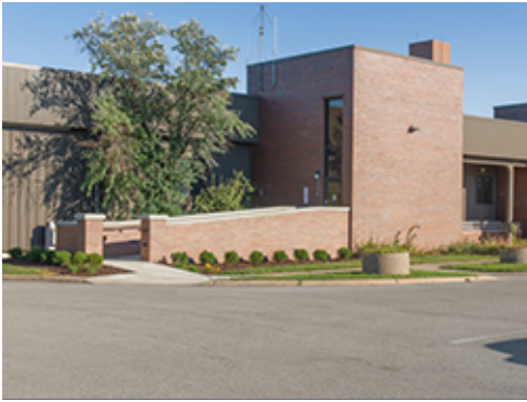
Ramp with Masonry Walls
