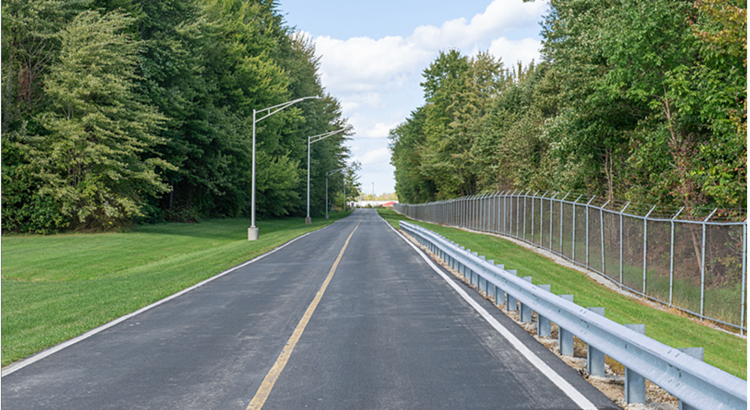
Route along Perimeter Fence
