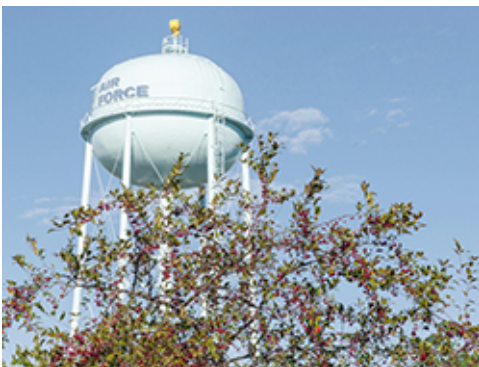
Water Service Element
