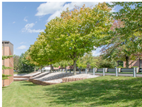
Slope Stabilized with Rock Mulch
