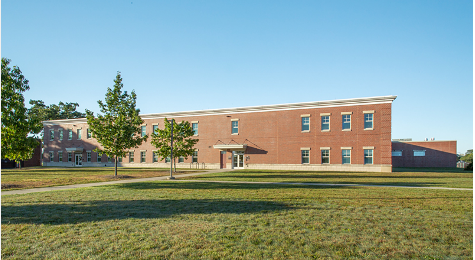
Standard Red Blend Brick with Accents at Base, Lintels and Sills
