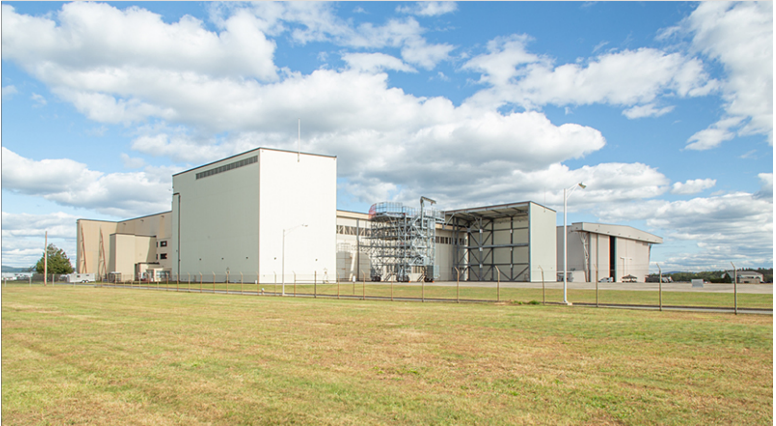
Group 3 Industrial Facilities along Flightline
