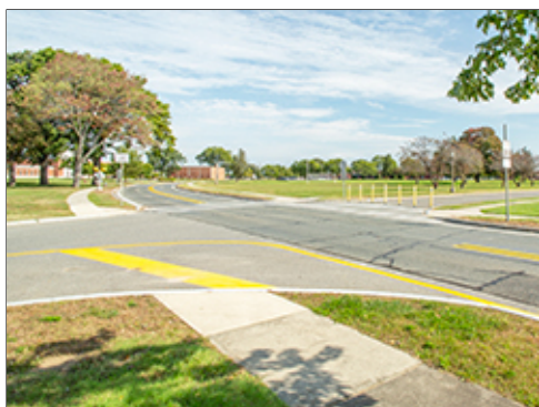
Standard Street Markings
