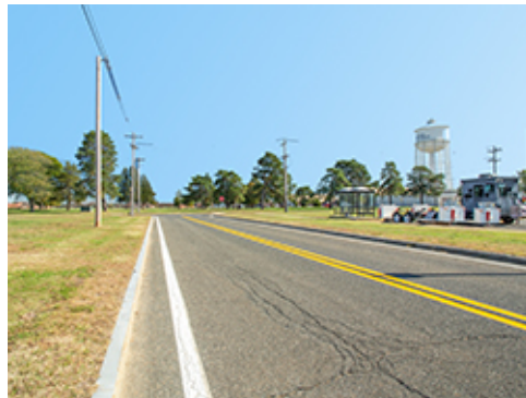
Integrated Overhead Utilities
