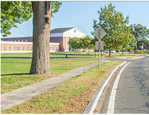
Detached Sidewalk near Group 1
