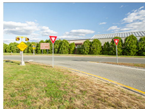
Organized Placement of Sign
