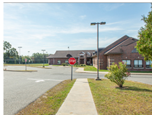
Double-Mast Fixture at Intersection
