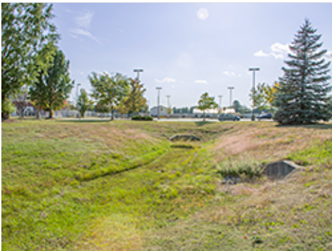
Landscaped Drainage Basin
