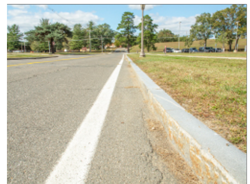
Standard Curb and Gutter
