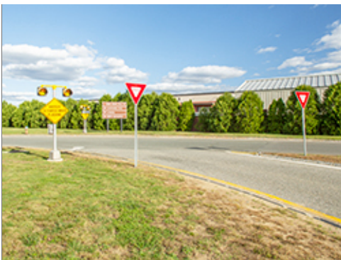
Traffic Devices at Intersection
