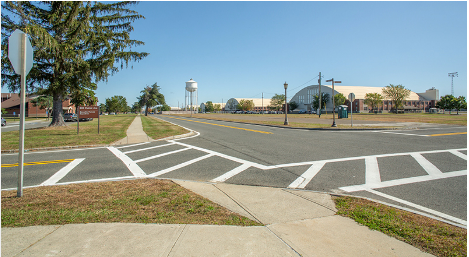
Standard Traffic Devices and Street Markings
