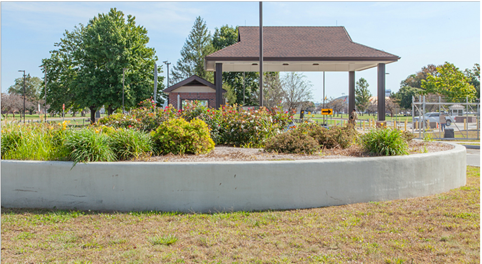
Raised Planting Bed Providing Visual Appeal and Serving Also as a Security Feature
