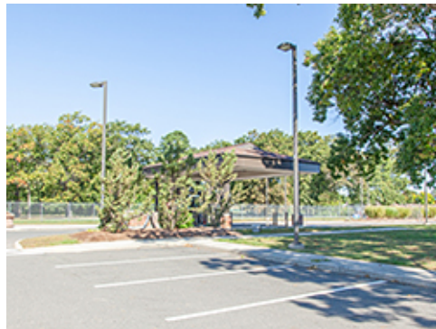
Parking Lot Fixture
