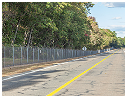
Fencing along Perimeter Road
