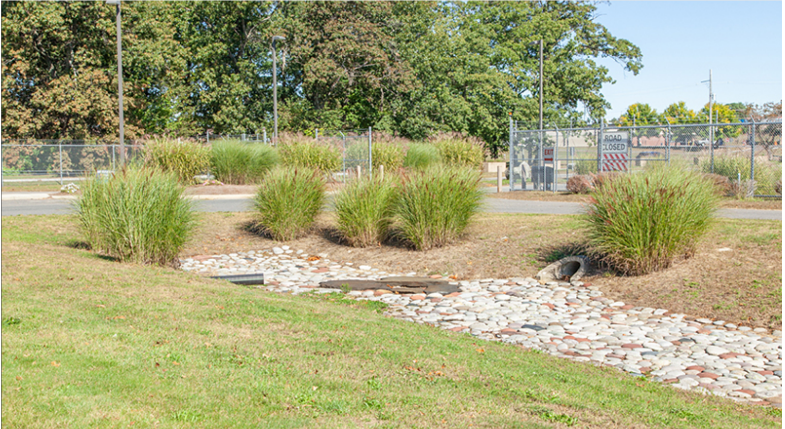
Drainage Feature with Integrated Landscape
