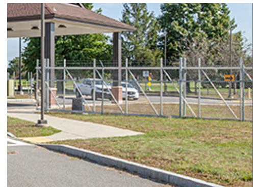
Fencing Adjacent to Gate
