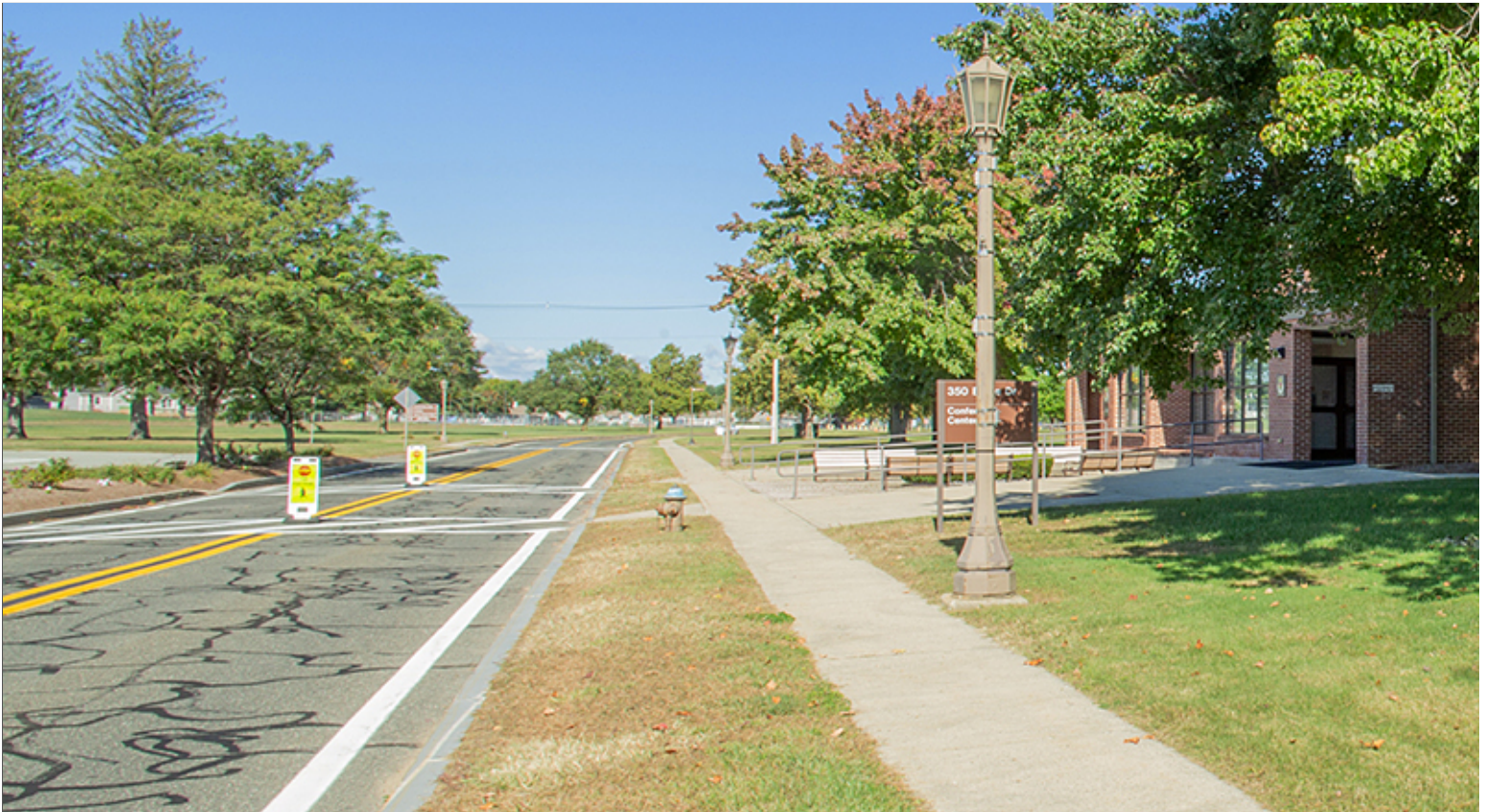
Detached Sidewalk Adjacent to Facility Group 2
