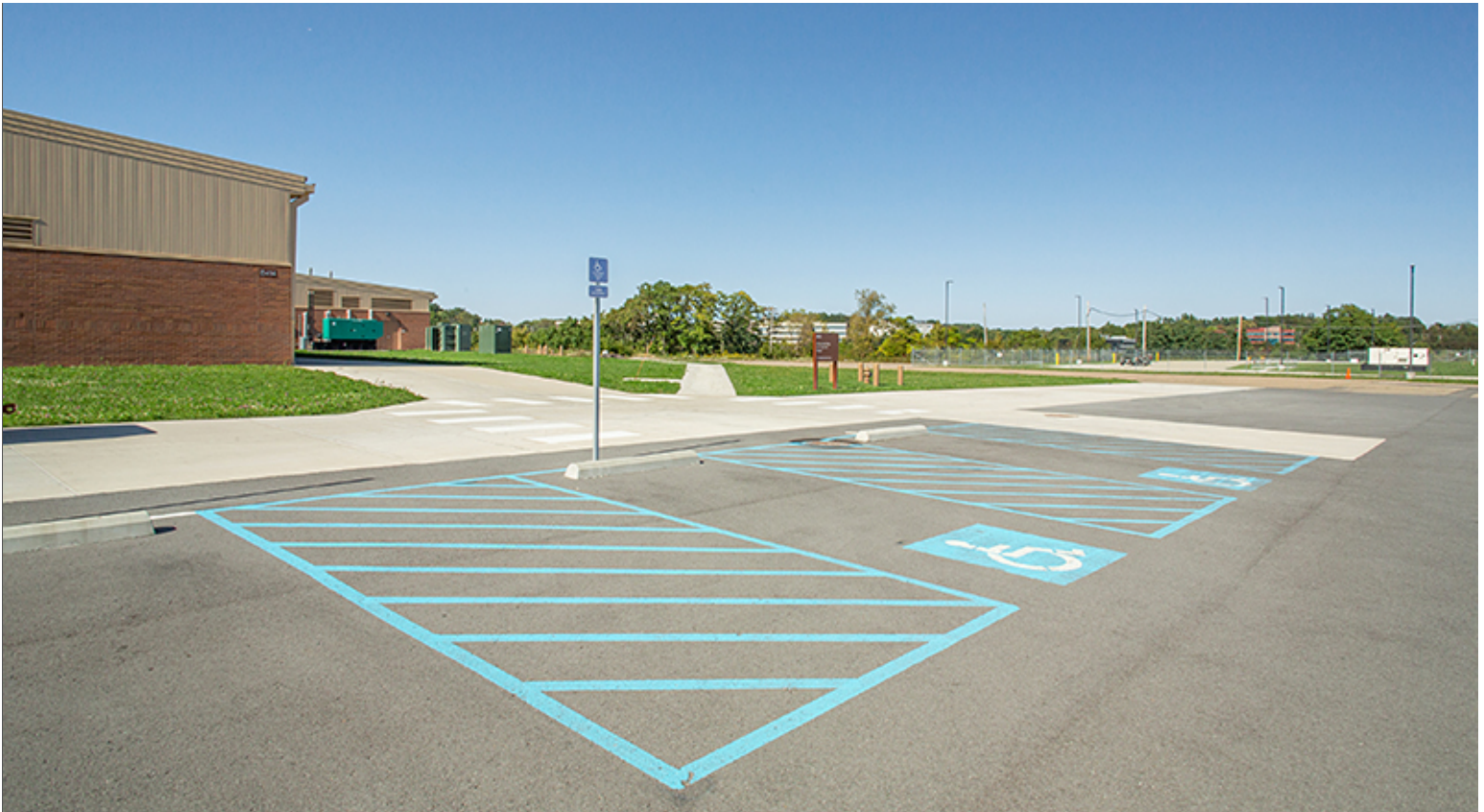
Sidewalk at Grade with Parking Lot and Direct Access to Main Entrance
