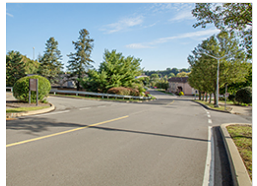
Intersection with Access to Parking
