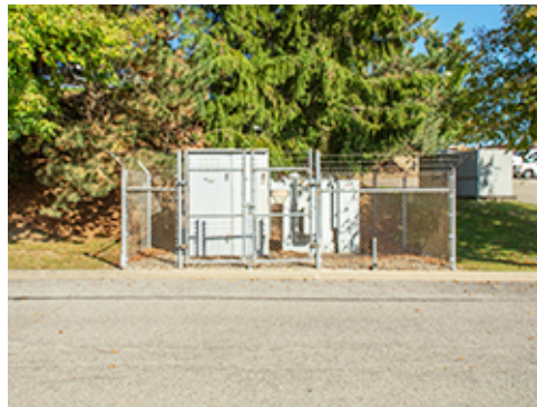
Standard Fencing at Group 3
