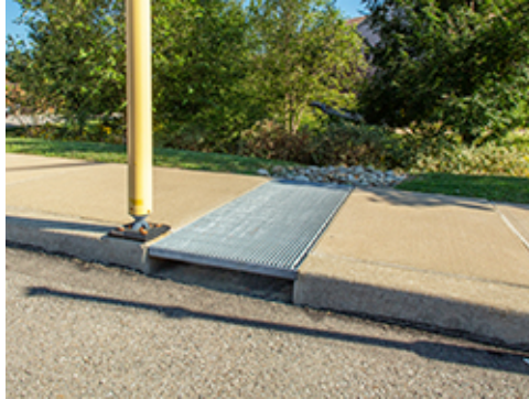
Drainage Inlet at Curb
