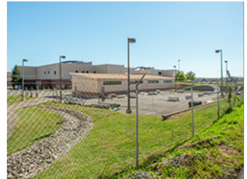
Security Fence along Group 3 Site
