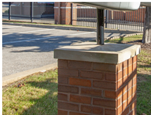
Brick Pier with Precast Cap
