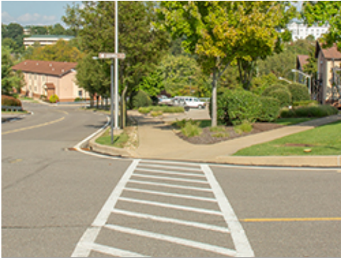
Standard Curb Ramp at Intersection
