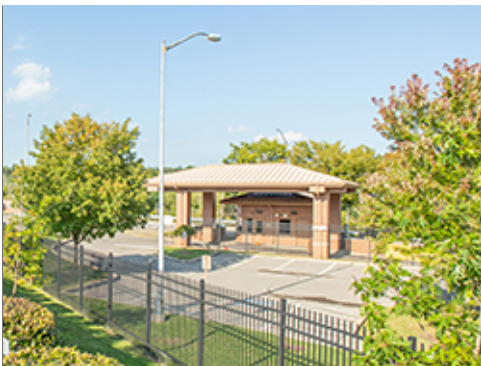
Tall Pole to Serve Street and Parking Lot
