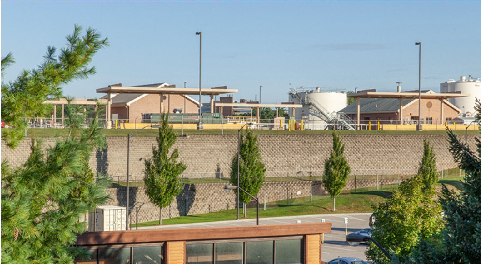
Retaining Walls Coordinated with Other Site Elements
