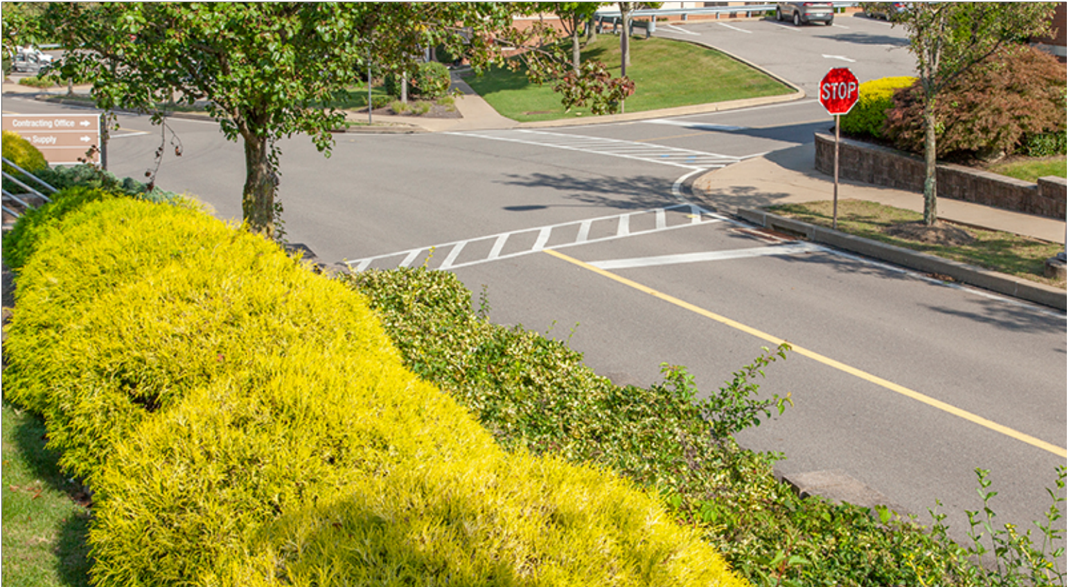
Coordinated Street Elements and Markings
