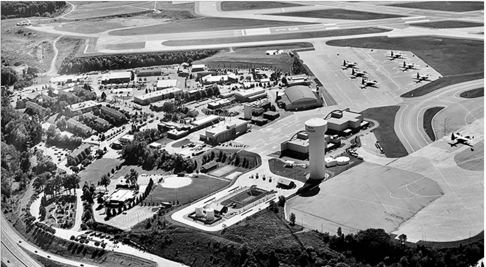
Aerial Photograph of Pittsburgh ARS Looking South
