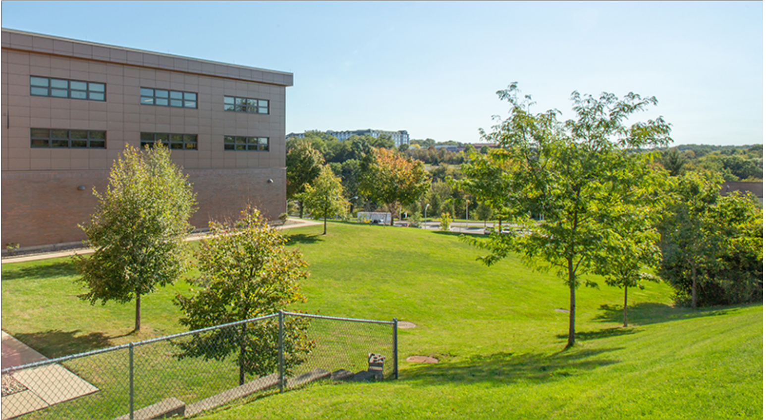
Grading to Accommodate Drainage
