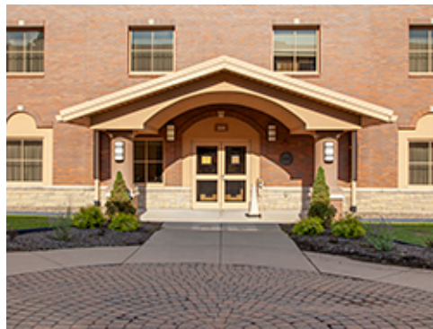
Concrete with Inset Unit Pavers
