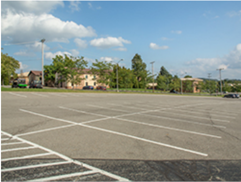
Asphaltic Pavement with White Striping
