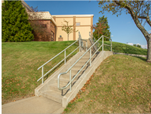
Site Stair with Landings and Railings
