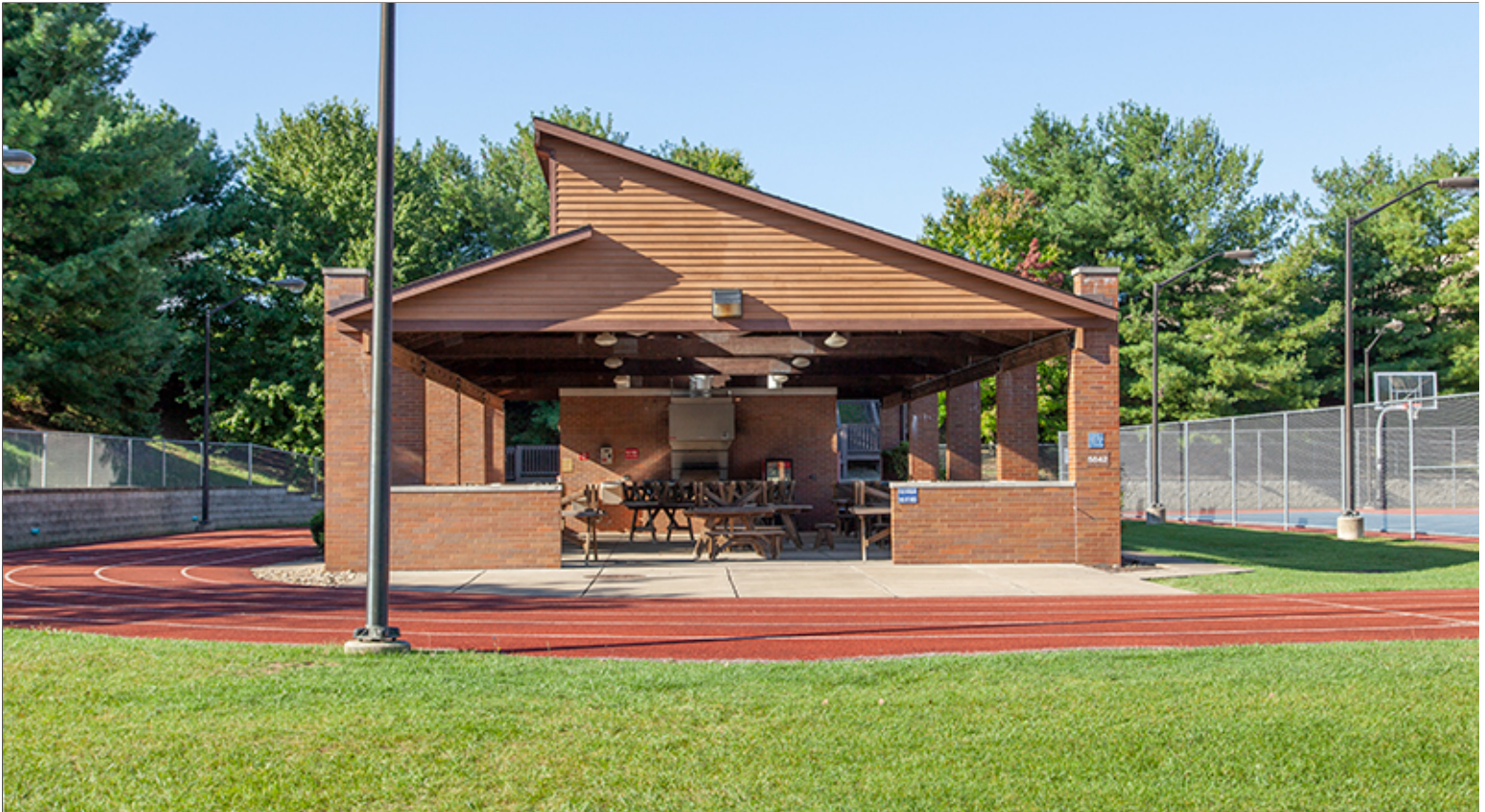
Recreation Area Picnic Pavilion
