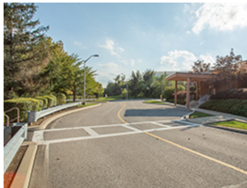
Typical Street Light
