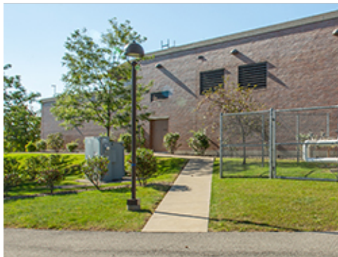
Pedestrian Scaled Lighting
