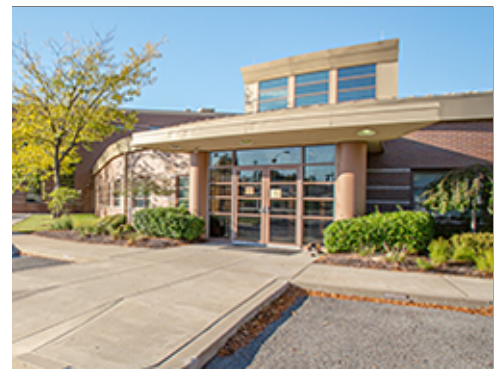
Pedestrian Scale at Entrance
