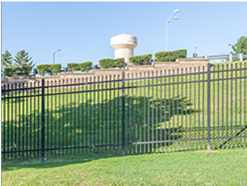
Metal Fence at Group 1
