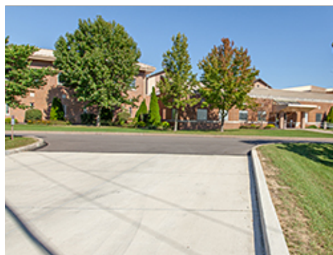
Transition in Street Paving
