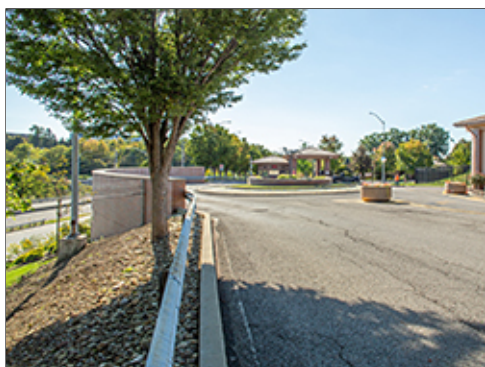
Integrated Landscape Retaining Wall
