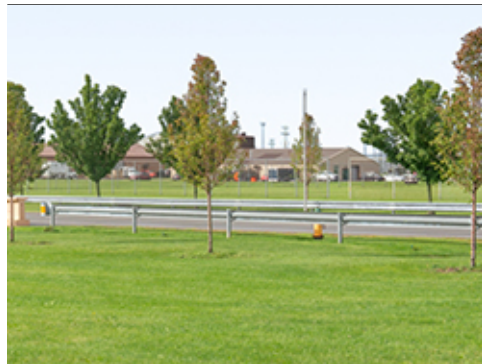
Guardrail Controlling Access
