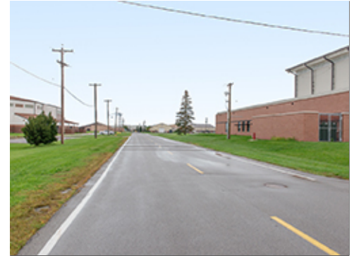
Overhead Electric Distribution at Group 2
