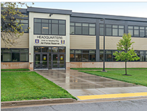
Concrete Entrance Plaza at Group 1
