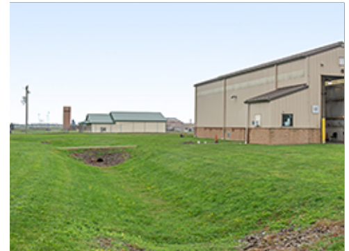
Basin with Drainage Element
