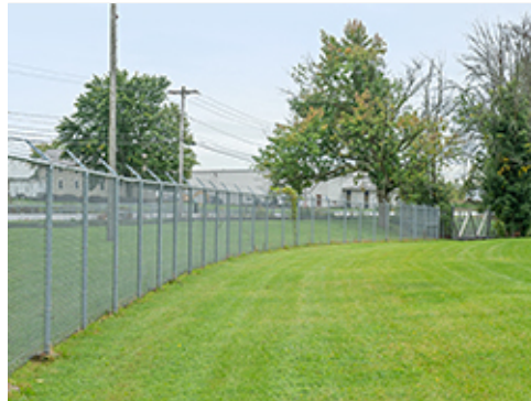
Chain Link Fencing at Group 3
