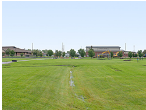
Basin with Vegetated Swale
