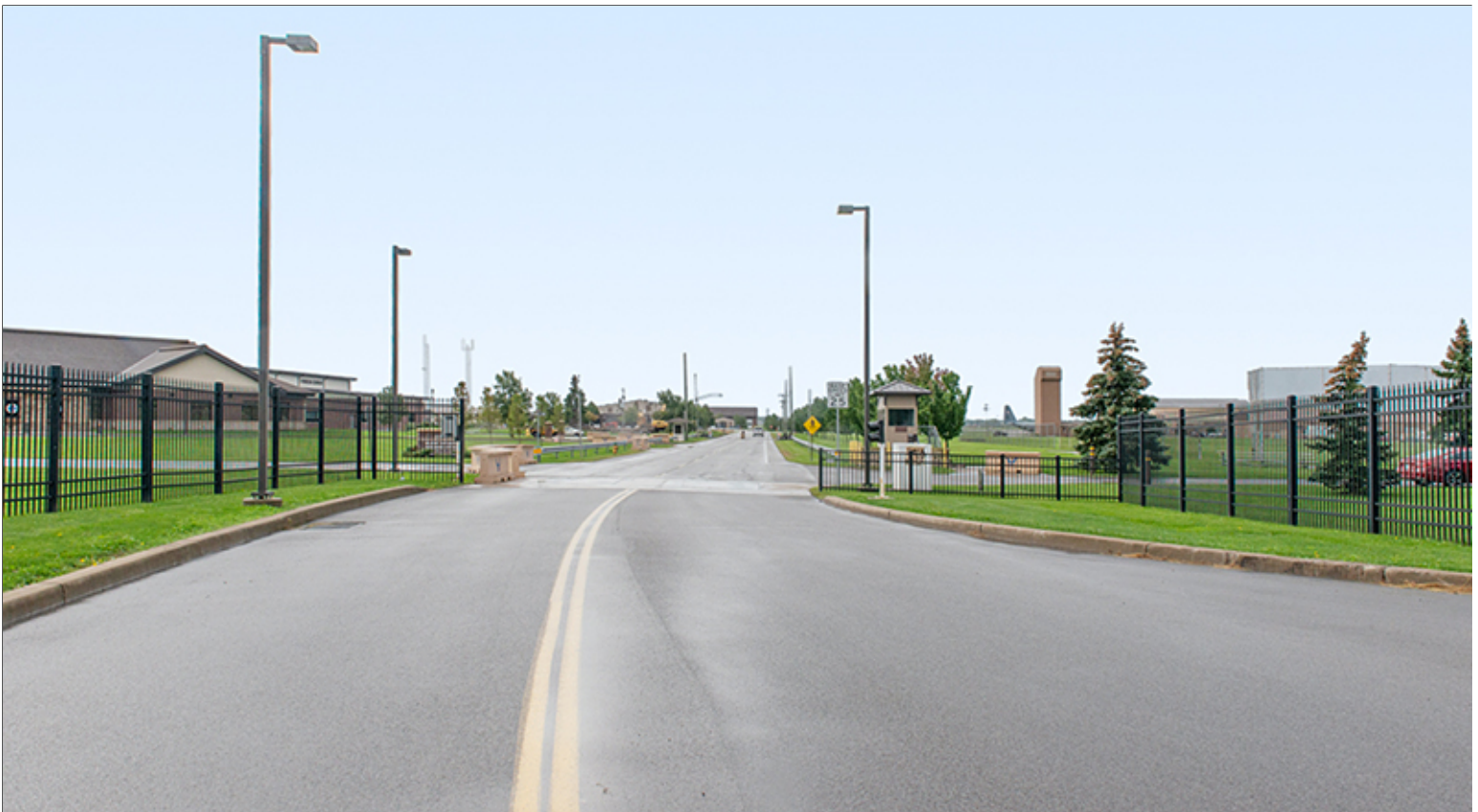
Intersection with Integrated Security Fencing Adjacent to Group 1 Main Gate
