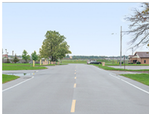
Typical Street Markings
