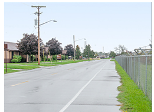
Local Street Adjacent to Perimeter Fence
