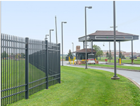
Metal Fence Adjacent to Group 1
