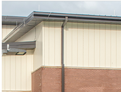
Metal Panels with Masonry Base
