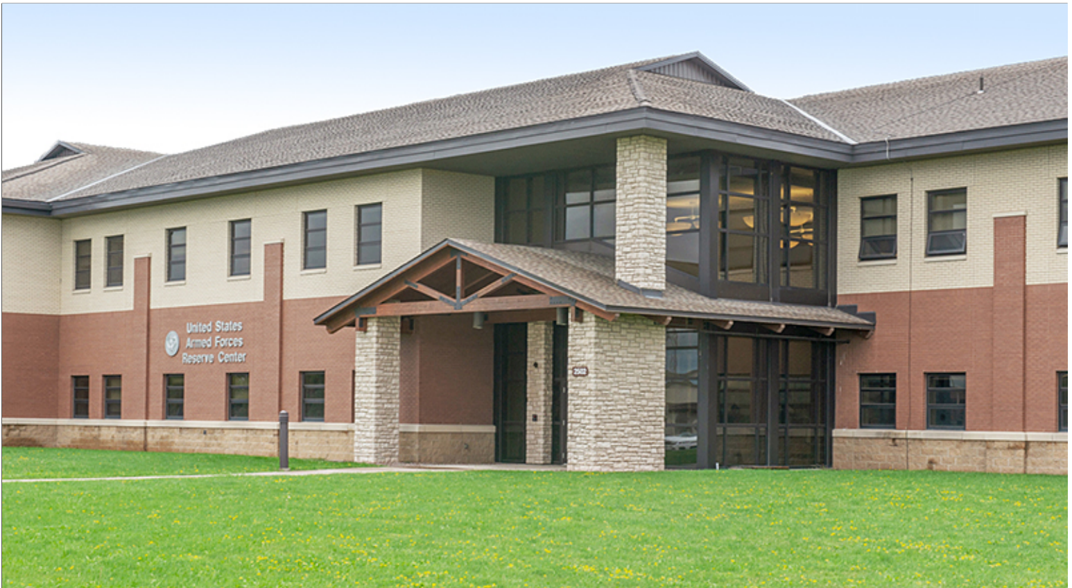
Regional Vernacular Theme with Functional Architectural Features for Shading and Weather Protection
