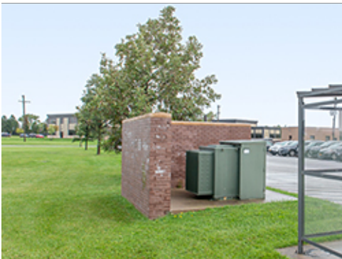
Masonry Screen Wall at Utility Element
