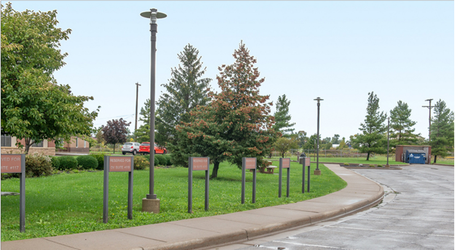
Buried Utility Service Lines at Group 2
