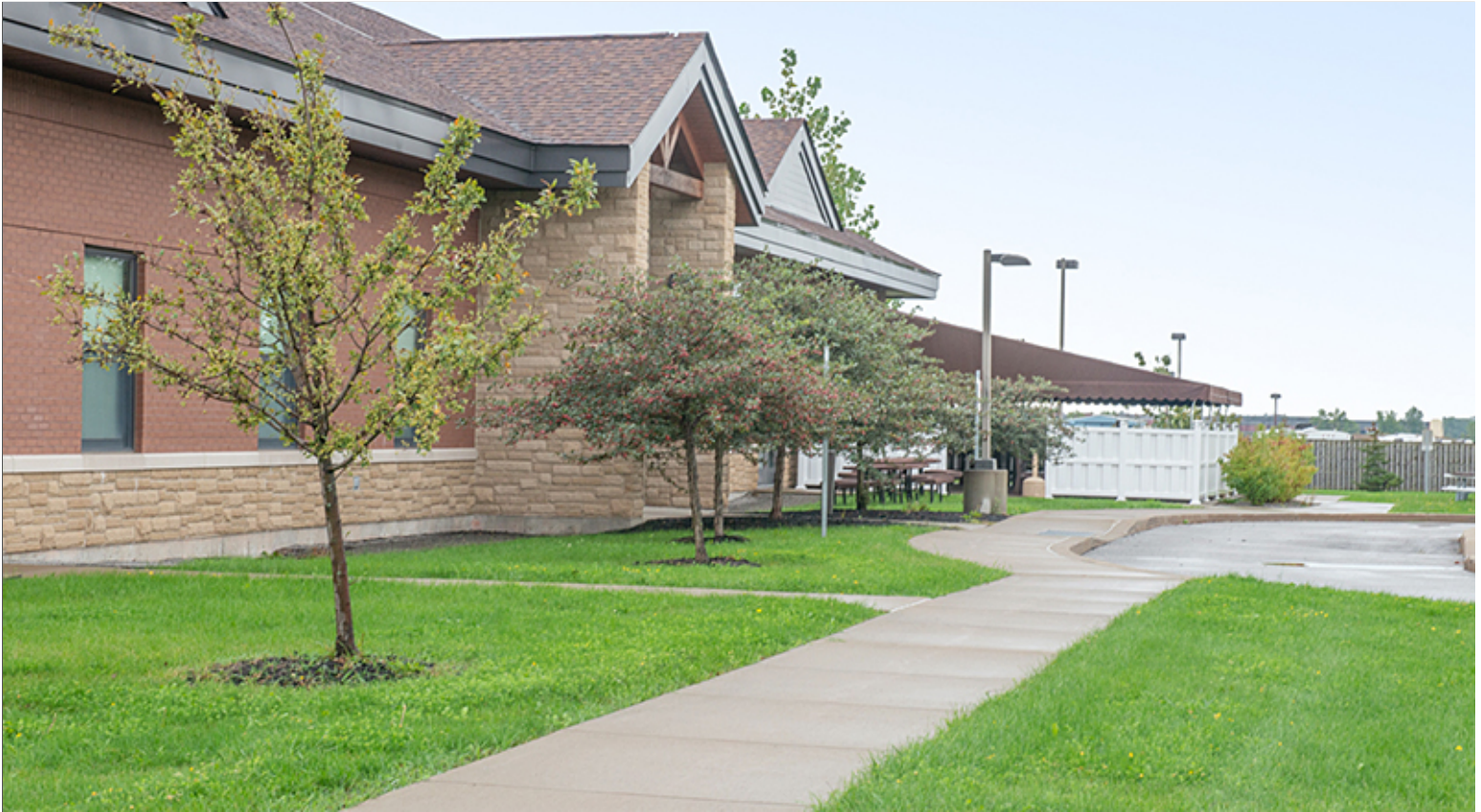
Concrete Paving at Group 2
