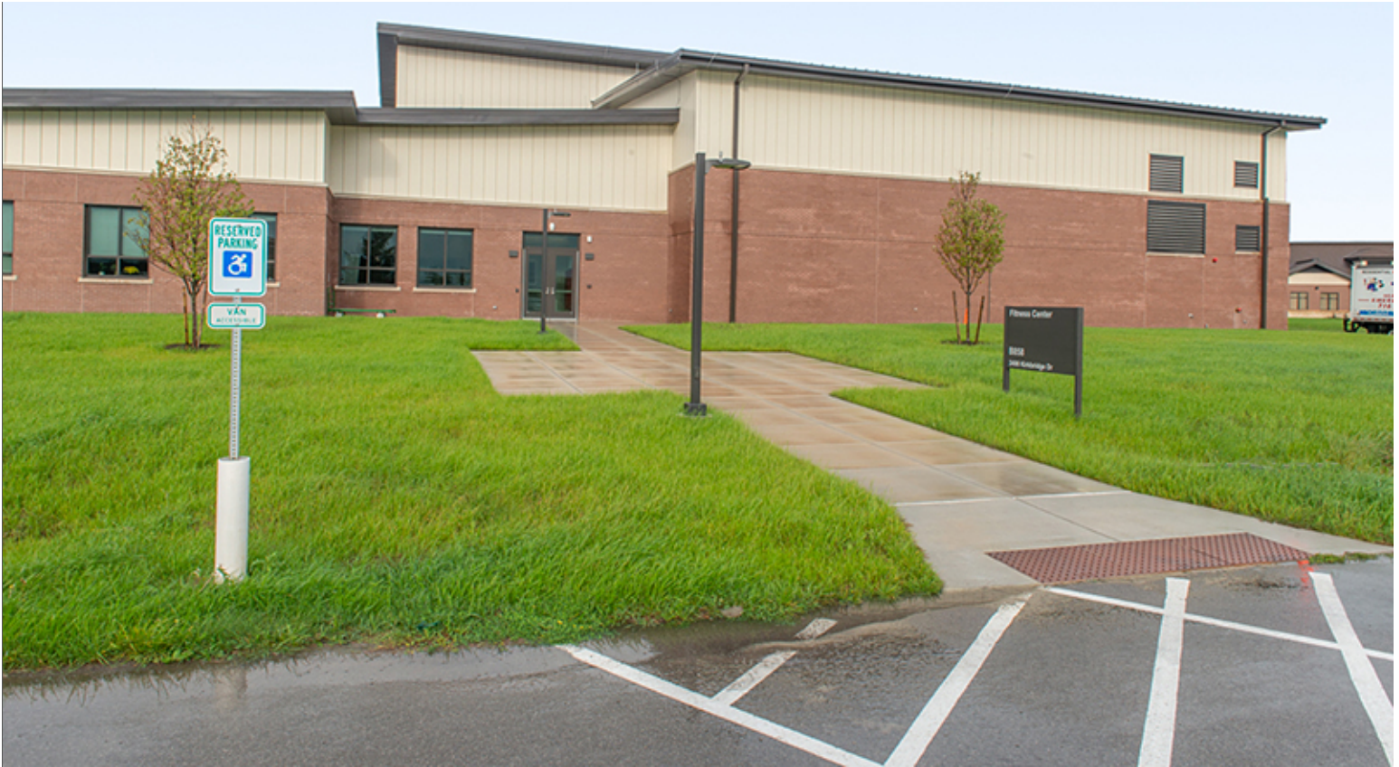
Standard Asphalt Paving with White Striping
