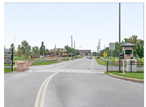
Entrance Avenue Security Elements
