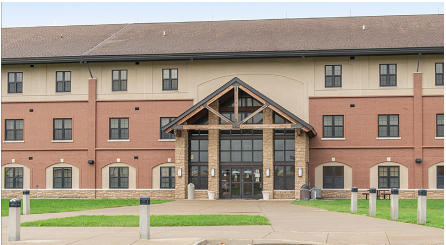
Concrete Paving at Group 2
