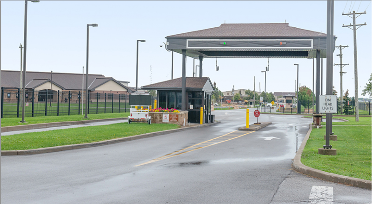
Primary Access to Niagara Falls ARS Via Entrance Avenue
