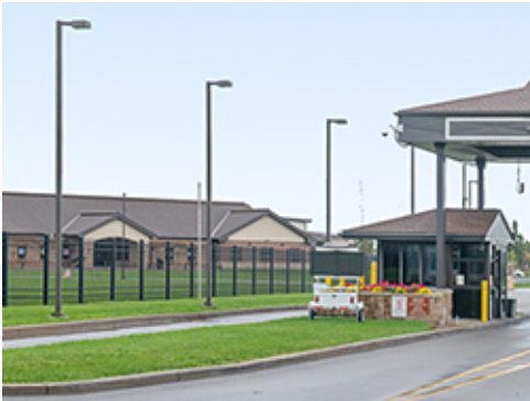
Uniform Street Lighting at Group 1
