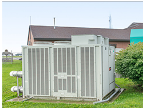
Vegetative Screening at Utility Element
