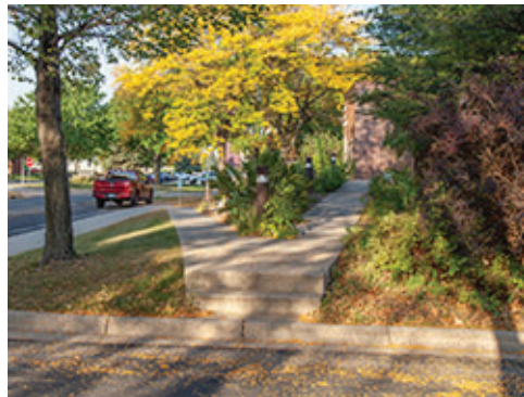
Steps at Ramp Switchback
