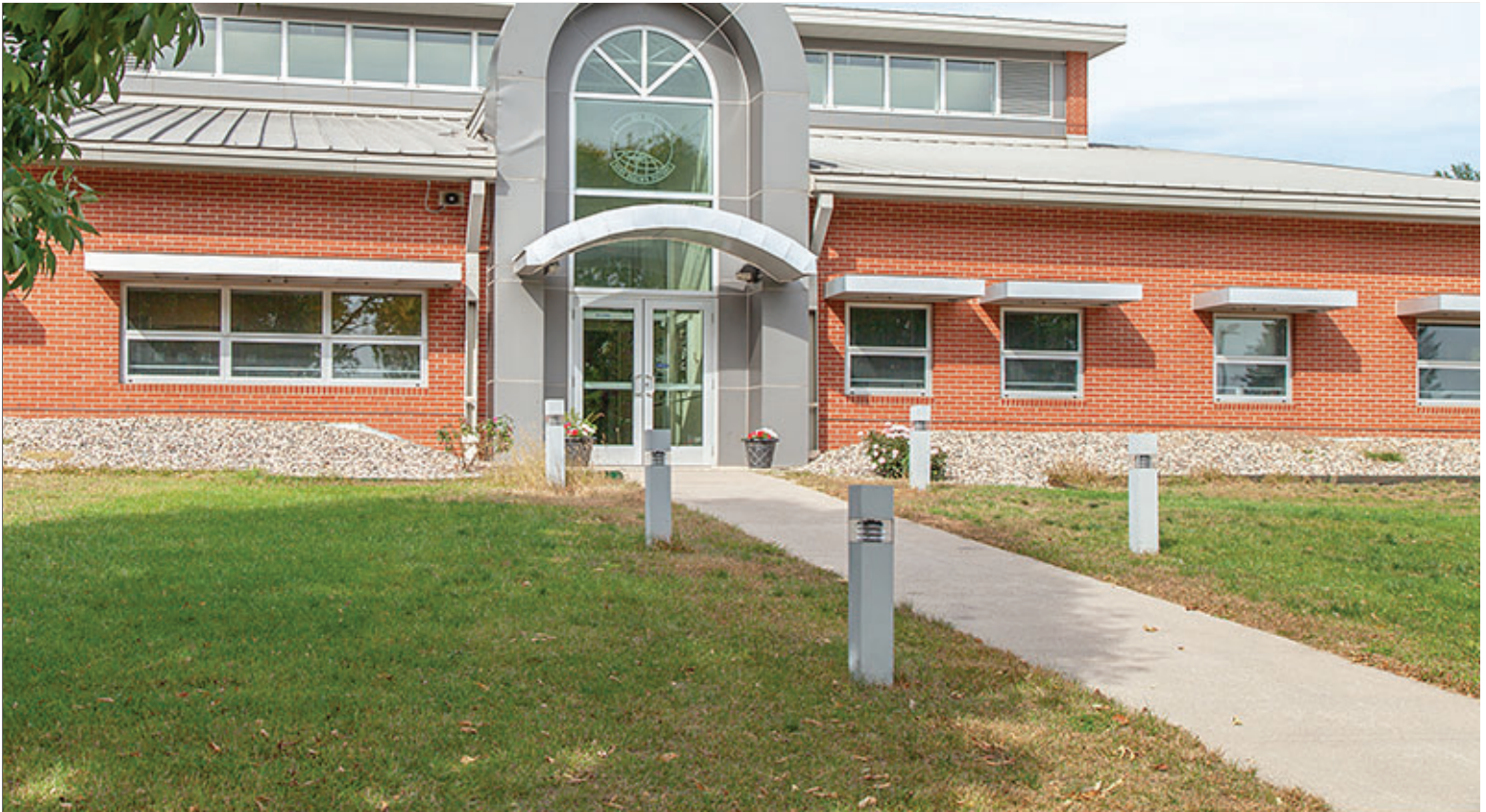
Concrete Sidewalk at Group 1 Main Entrance
