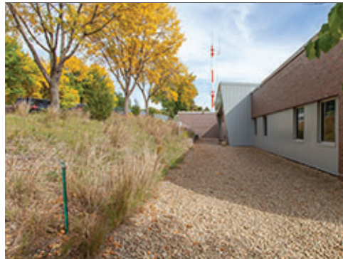
Planting to Stabilize Slope
