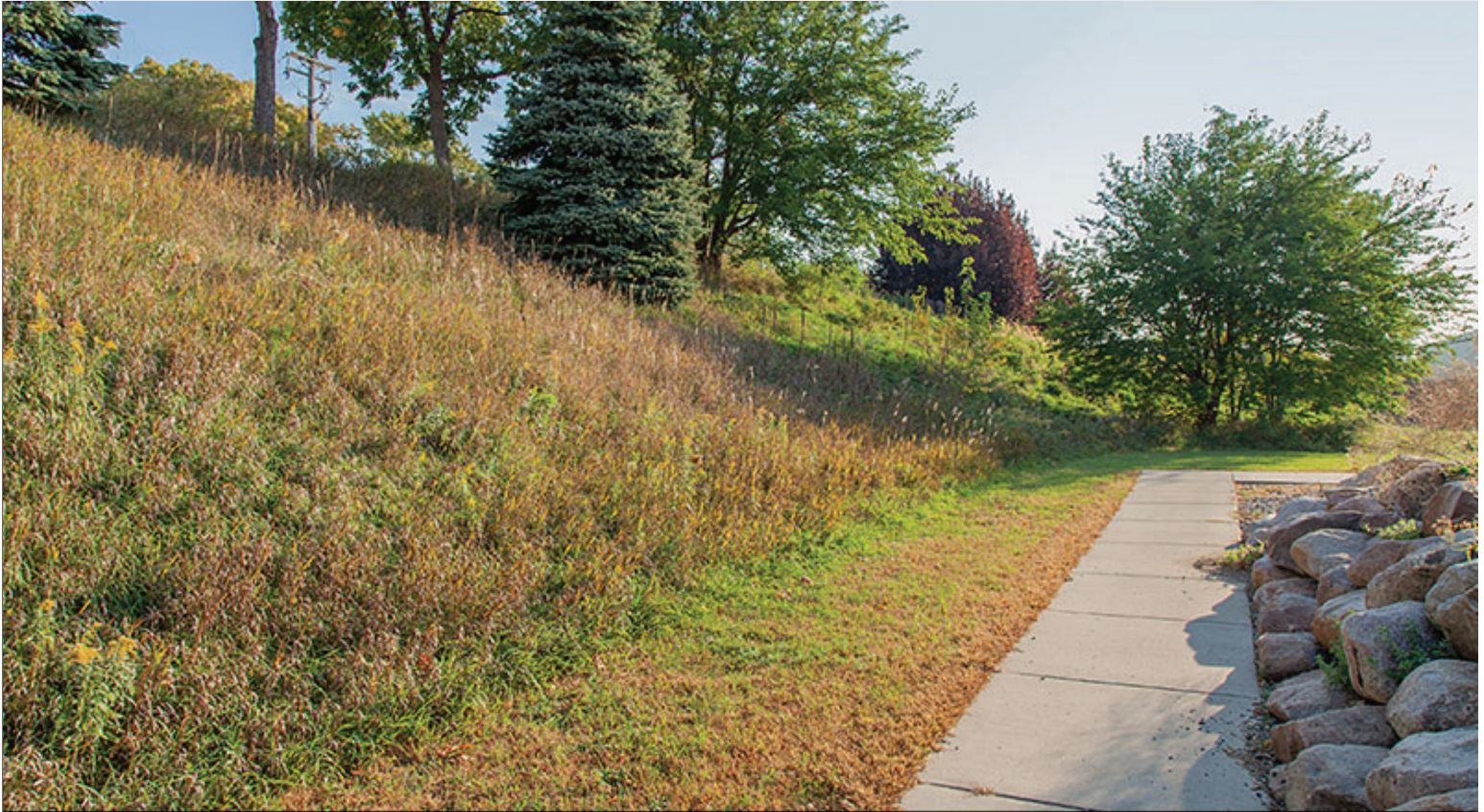
Slope Stabilization with Vegetation and Boulders
