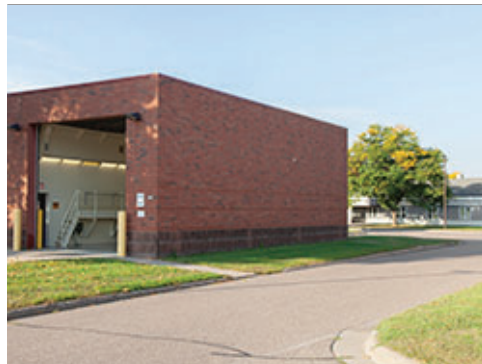
Paving without Markings
