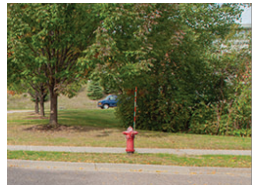
Hydrant with Marker for Snow Removal
