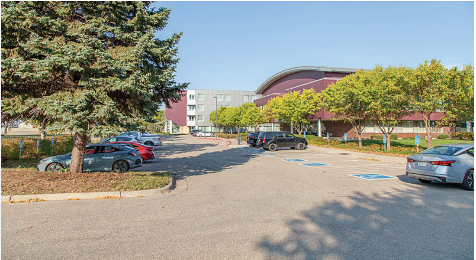
Asphaltic Concrete Paving with Standard White Striping and Accessible Parking Symbols
