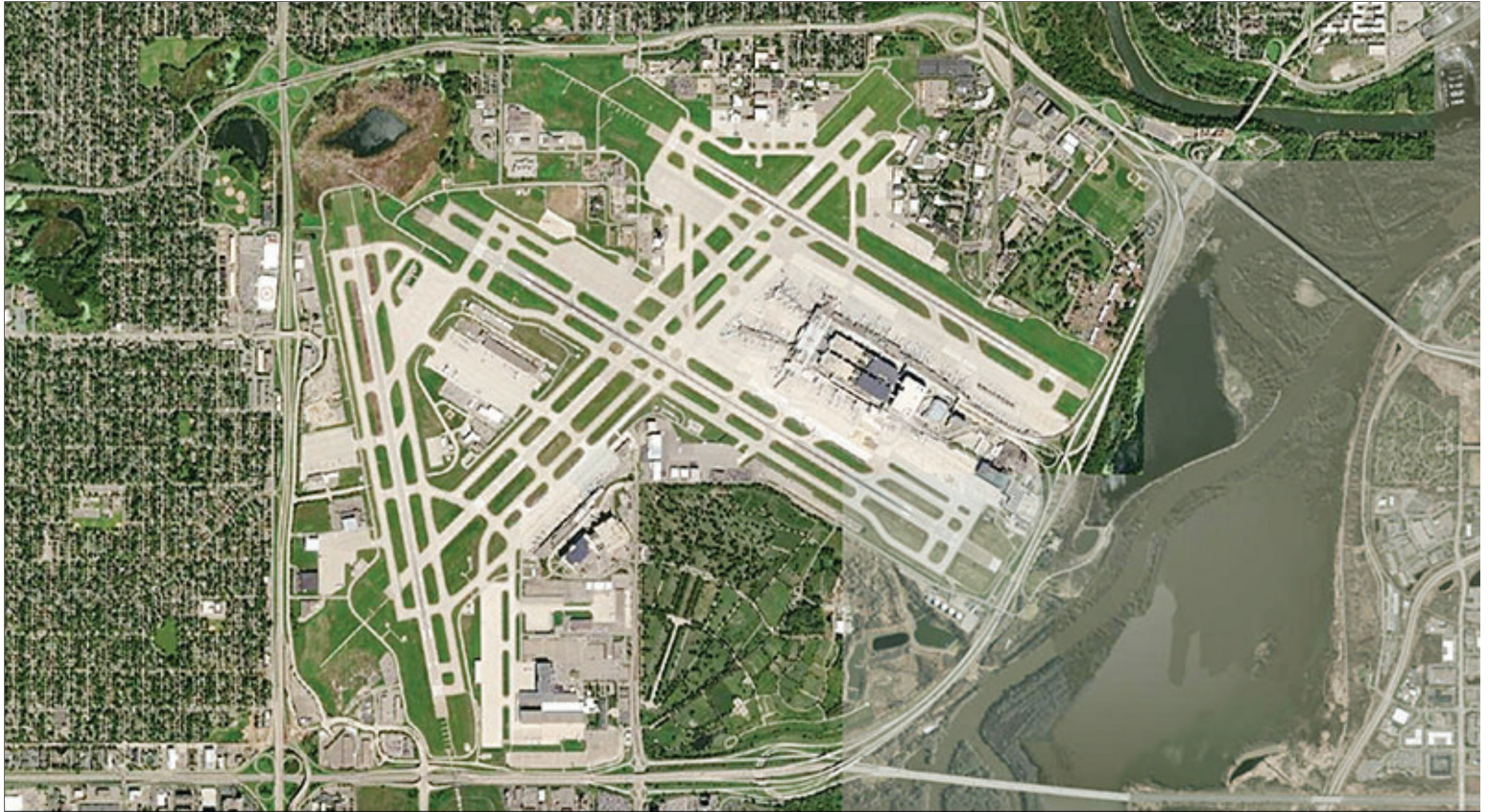
Minneapolis-Saint Paul Air Reserve Station along the Northern Boundary of Minneapolis-Saint Paul International Airport
