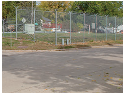
Fence along Perimeter Road
