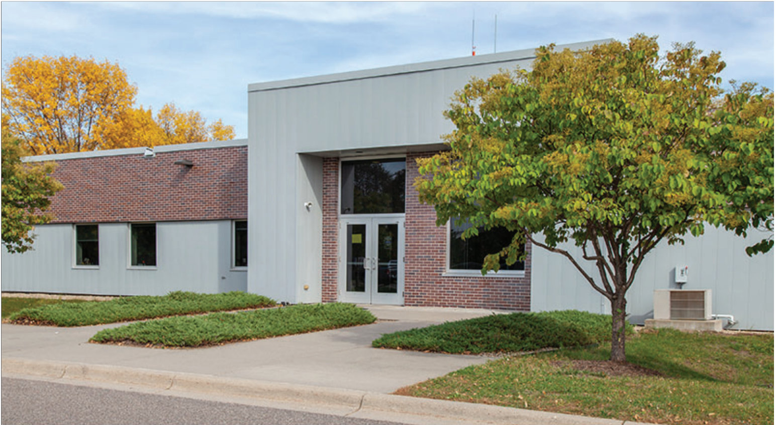
Contemporary Vernacular Theme with "Minn-St Paul" Blend Brick and Flat Metal Panels
