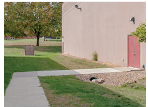
Stormwater Element at Sidewalk
