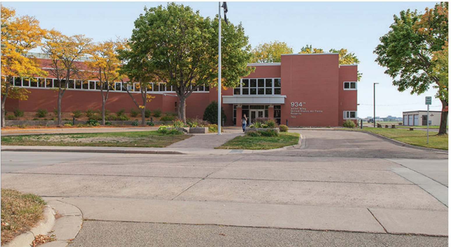
Intersection at Group 1
