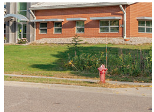
Fire Hydrant with Marker
