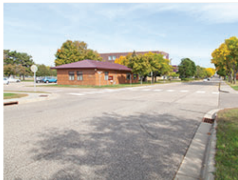
Stormwater Inlet at Curb and Gutter
