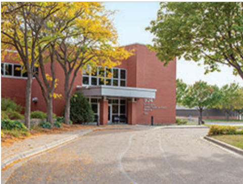
Red Brick at Group 1
