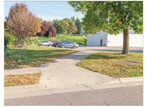
Curb Ramp at Group 3
