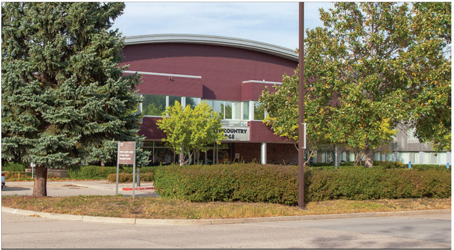
Predominant Use of Ribbed Metal Sheeting with Form and Massing Used to Define Main Entrance
