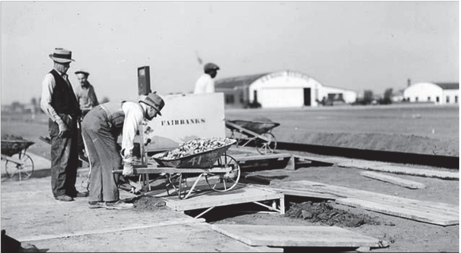
Wold-Chamberlain Field's First Paved Runways Being Laid by the WPA, Circa 1937
