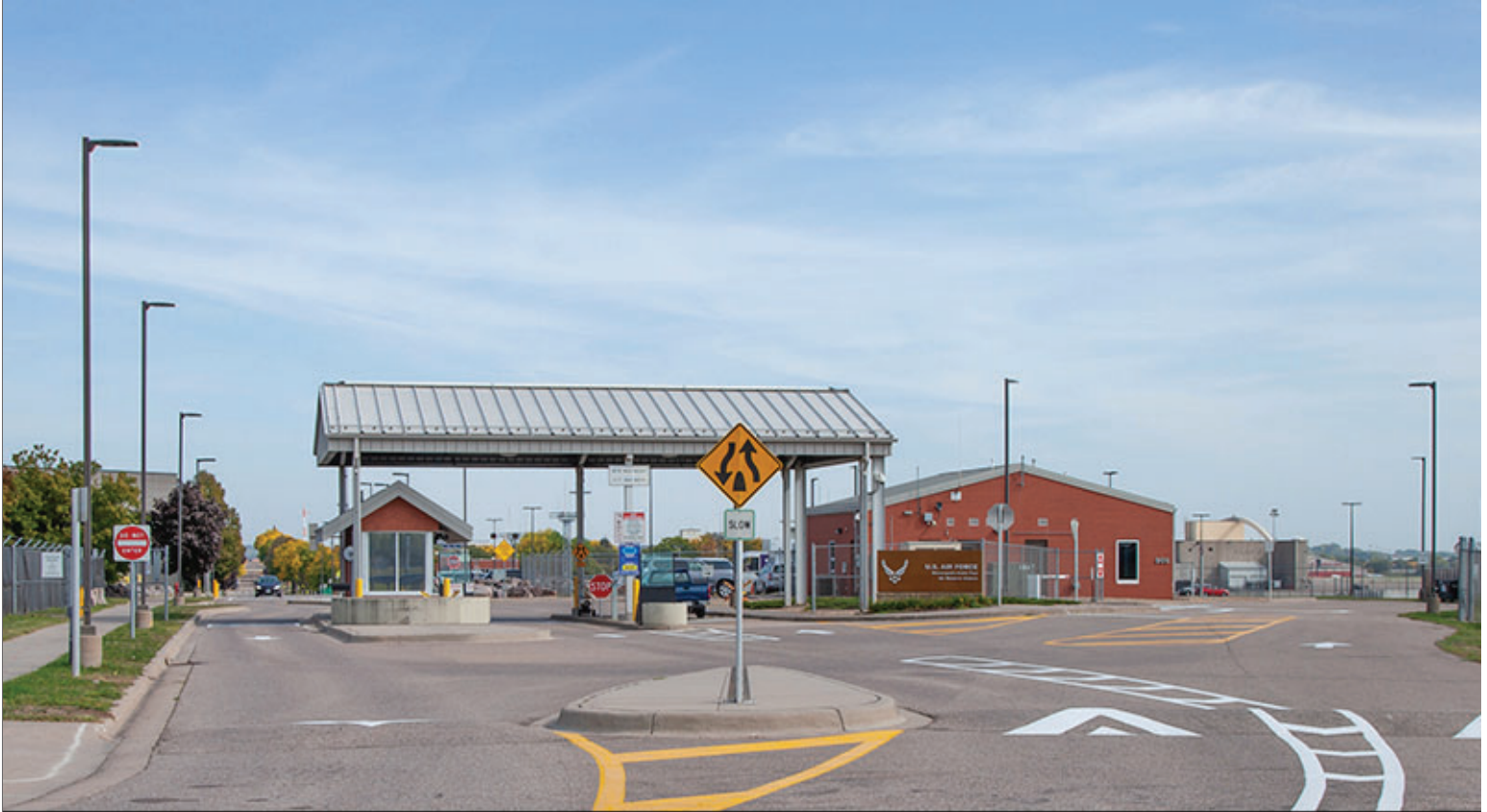
Main Gate at South 34th Avenue and Military Highway
