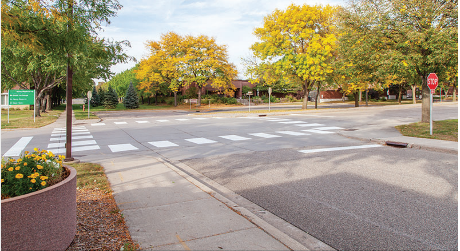
Intersection at Military Highway and Kittyhawk Avenue
