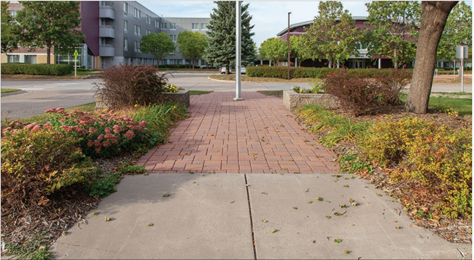
Unit Pavers at Installation Flagpole
