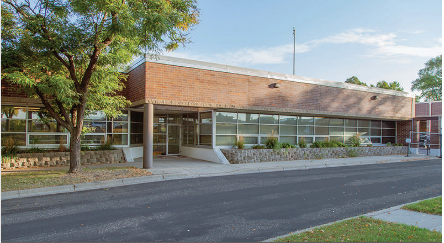
South Facing Facade with Appropriate Overhang for Shading
