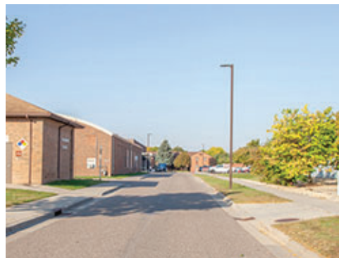
Buried Utility Lines
