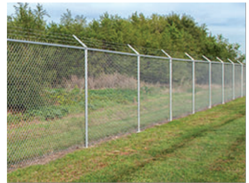
Chain Link Perimeter Fence
