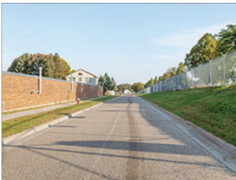
Detached Sidewalk on One Side
