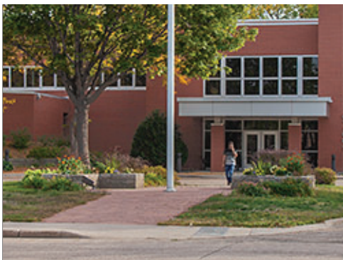
Colored Concrete Paving at Group 1
