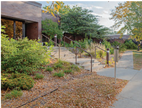
Stair with Adjacent Ramp
