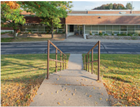
Connection to Main Entrance
