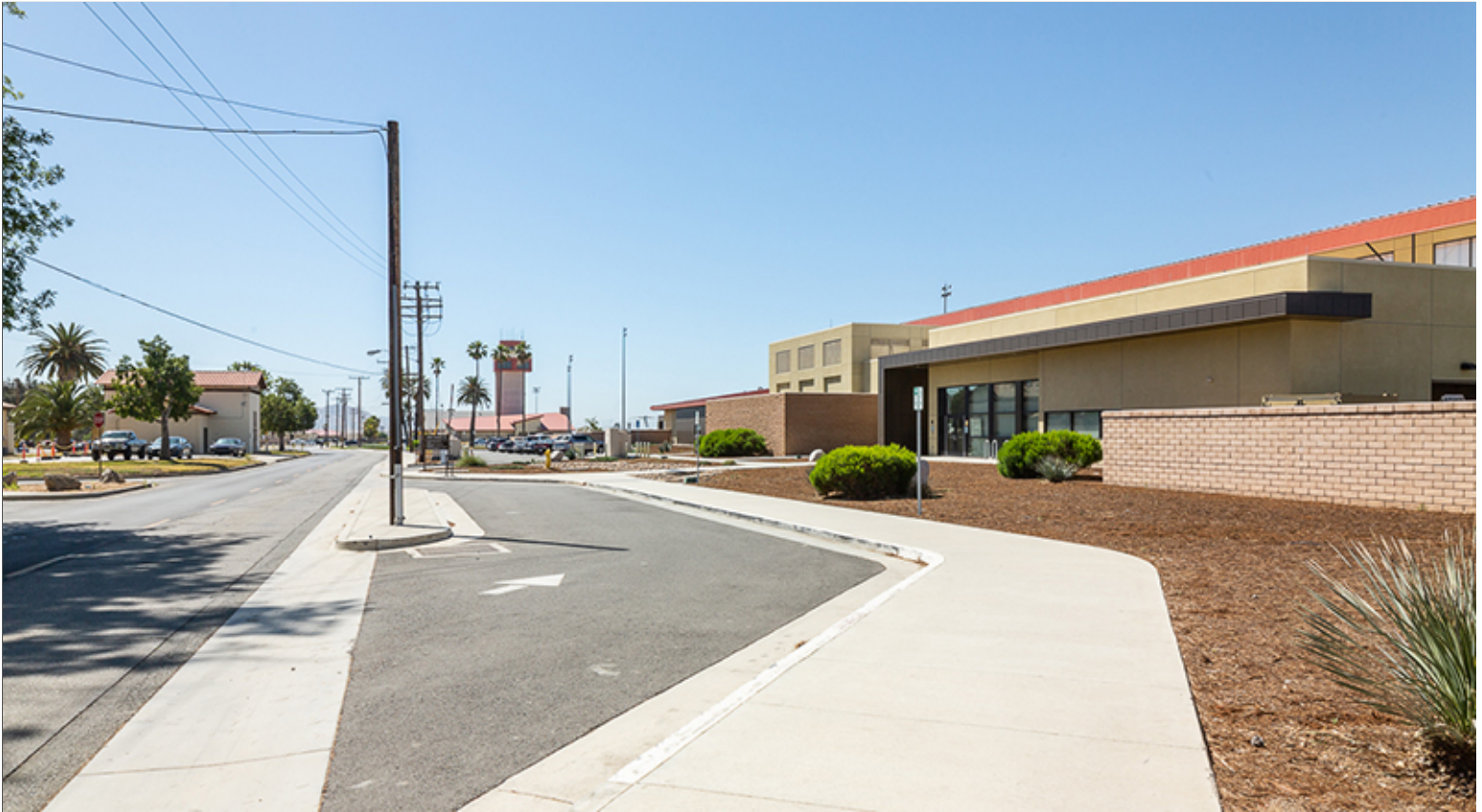
Natural Concrete Sidewalk along Drop-Off Lane
