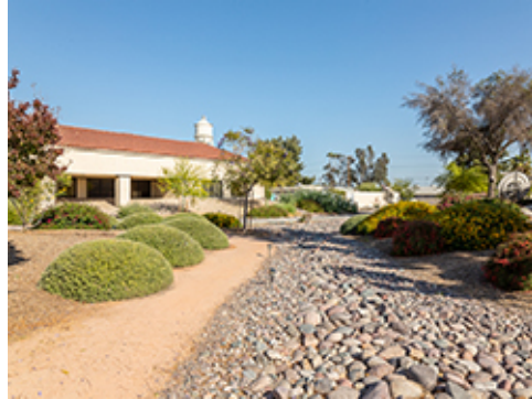
Drainage path with River Rock Mulch
