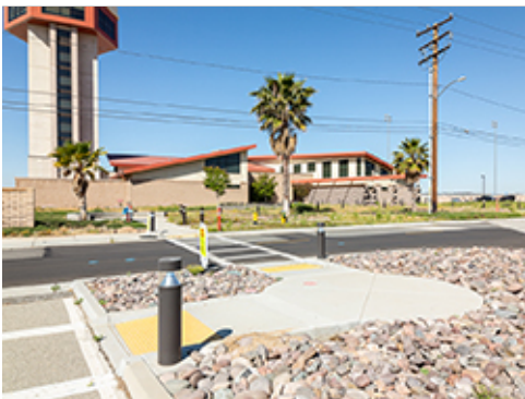
Link to Parking Area
