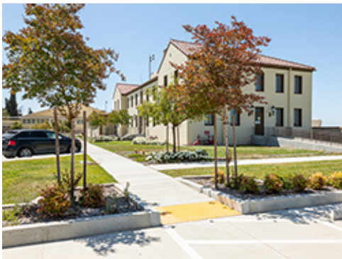
Sidewalk with Curb Ramp at Parking Area
