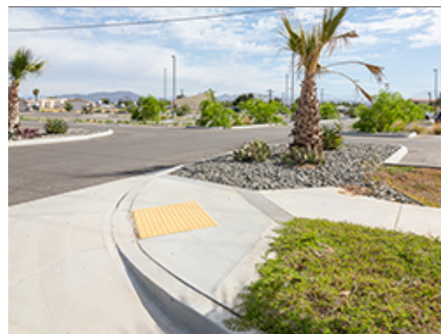
Accessible Curb Ramp
