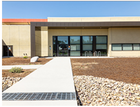
Flush Mounted Grate for Drainage
