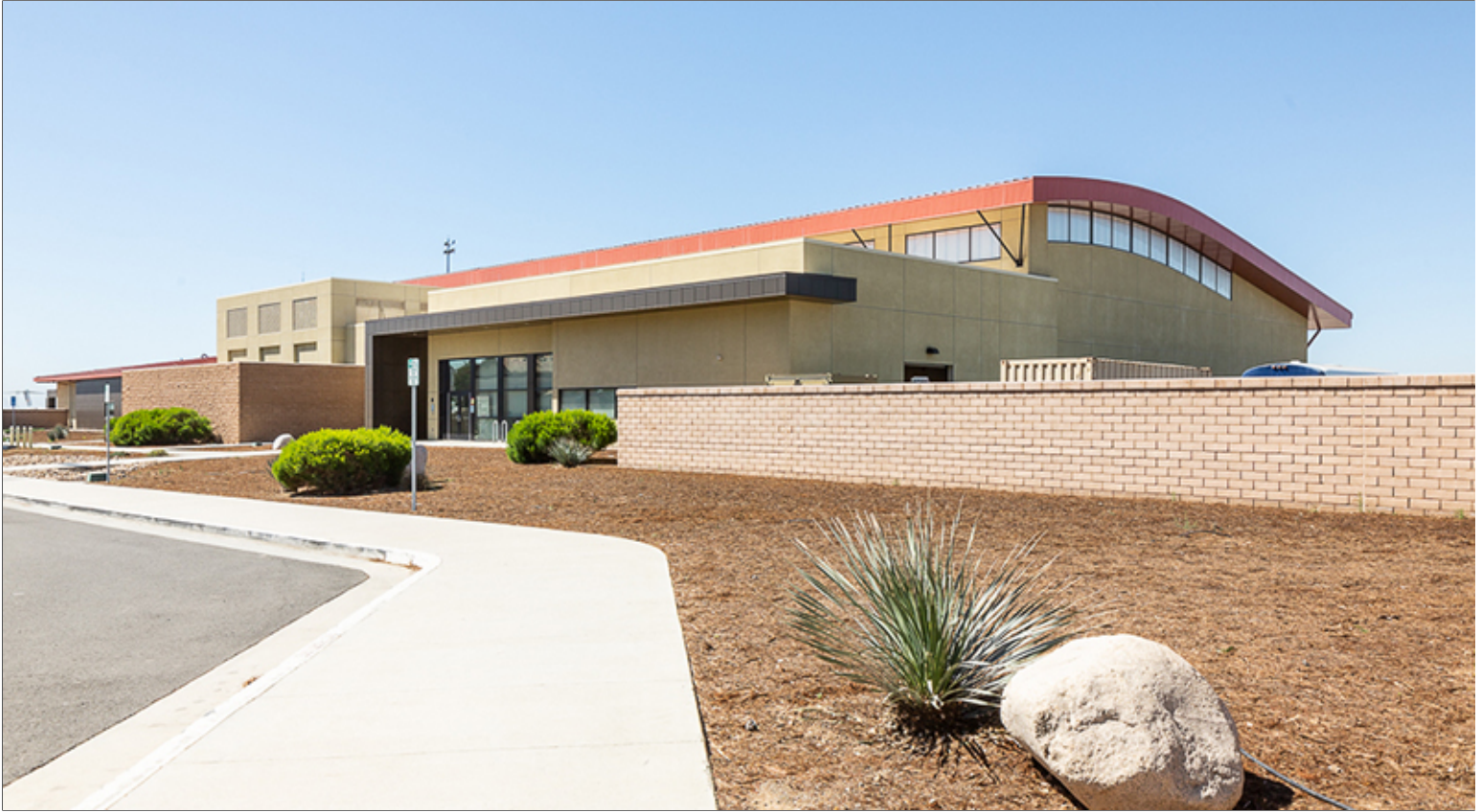
Functional Shading at Entrance and Windows
