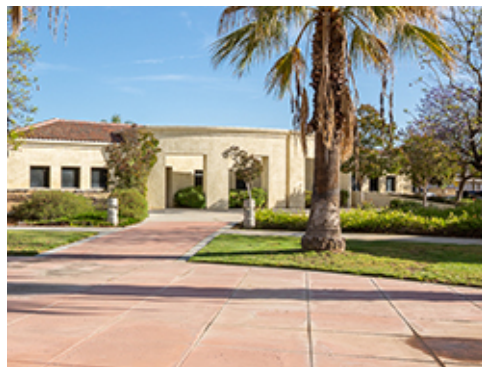
Colored Concrete Plaza
