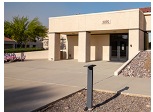
Concrete Entrance Plaza
