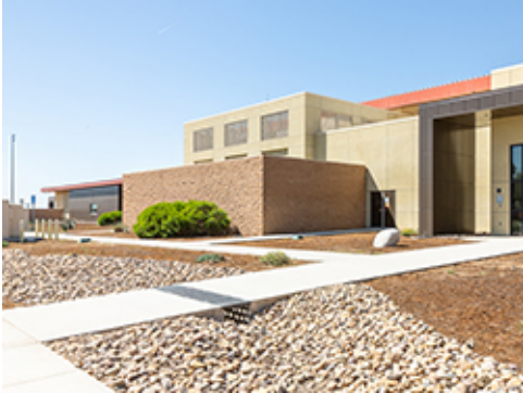
Grate at Sidewalk
