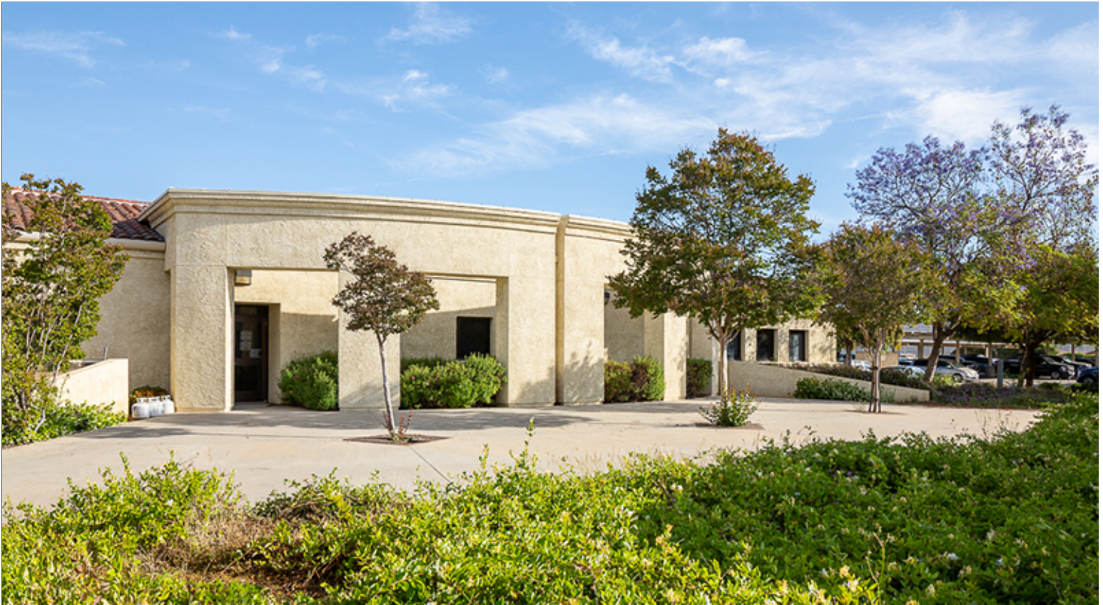
Natural Concrete Paving at Group 2 Plaza
