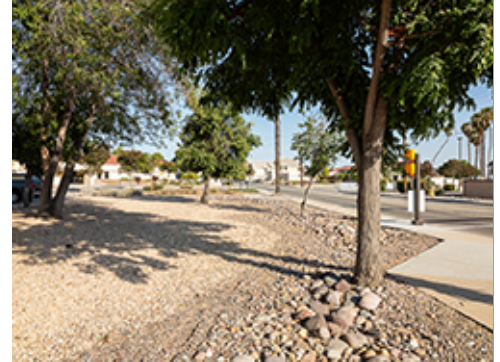
Drainage Swale with Tree Planting
