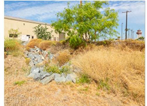
Erosion Control Measures
