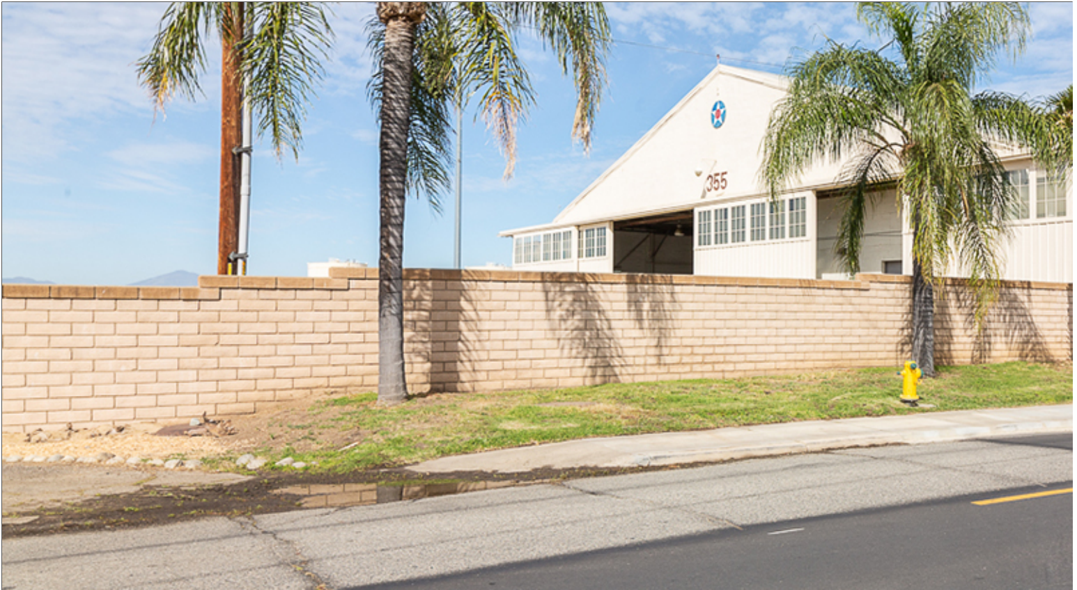
Masonry Screen Wall at Group 3
