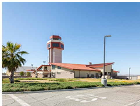
Parking Lot Fixture
