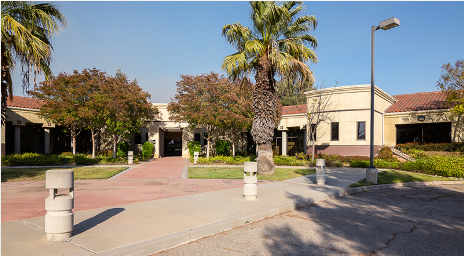
Colored Concrete Paving at Group 2
