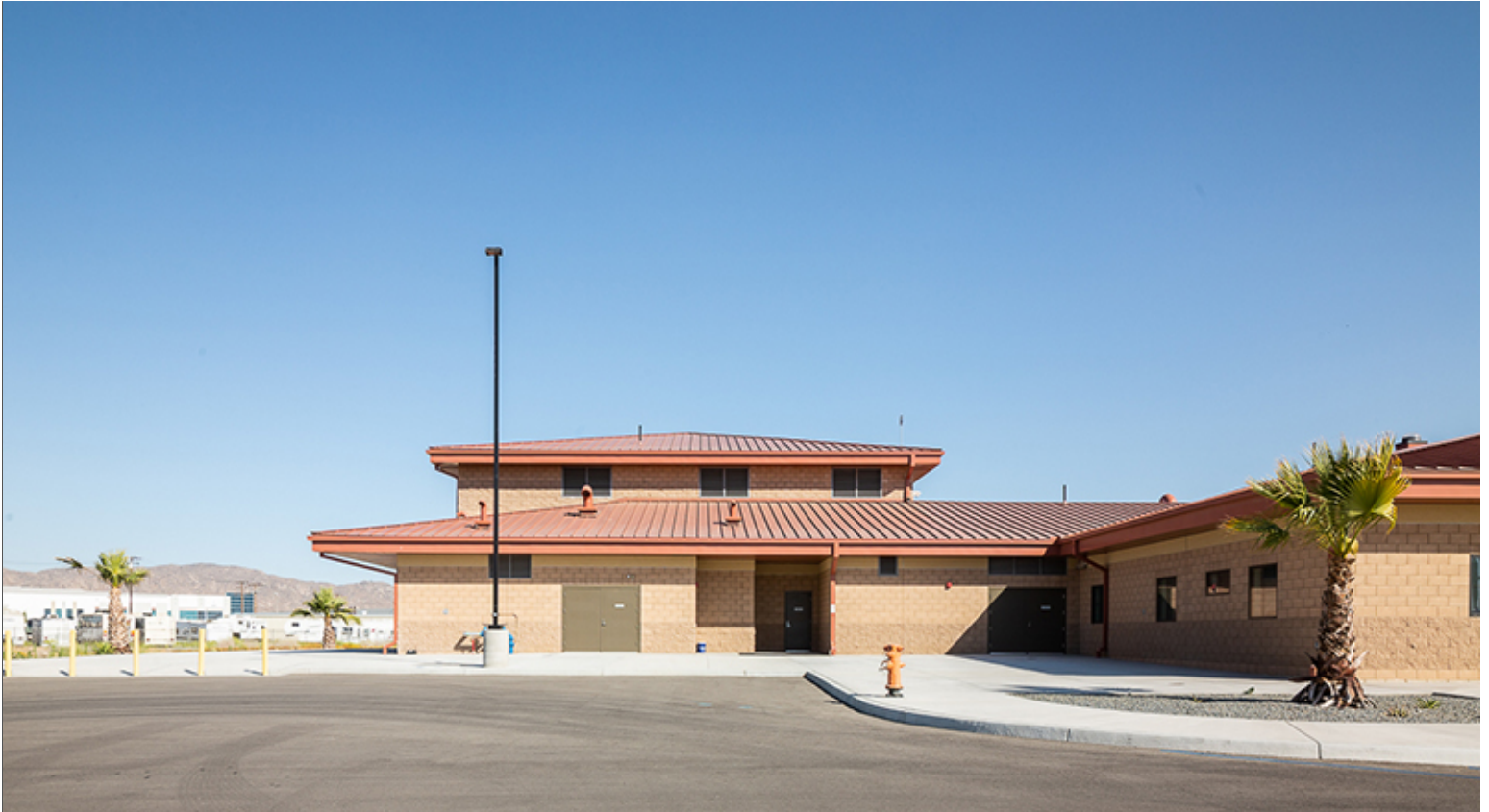
Group 3 with Tall Concrete Base for Durability
