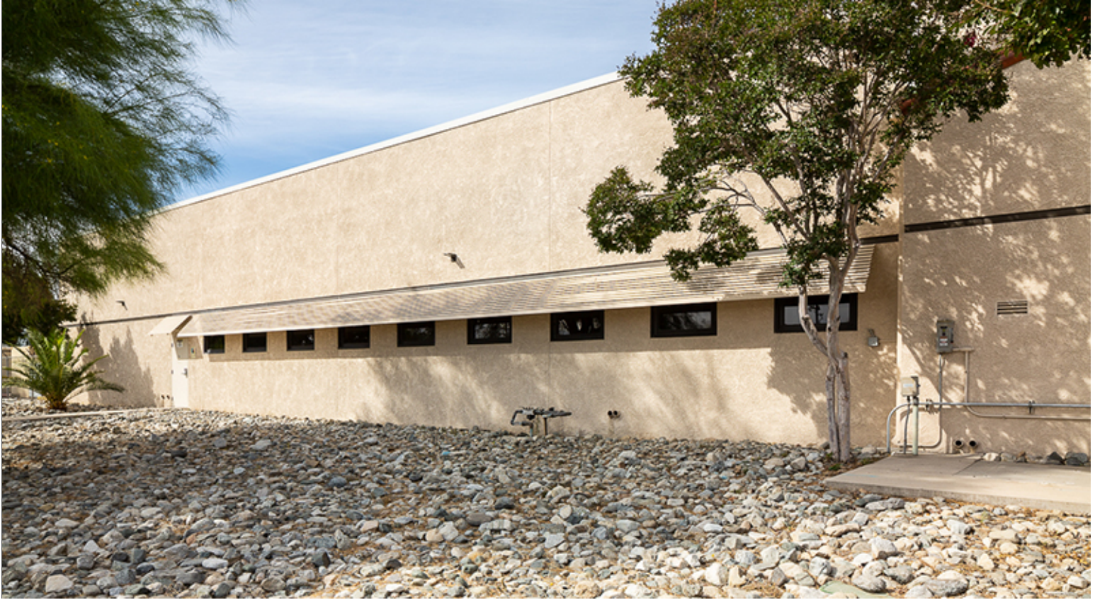
Stucco Wall Systems and Shading Device in Earth-tone Colors
