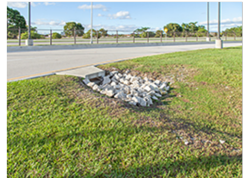
Rip Rap for Erosion Control
