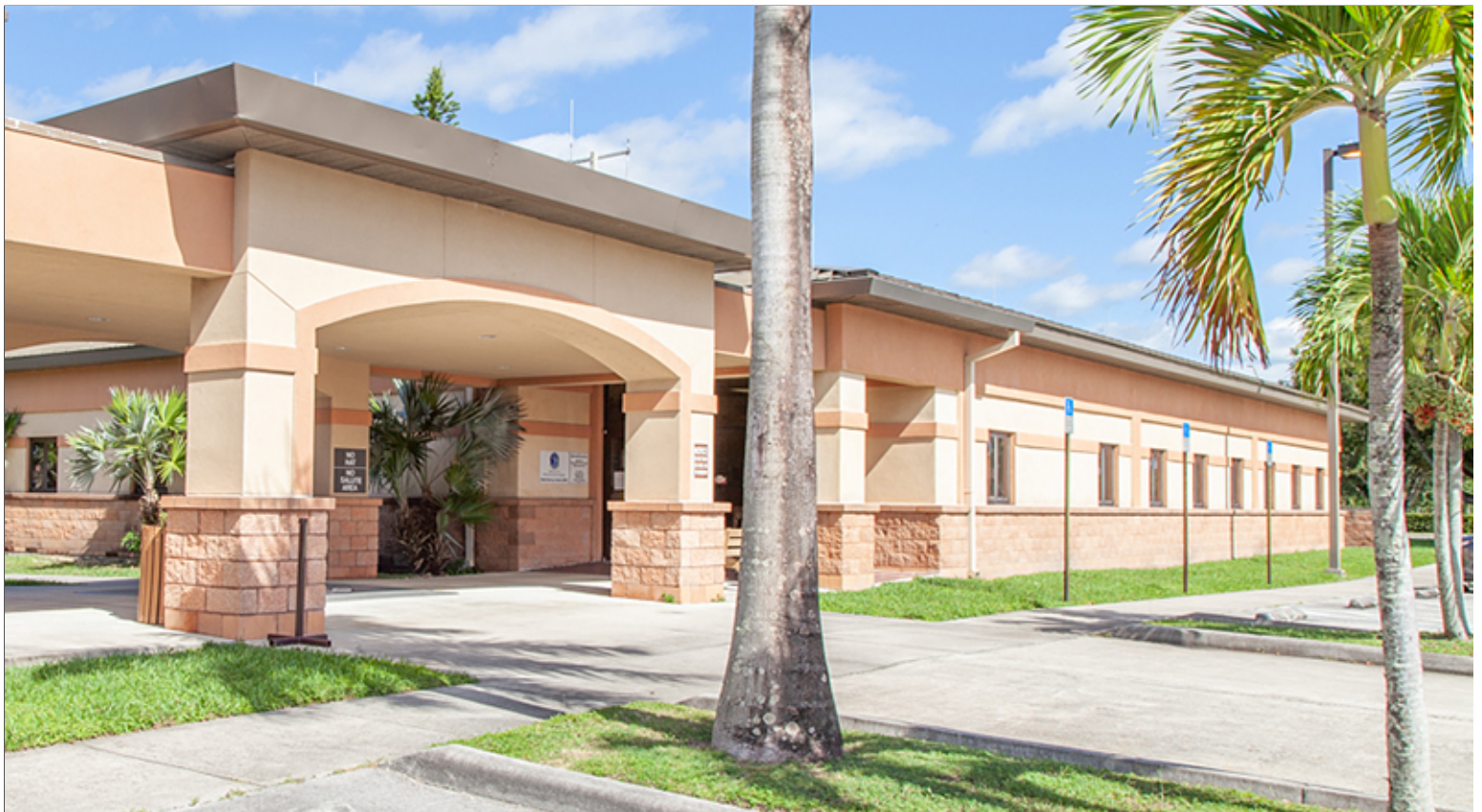
Concrete Masonry Unit (CMU) Wainscot and Water Table and Stucco with Main Color and Accent Color
