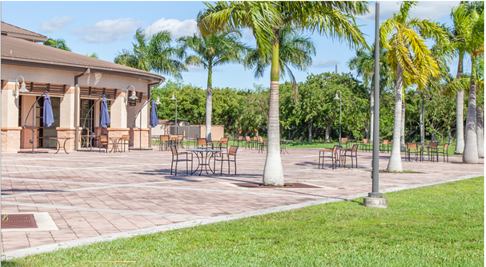
Plaza at Group 2 Lodging with Integrally Colored Unit Pavers and Concrete Edging
