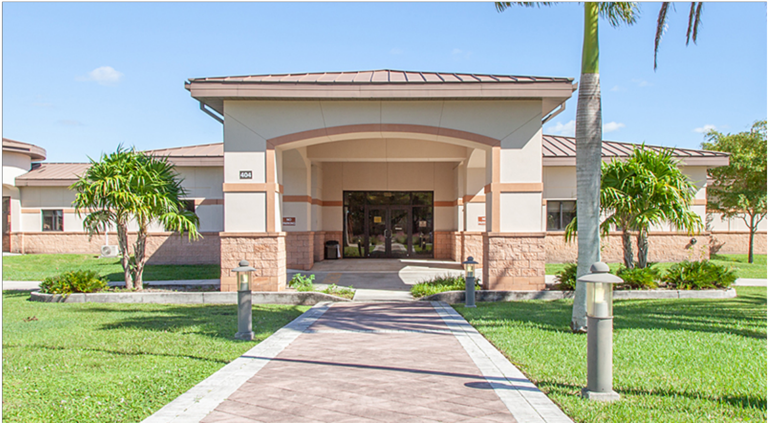
Entrance Plaza at Group 2 with Porte Cochere
