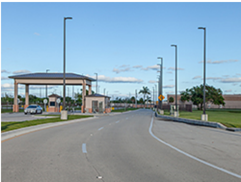
Typical Street Lighting Fixtures
