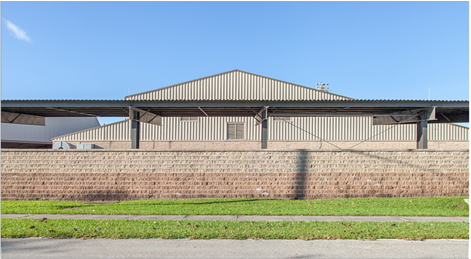
Group 3 Facility with Compatible Masonry Screen Wall
