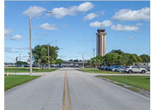
Ploesti Road Approach to Tower
