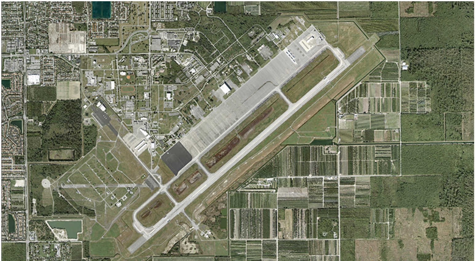
Aerial Photograph of Homestead Air Reserve Base and Adjacent Community
