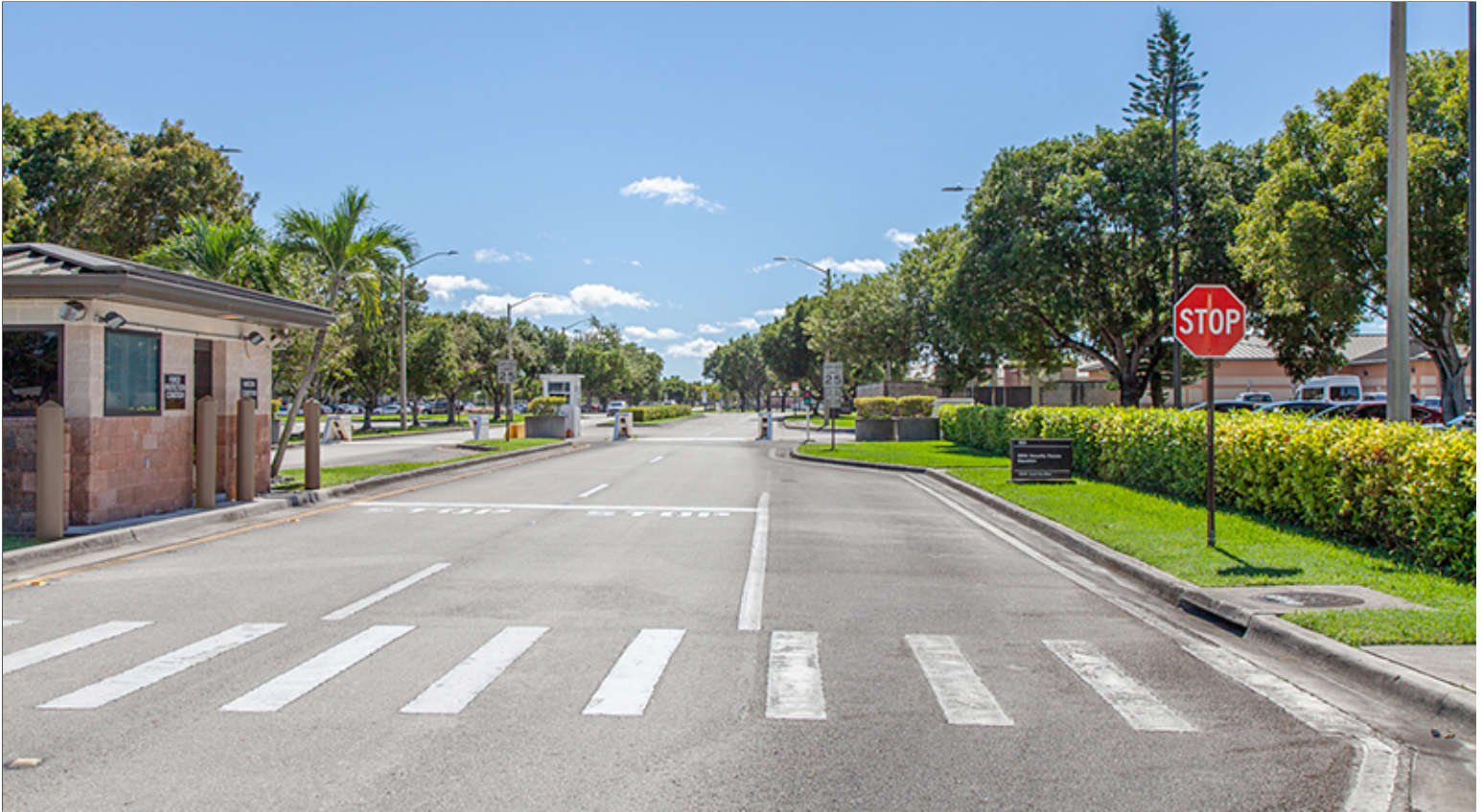
Original Main Gate with Preserved Divided Lanes and Street Elements
