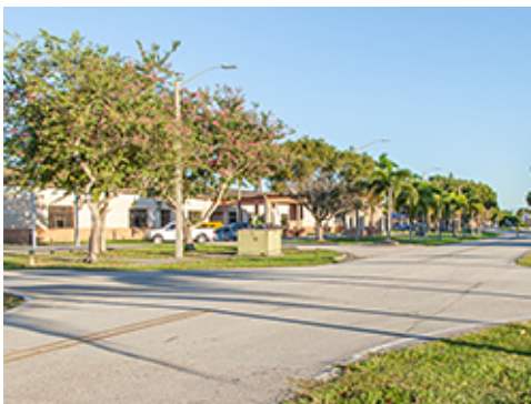
Buried Service Lines and Utility Cabinet
