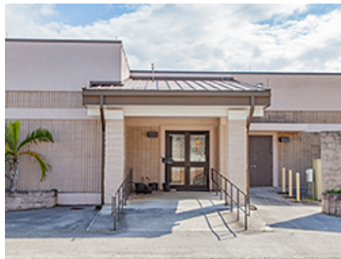
Ramp at Entrance in Group 3
