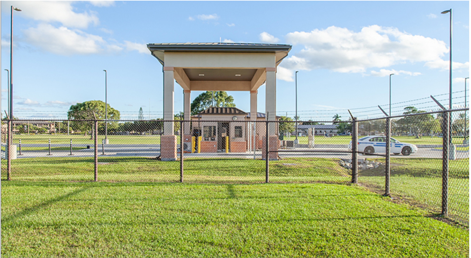
Chain Link Fencing at Main Gate
