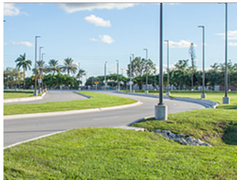
Grass Median at Approach to Biscayne Drive
