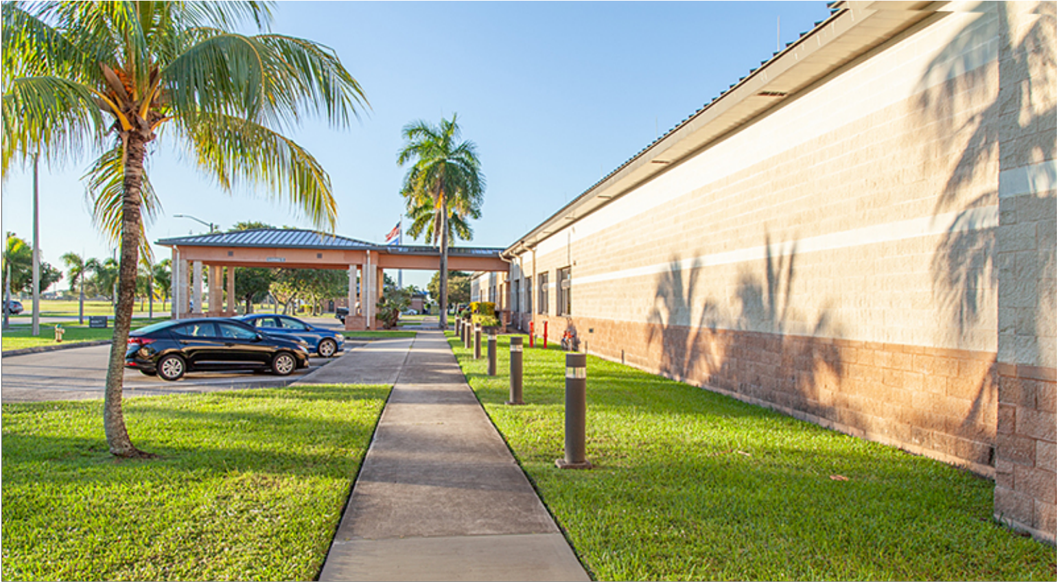
Lighted Bollards Defining Walkway at Group 1
