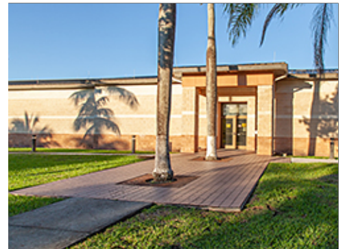
Tile Paving at Group 1
