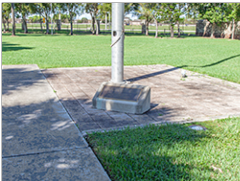
Bronze Plaque on Concrete Base
