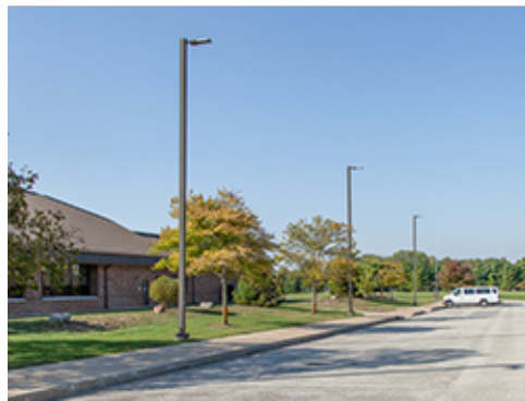
Single Fixture at Parking Lot Perimeter
