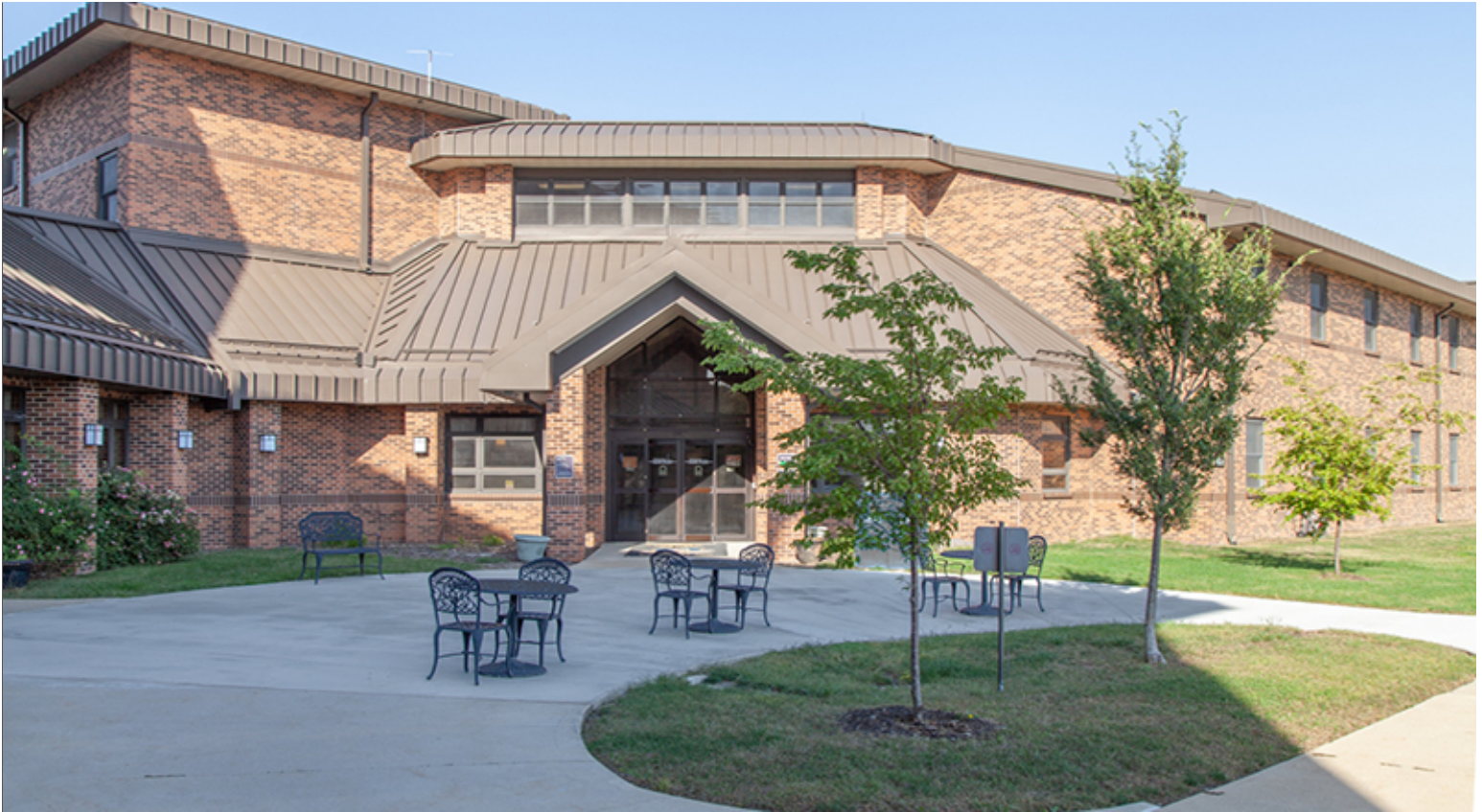
Concrete Paving at Group 2 Lodging Plaza
