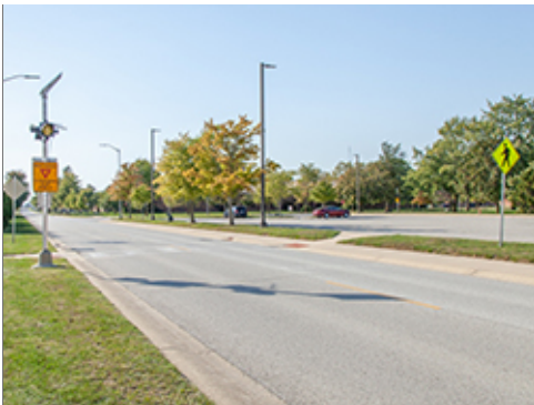
Crosswalk with Flashing Signal
