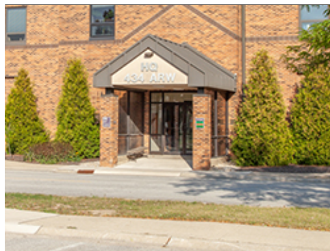
Covered Entrance with Concrete Paving
