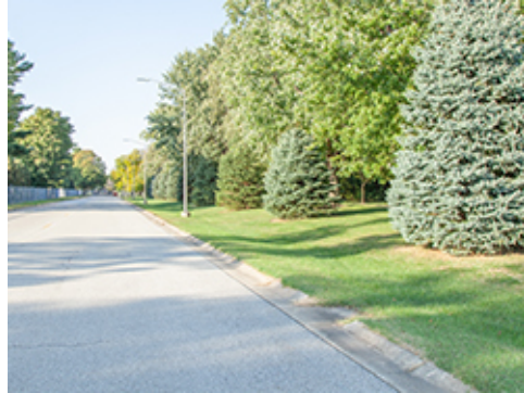
Drainage Swale along Street
