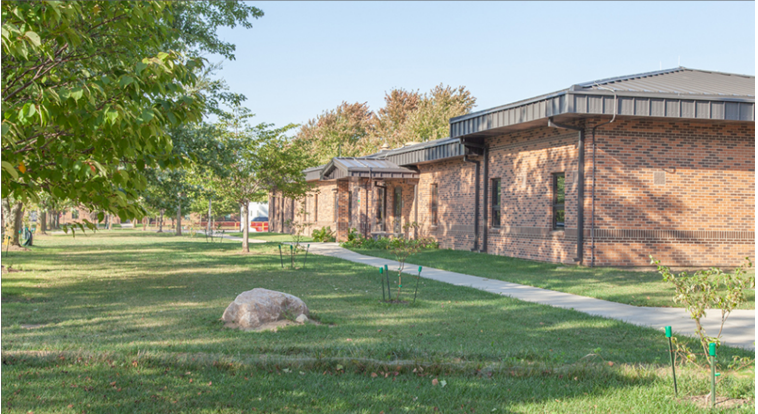
Site Grading and Roof Drainage Directed to Grass Area
