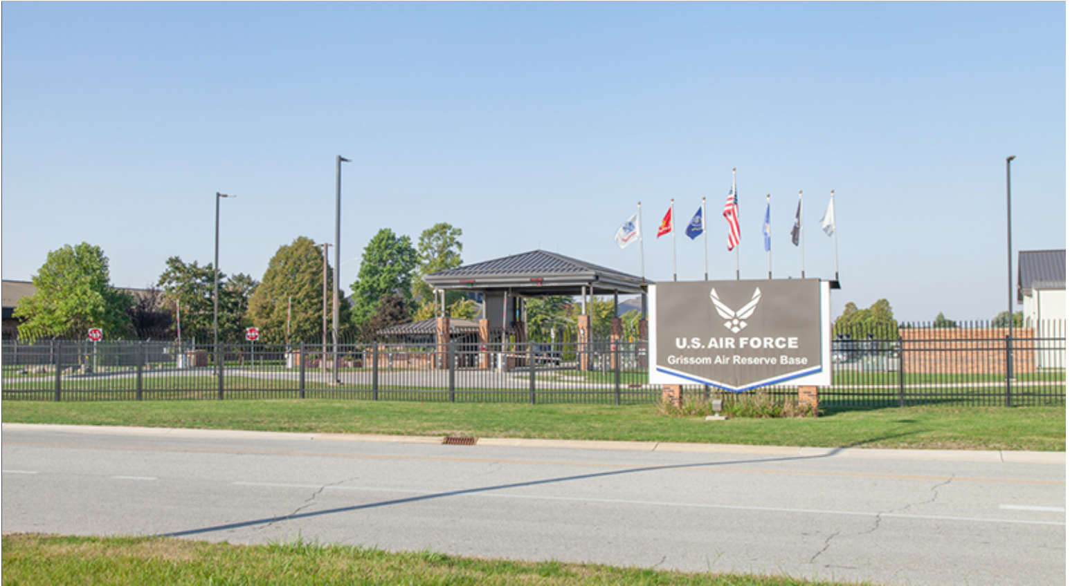
Group 1 Main Gate at North Hoosier Boulevard
