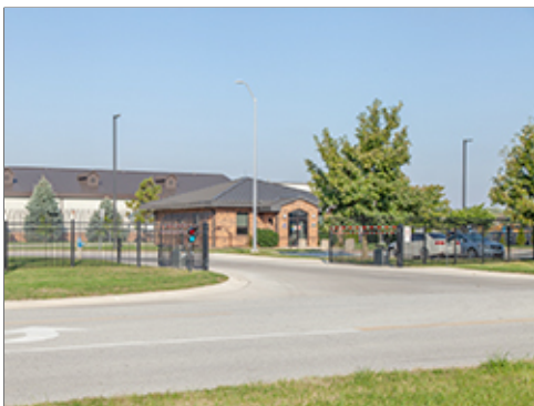
Security Fencing and Elements
