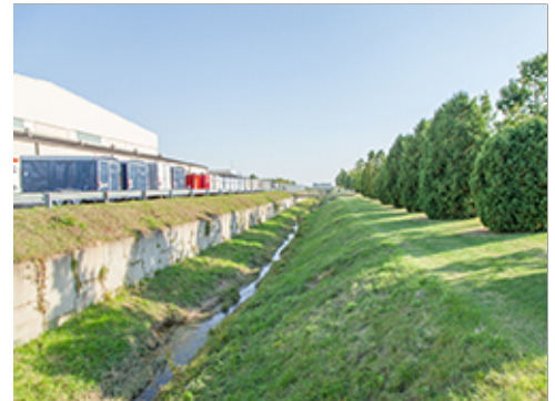
Channel with Engineered Retaining Wall
