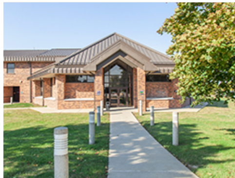
Lighted Bollards along Sidewalk
