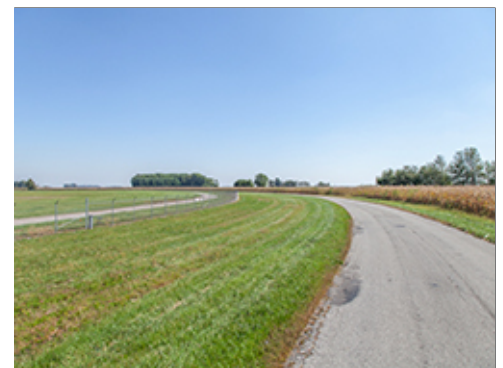
Road along Perimeter Fence
