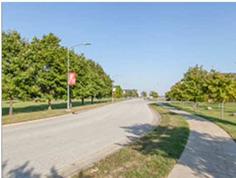
Collector with Detached Sidewalk
