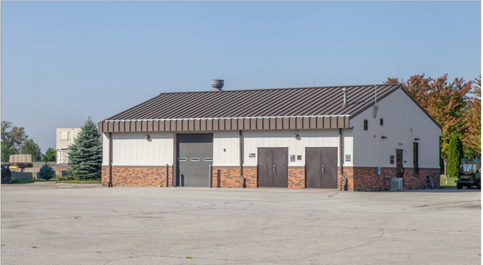
Underground Utility Service Lines at Group 3
