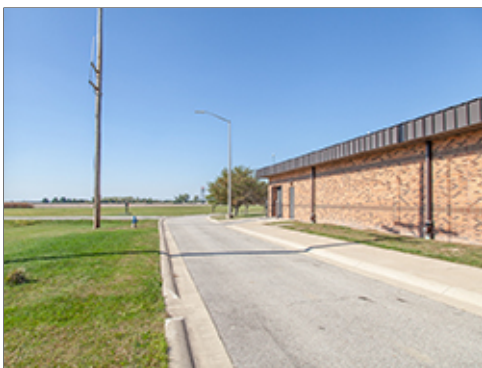
Local Street with Attached Sidewalk
