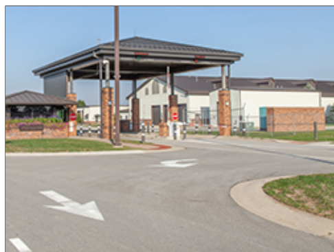
Standard Street Markings
