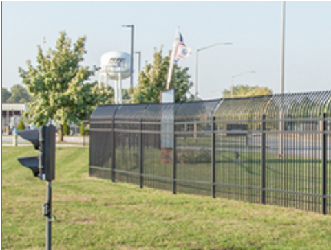
Metal Fence at Group 1
