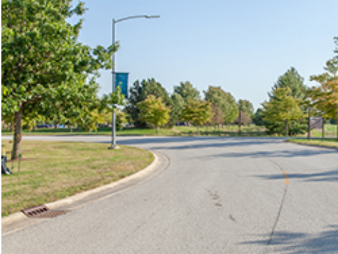
Drainage Inlet at Curb
