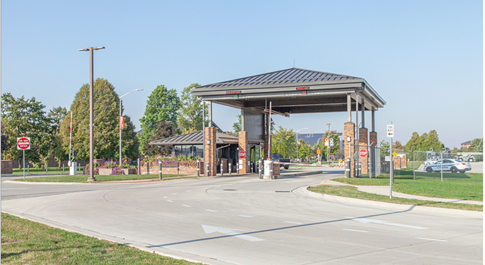
Main Gate at North Hoosier Boulevard
