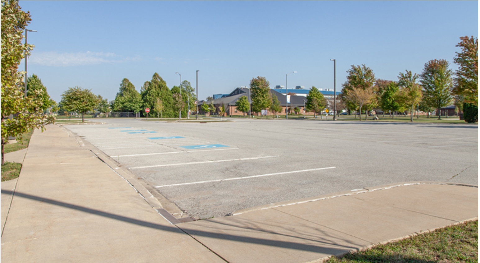
Standard Bituminous Paving and White Striping
