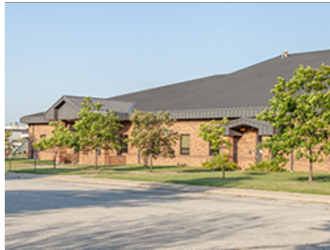
Consistent Entrance Features
