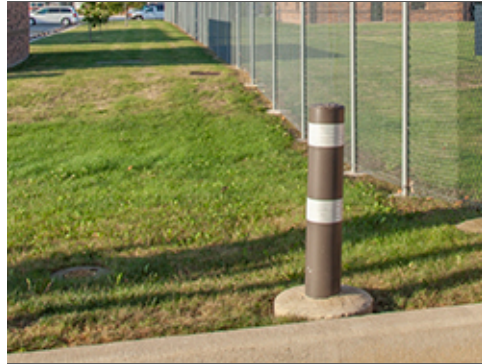
Steel Pipe Bollard
