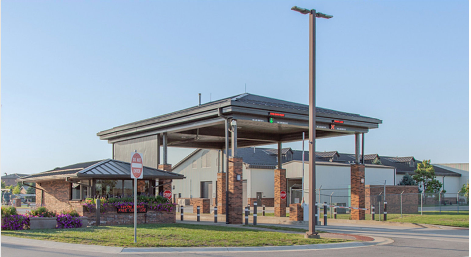
Dual Fixture at Main Gate
