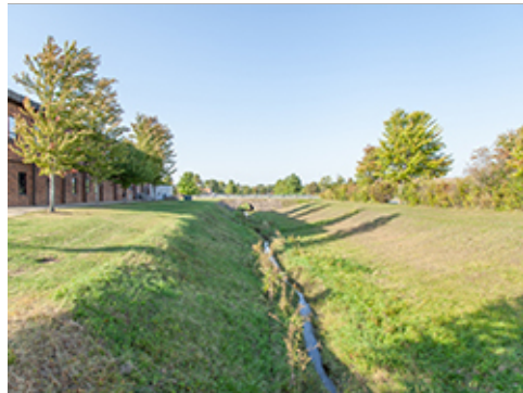
Vegetated Drainage Channel
