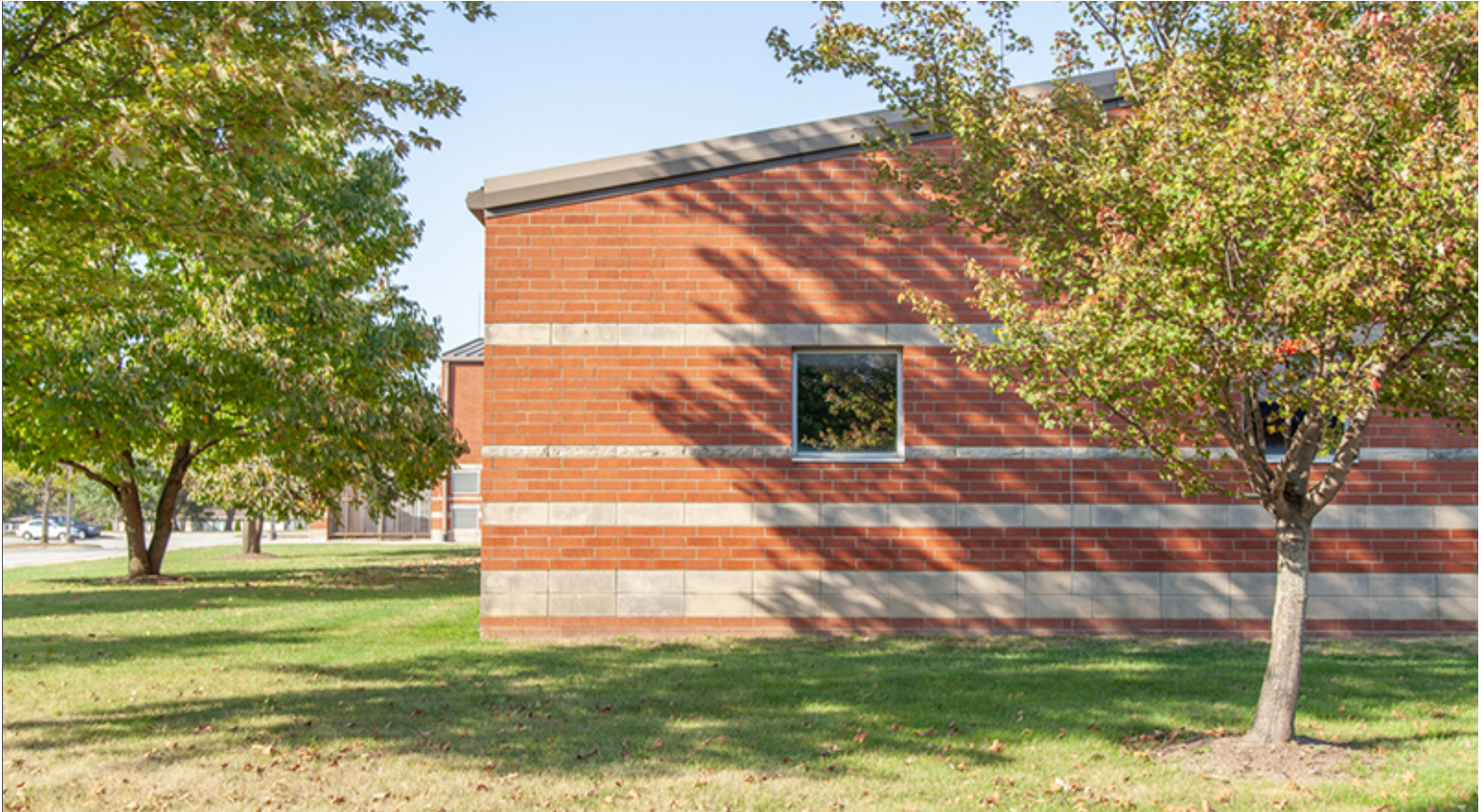
Deciduous Trees for Shading in Summer and to Promote Solar Heat Gain in Winter
