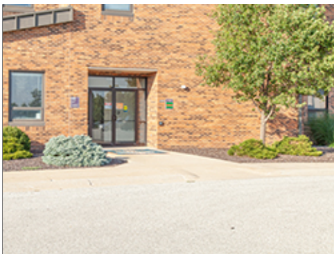
Concrete Entrance Plaza
