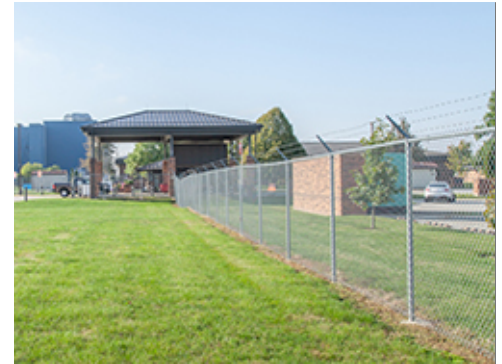
Security Fence along Group 3 Site
