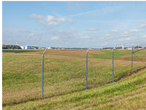
Fencing along Airfield
