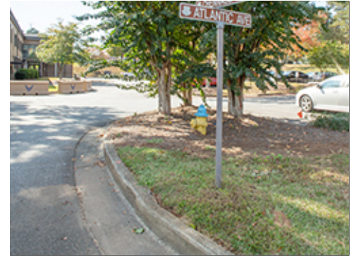
Fire Hydrant near Intersection
