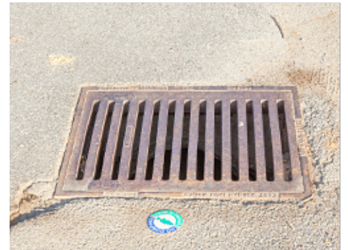
Grate with Adjacent Medallion
