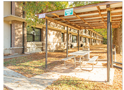
Covered Picnic Area at Group 2 Lodging
