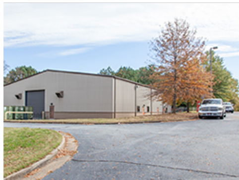
Grass Planting at Corner
