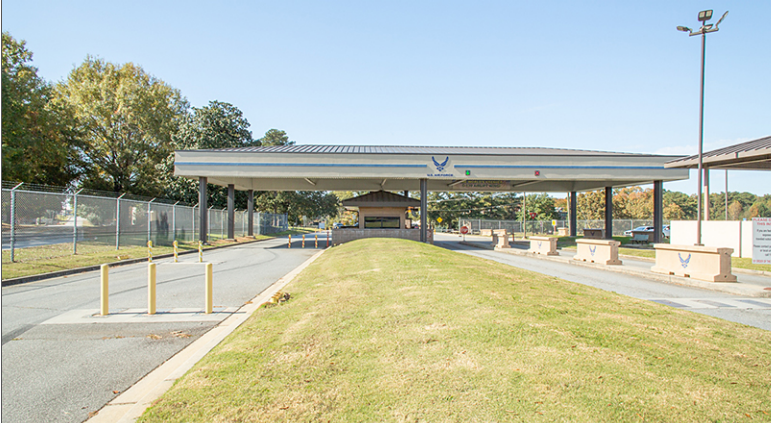
Approach to Main Gate at Atlantic Avenue SE
