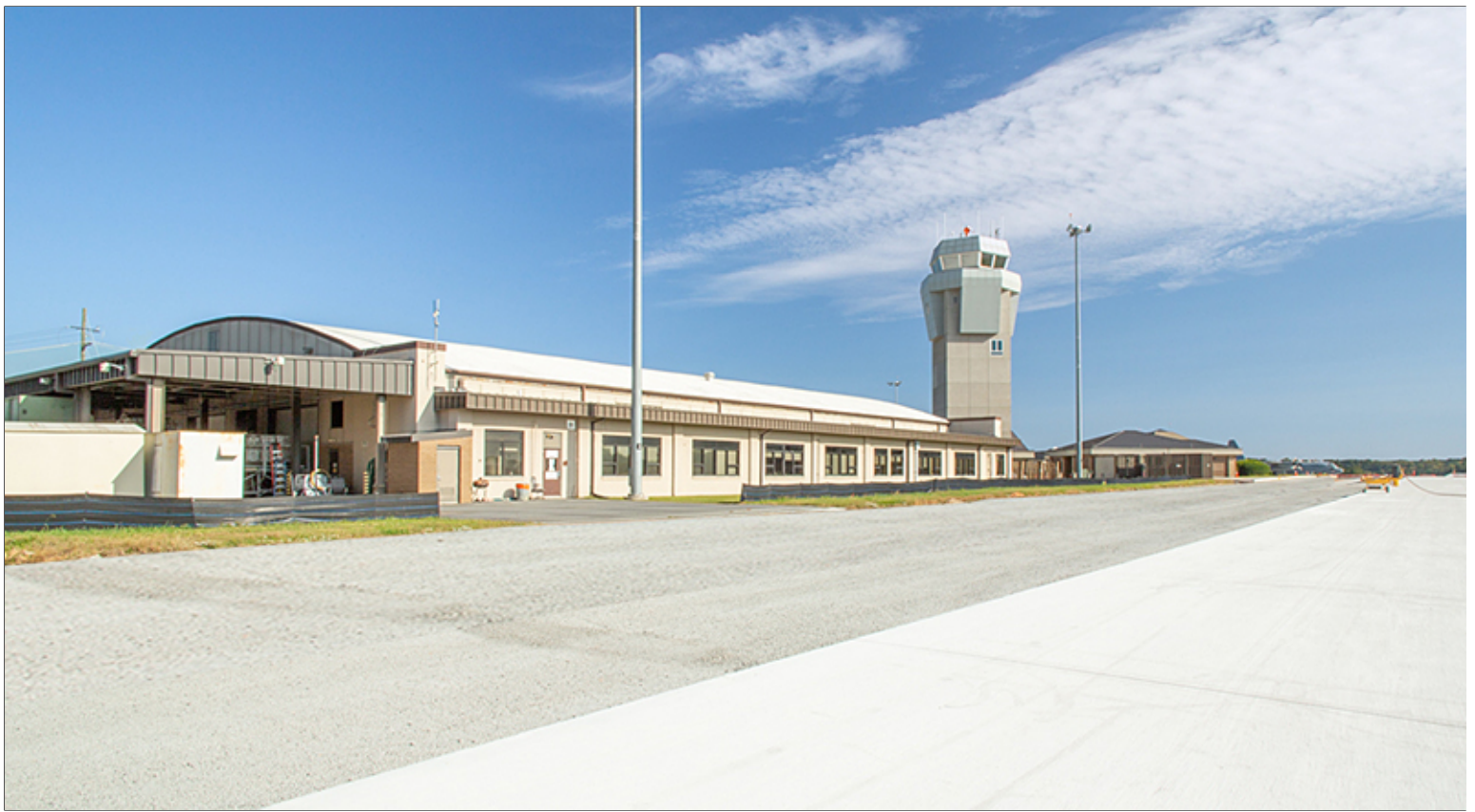
Architectural Features Typical of Group 3 in Foreground
