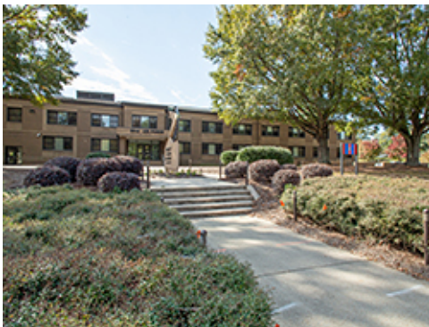
Site Stair at Group 1
