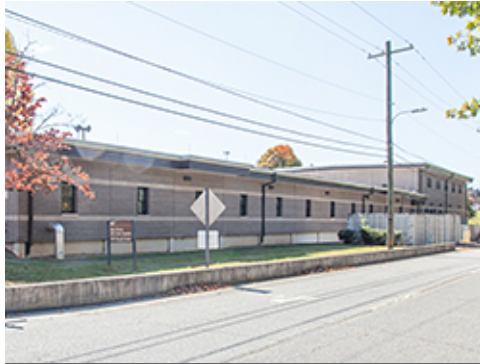
Overhead Service Lines
