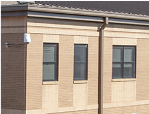
Brick Detailing at Windows
