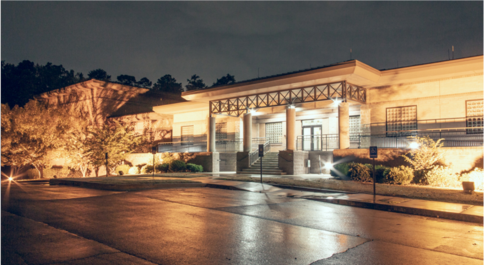
Coordinated Architectural Up-Lighting and Building Lighting at Group 1
