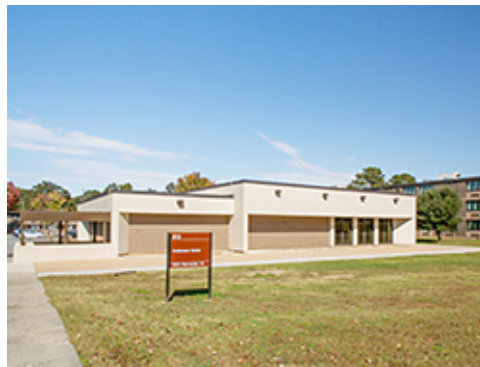
Administrative Group 2 Facility
