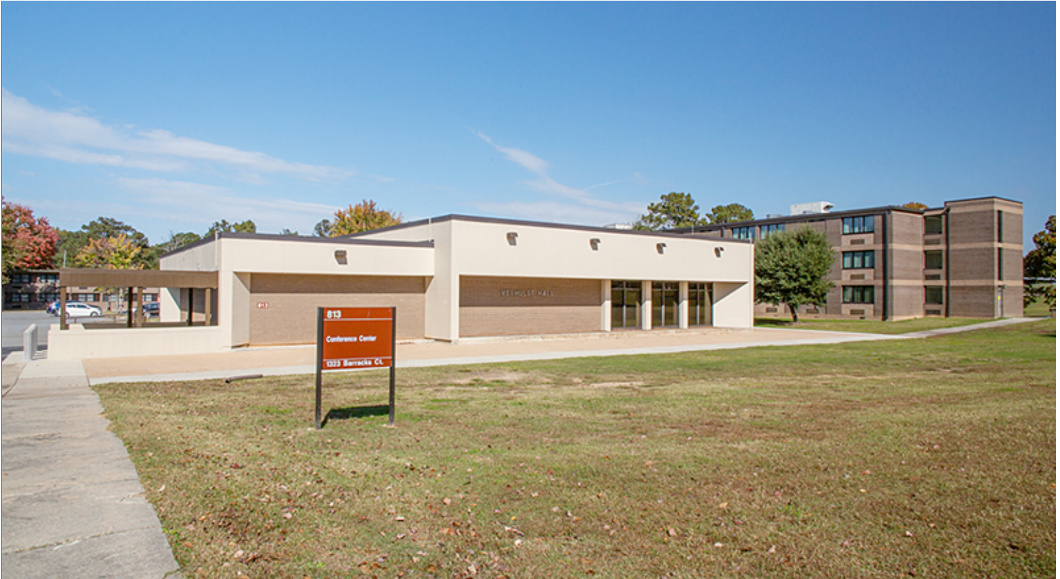
Coordinated Placement of Building Identification Sign
