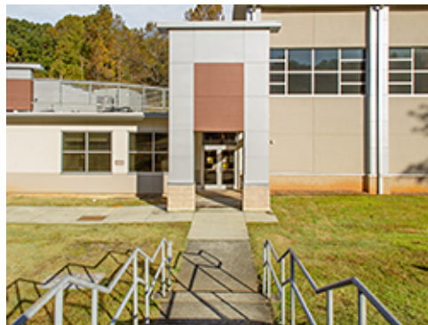
Group 2 Site Stair at Entrance
