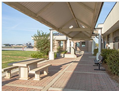
Red Pavers with Concrete Edging
