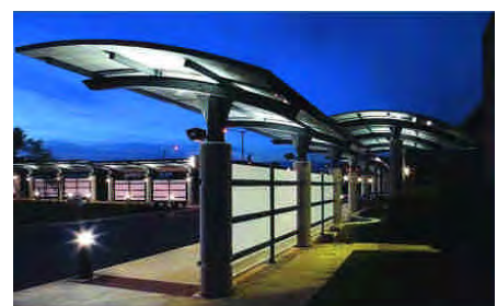
+ Sun shading (for the passenger terminal) should be compliant with building design
