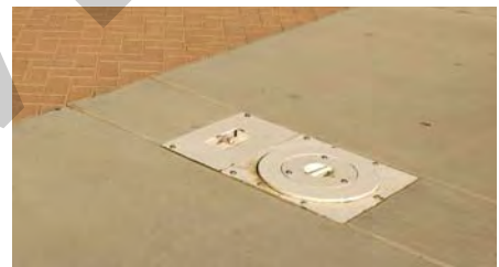
Recessed security bollard system
