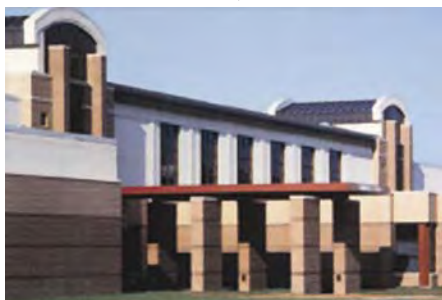
+ Unique roof line may be appropriate for this focus area.
