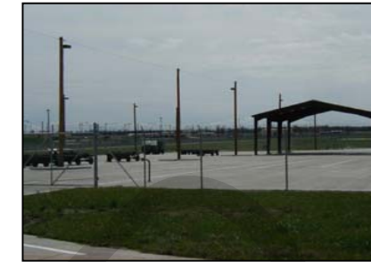
Lightning Protection System
