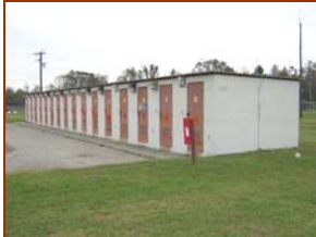
Figure 4.17 Segregated Magazine Storage - Langley AFB, VA
