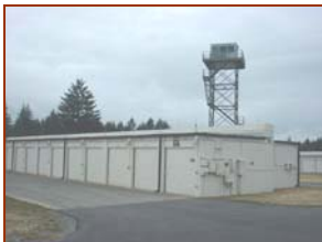
Figure 4.15 Multi-cubicle Magazine Storage - McChord AFB, WA
