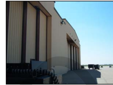
Wide Hangar Doors
