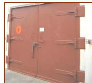
Figure 3.19 High Security Hasp on Storage Igloo - Luke AFB, AZ
