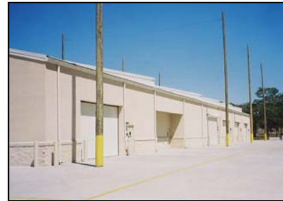
Drive-through Maintenance Bays
