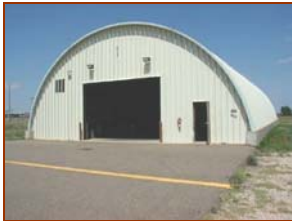
Figure 4.20 Above Ground Magazine Storage - Cannon AFB, NM
