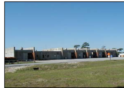
Exterior View of Surveillance and Inspection Shop
