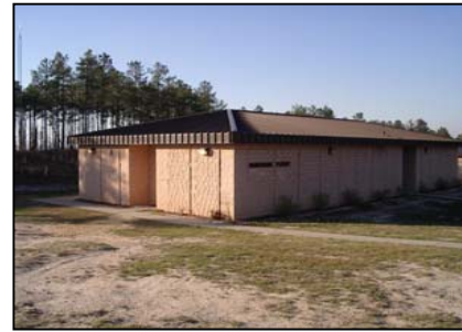
Munitions Administration Building
