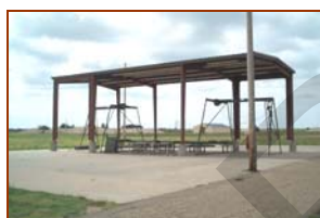
Figure 4.26 Ancillary Explosives Facility - MAC Pad - Cannon AFB, NM
