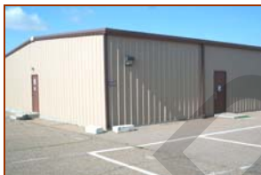
Figure 4.38 Munitions Administration Facility - Cannon AFB, NM
