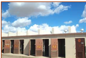
Figure 4.18 Segregated Magazine Storage - Luke AFB, AZ
