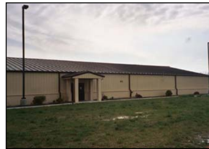
Munitions Administration Building
