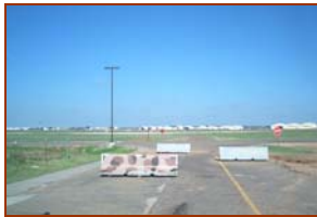
Figure 3.17 Security Barriers Protecting Entrance to Munitions Storage Area - Cannon AFB, NM
