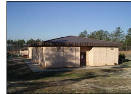
Block Construction with Metal Roof
