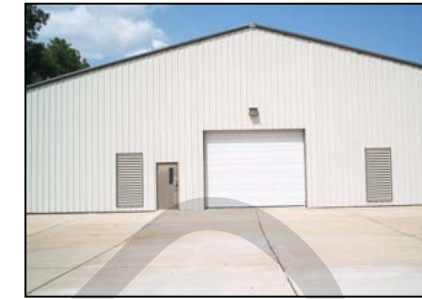
Surrounding Concrete Apron
