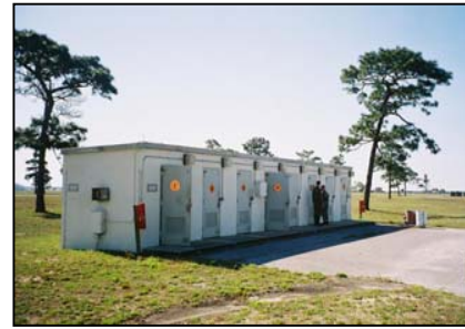
Segregated Storage Facility
