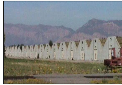
Segregated Bay Storage Area
