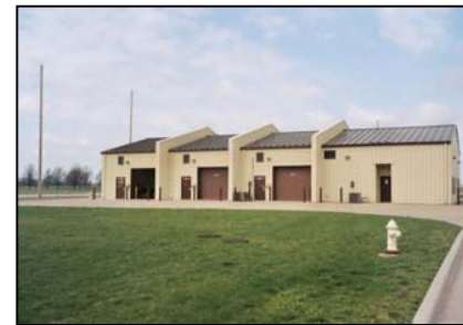
Wide Apron Provides Easy Access to Drive-thru Bays
