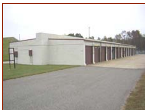
Figure 4.16 Multi-cubicle Magazine Storage - Langley AFB, VA
