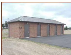
Figure 4.31 Munitions Holding Point - McChord AFB, WA
