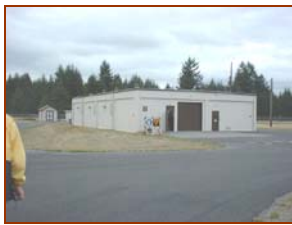
Figure 4.11 Surveillance and Inspection Shop - McChord AFB, WA
