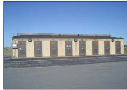
Segregated Storage Facility
