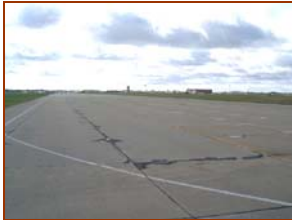
Figure 4.28 Dangerous Cargo Pad - McCord AFB, WA
