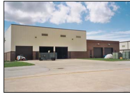
This Dual-use Facility Houses Load Crew Training (shown on left) with a Weapons Release Shop on the right
