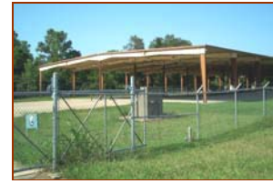
Figure 4.27 Ancillary Explosives Facility - Barksdale AFB, LA
