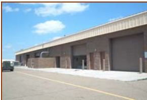
Figure 3.5 Exterior Elevations Employ Non-combustible Materials – Munitions Maintenance Facility – Cannon AFB, NM
