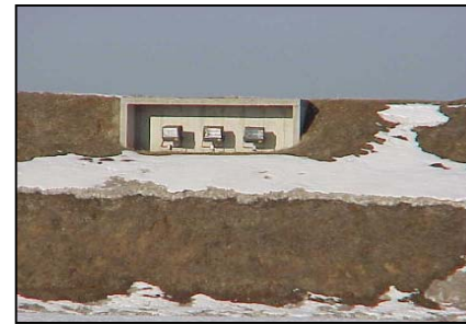
Revetment and Lighting
