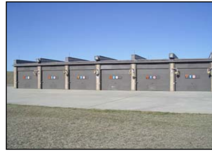
Multi-cubicle Magazine Storage Facility
