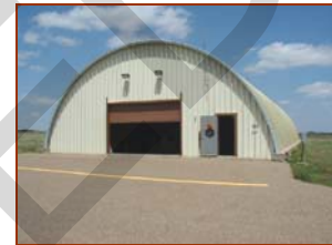
Figure 3.6 Steel-constructed K-span – Above Ground Magazine – Cannon AFB, NM
