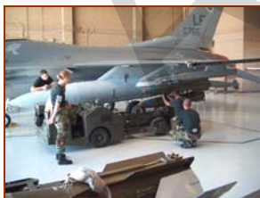
Figure 3.12 Chemical-resistant Urethane on a Concrete Floor – Munitions Loading Crew Training Facility - Luke AFB, AZ
