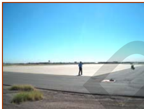
Figure 4.29 Dangerous Cargo Pad - Langley AFB, VA
