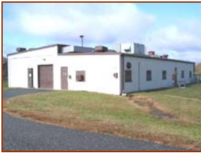
Figure 4.10 Surveillance and Inspection Shop - Langley AFB, VA
