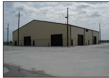
Drive-through Doors and Large Pad for Improved Access
