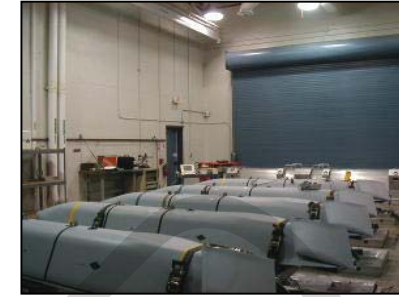
Large Maintenance Bay with Roll-up and Personnel Doors
