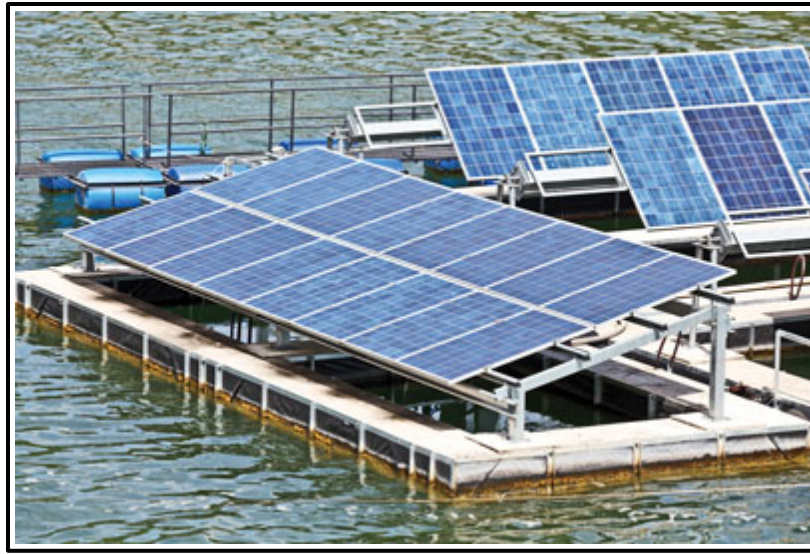
Figure 8. Floating PV system.
