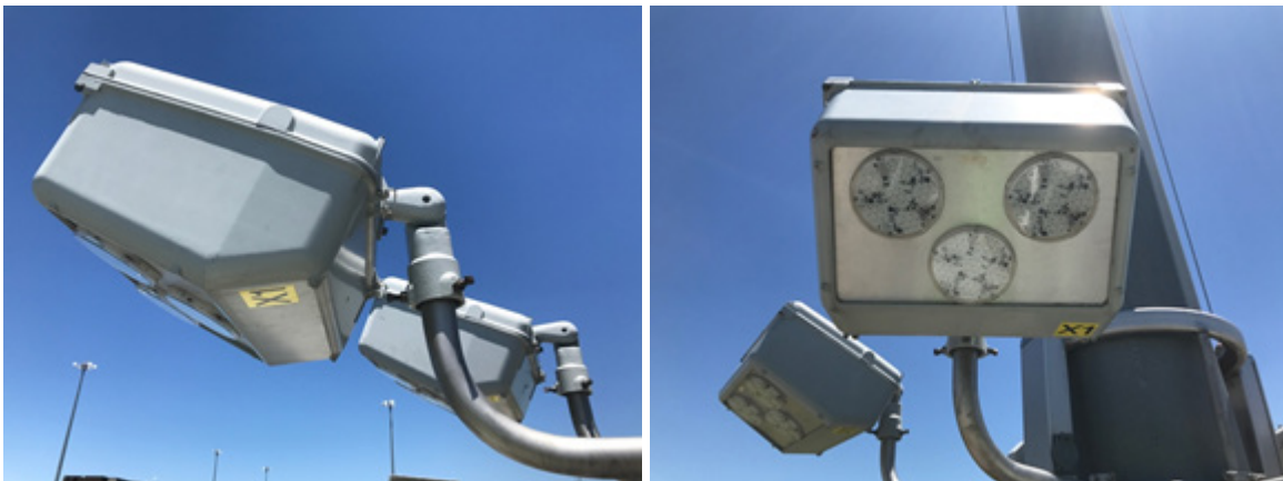
Figure 37. Locks No. 27 fixture retrofit.
