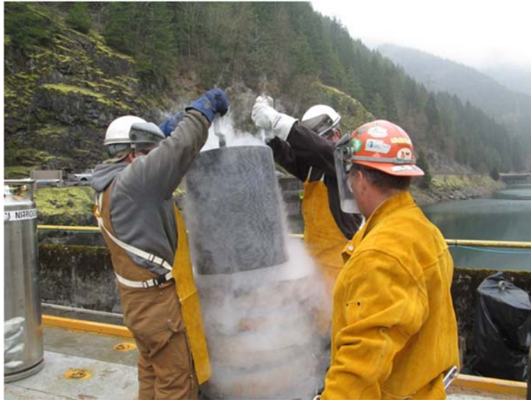
Figure 4. Spillway radial gate trunnion bushing - freezing in liquid nitrogen (USACE).
