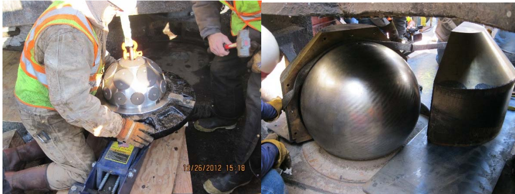
Figure 8. Lock 6 and LPV 144 pintle installation.
