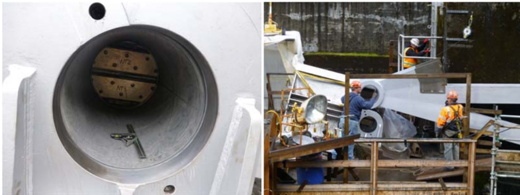
Figure 3. Textile reinforced polymer self-lubricated materials for radial gate trunnion bushing (USACE).
