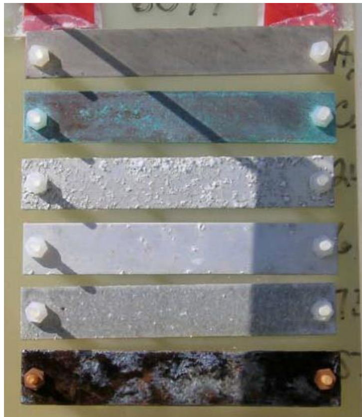
From A Decade of Corrosion Monitoring Report
