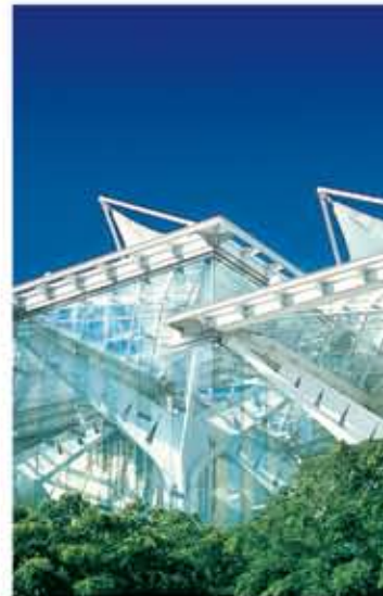
The Hawaii Convention Center, Architect: Wimberly Allison Tong & Goo. Design and Planning: LMN Architects. Features the largest suspended glass wall in the U.S. fabricated by Oldcastle Glass ® in Stackwall. ™
