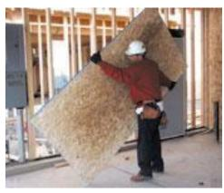
Wall C with Fire Rated Plywood is sometimes preferred over Expanded Metal for enhanced walls to mitigate against surreptitious entry.
