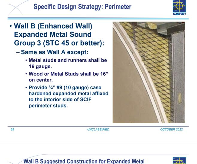
Only for sound attenuation of wall: Don't Forget Ceiling and Floors
