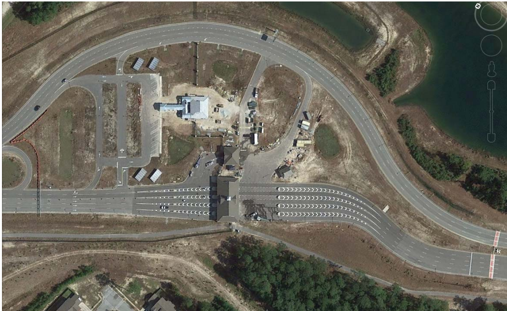
USMCB CAMP LEJEUNE- WILSON BLVD GATE
