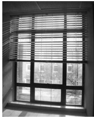
FIGURE 4 Used in conjunction with glazing film, blast blinds retain historic windows while providing improved thermal efficiency and blast protection. Supporting cables are anchored at the top and bottom of the window frame, so blinds can be opened and closed, not raised or lowered. (GSA)
