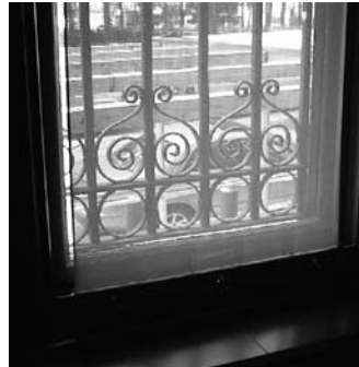
FIGURE 5 Blast shade detail showing fabric anchored to the window frame to contain glass fragments and sash units. Shades can be designed to conform to the contours of arched windows and other unusual openings. (GSA)
