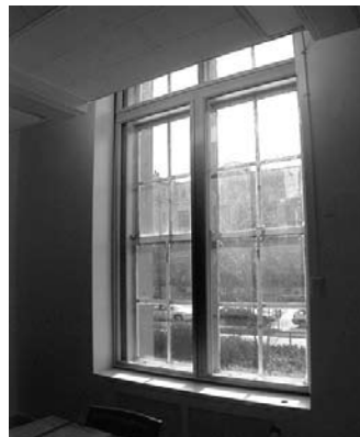
FIGURE 6 Interior views of blast-resistant storm windows. They are designed to contain flying debris, preserve the historic character of building exteriors and interiors, admit daylight, offer energy savings and, with operable product options, allow fresh air inside the building. (Oldcastle-Aral, Inc.)
