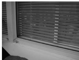
FIGURE 7 Detail views of demountable blast-resistant, thermal storm windows with built-in blinds to control daylight. (Chad Randal, National Park Service)
