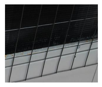
Coated HVAC fins have been proven to extend the life of a system.
