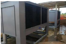
A newly acquired HVAC system with coated fins is placed within protective wall to extend the life of the system (Guam).
