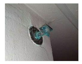
Corrosion related to health and safety is more likely to elevate corrective actions. Pictured is a highly corroded sprinkler head.
