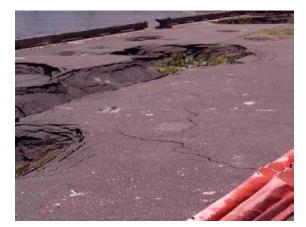
Wharf deterioration (nonmission-essential) is allowed to continue because of a lack of funds.
