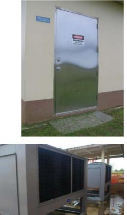
An example of a corrosionresistant stainless steel door in a high ESI zone (Guam).
