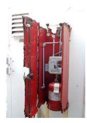
This corroded fire extinguishing system could be elevated as a safety priority. On the topic of competition for corrosion-related resources, the field representatives provided the following input:
