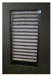
Local standards in Guam call for sealing intake of chiller rooms to mitigate corrosion.
