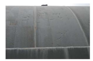
Pitting corrosion on a fuel tank, Guam.
