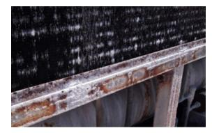
Uncoated fins on this HVAC system are less than 2 years old.
