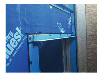
**Fig. E.3** View of air and weather barrier integrated into rough opening to receive replacement window
