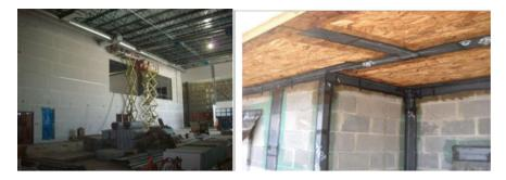
**Fig. 9.9** Gypsum air barrier partition wall used to compartmentalize an interior space: Left, see rear wall; Right, CMU and OSB sheathing is used as an air barrier assembly. (Photo courtesy of Nicholas Alexander, USACE)
