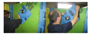
e. Step 5: When the area has been covered with the self-adhered membrane and rolled with a membrane roller, the installer can then apply a bead of sealant over all non-factory areas that have been cut or where there are any chances of air or water infiltration into the assembly. The sealant then needs to troweled to a smooth finish.
