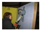
b. Step 2: Apply manufacture's approved primer/adhesive to the wall in the approved method and allow to flash off or cure according to the climactic conditions for that day. These primers are required on all substrates that are going to have a sheet rubberized asphalt membrane installed. If a butyl membrane is being installed, primers are not required in some cases.
