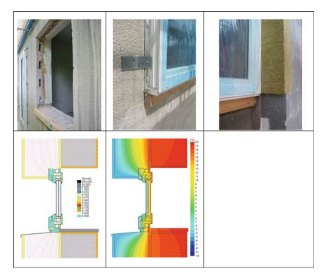
Fig. E.10 Example of old window replacement: (a) old Window opening with masonry rabbets removed. (b) The addition of a horizontal wooden support facilitates fixture of windows; it is installed and leveled in advance and bears the window's weight. The window is then fixed with stainless steel angle brackets. (c) Top and lateral parts of the window frame are covered with the exterior wall insulation as far as possible. (d) Schematic of window installation. (e) Thermal image of window performance
