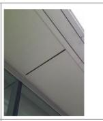
Seal all joints in this soffit using a Dymonic® color-matched product. Need outside quotes for this type of work
