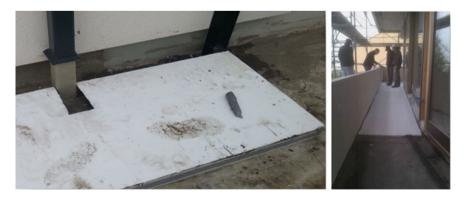
Fig. C.19 Loose lay, adhesive, or mechanical fix to terrace or balcony. Increase R-value without increasing thickness above safety height for fall/water ingress. System is compatible with traditional membrane and ballast systems
