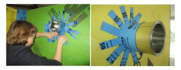
d. Step 4: Install a sheet of self-adhering membrane over the previously installed fanned out membrane. This can be done using two overlapping pieces or one continuous piece over the detailed area.
