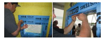
k. Step 11: These installed pieces should now be rolled with a membrane roller to properly adhere them to the substrate.
