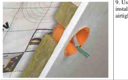
9. Use the space from the inside for electronic installation without damaging vapor retarder/ airtightness
