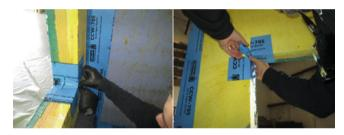
h. Step 8: Next, install a strip of membrane across the sill of the rough opening that extends past the jams by approximately 4 ½ in. if you are using 9-in.-wide transition membrane. Then cut the membrane at each corner of the rough opening and fold the membrane onto the sill.
