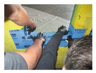
i. Step 9: Install strips of transition membrane on each of the jams, starting at the top of the sill. Cut horizontally across the membrane from the edge of the rough opening and fold into the rough opening.
