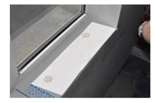
Fig. C.15 Mechanical fixing (Polymer) of IWI thermal bridging assembly at window reveal (Aerogel Blanket, Vapor Barrier + MGO board)
