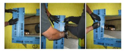
j. Step 10: Now install a piece of transition membrane across the head of the window. Then cut vertically to the inner edge of the rough opening and fold the membrane up into the underside of the head area of the rough opening.
