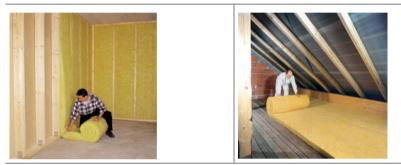
Batts and rolls are available in widths suited to standard spacing of wall studs, attic trusses or rafters, and floor joists. Note the batt insulation in between the roof rafters.
