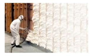
foam insulation as a vapor barrier, so installation might require an additional vapor retarder.
