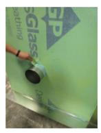
c. Step 3: Sealing round penetrations by cutting self-adhered membrane to fan out around the penetration.
