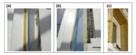
Fig. E.13 Window/wall gap is sealed using mesh glued to the window frame from the outside using adhesive connector (c, d, e). Plaster is laid over the mesh and then painted over
