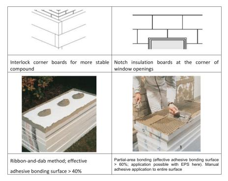
Fig. C.1 Examples of insulation installation using adhesives
