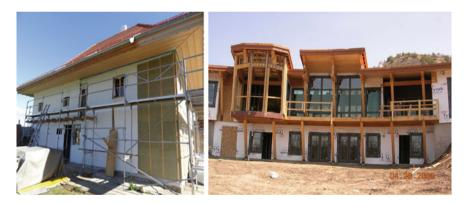
Fig. C.16 Mechanically fixed to battens in strip or blanket format to increase R-value and reduce repeat thermal bridging through studs
