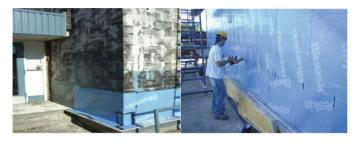
Fluid-applied air barrier installed over an existing exterior wall area and insulated with medium-density closed-cell spray polyurethane foam.
