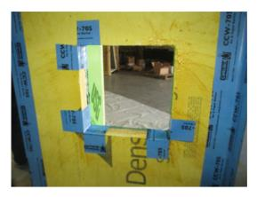
g. Step 7: Then install a bow tie-shaped piece of membrane into each corner of the rough opening. This piece is installed to prevent water or air from entering into the assembly at the small hole that remains in each of the corners of the rough openings.
