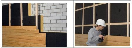
Ventilated façade with wooden supporting structure and wooden cladding profiles
