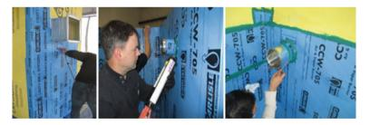
f. Step 6: Detailing around windows and doors. Prime all surfaces as previously mentioned. Then install a piece of membrane into each corner of the rough opening with one half of the membrane folded onto the wall area as shown.
