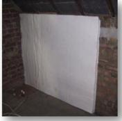
Fig. C.17 Mechanical and adhesive fix to internal wall. Finish with wet plaster/lime or rigid facing board according to customer needs. Perform robust risk assessment to determine hygro-thermal impacts of IWI upgrade
