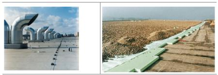
Flat roof with insulation layer (XPS) on top of waterproofing (Umkehrdach)
