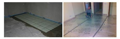
Fig. C.20 Loose lay or panel application, suitable for domestic loadings. Address heat loss through concrete slab without requiring door/threshold adjustments
