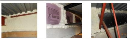
After. Typical soffit: usually can be blocked vertically from interior of building and sealed when access is not possible for sealing joints from exterior
